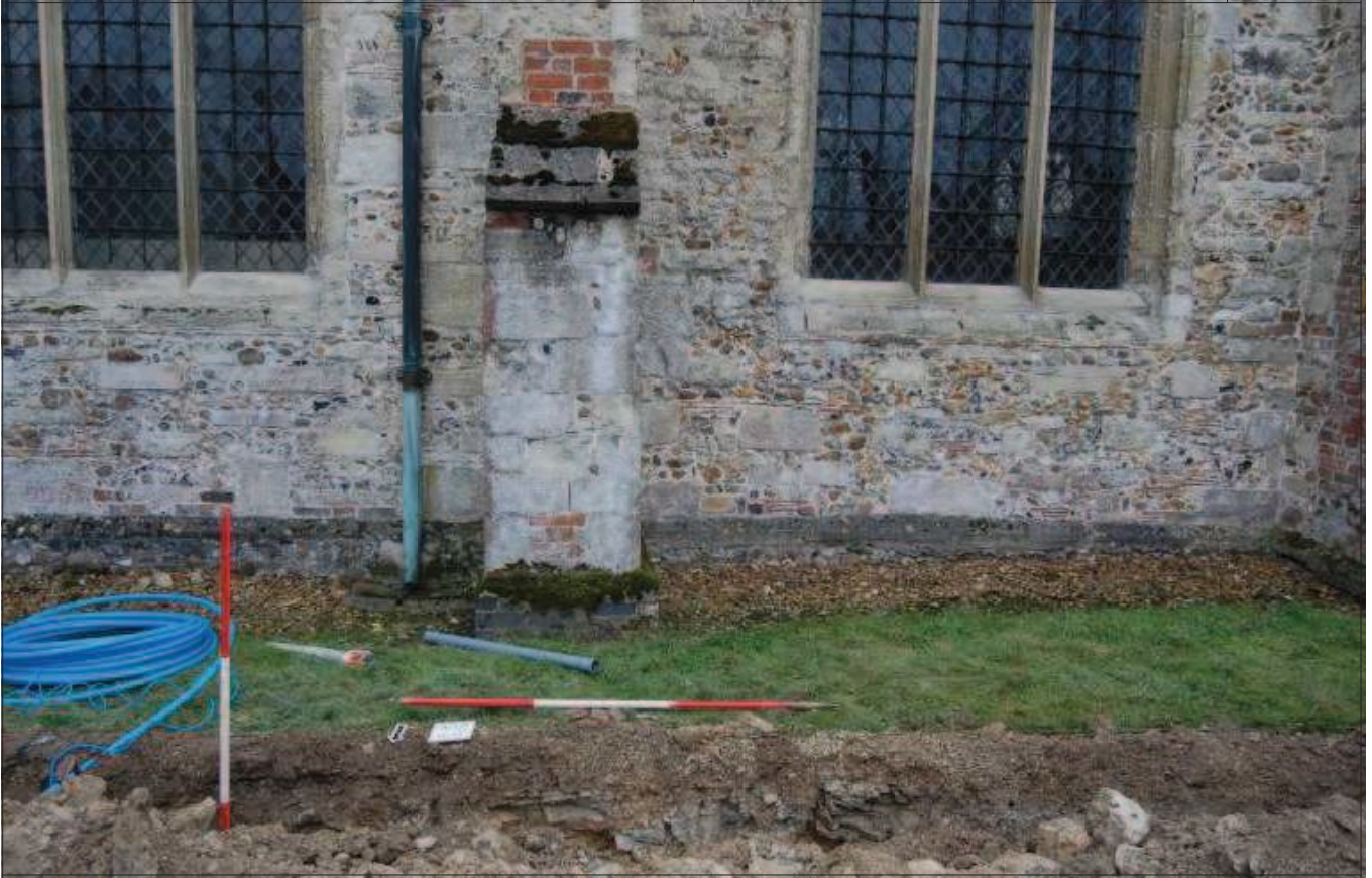
Plate 3: Stone foundation [01] in context looking south
