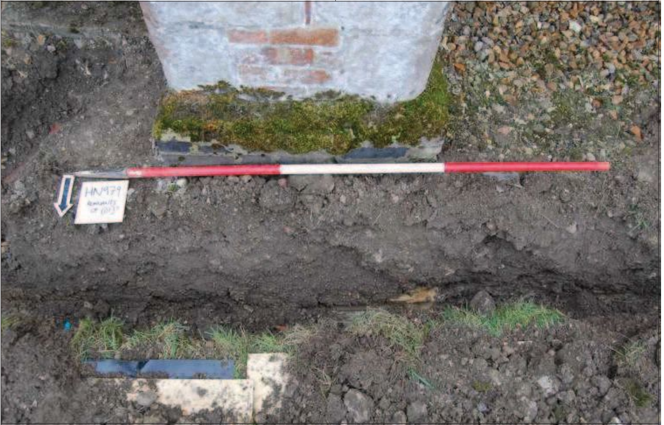
Plate 5: Re-excavated drain trench on line of foundation [01] looking south
