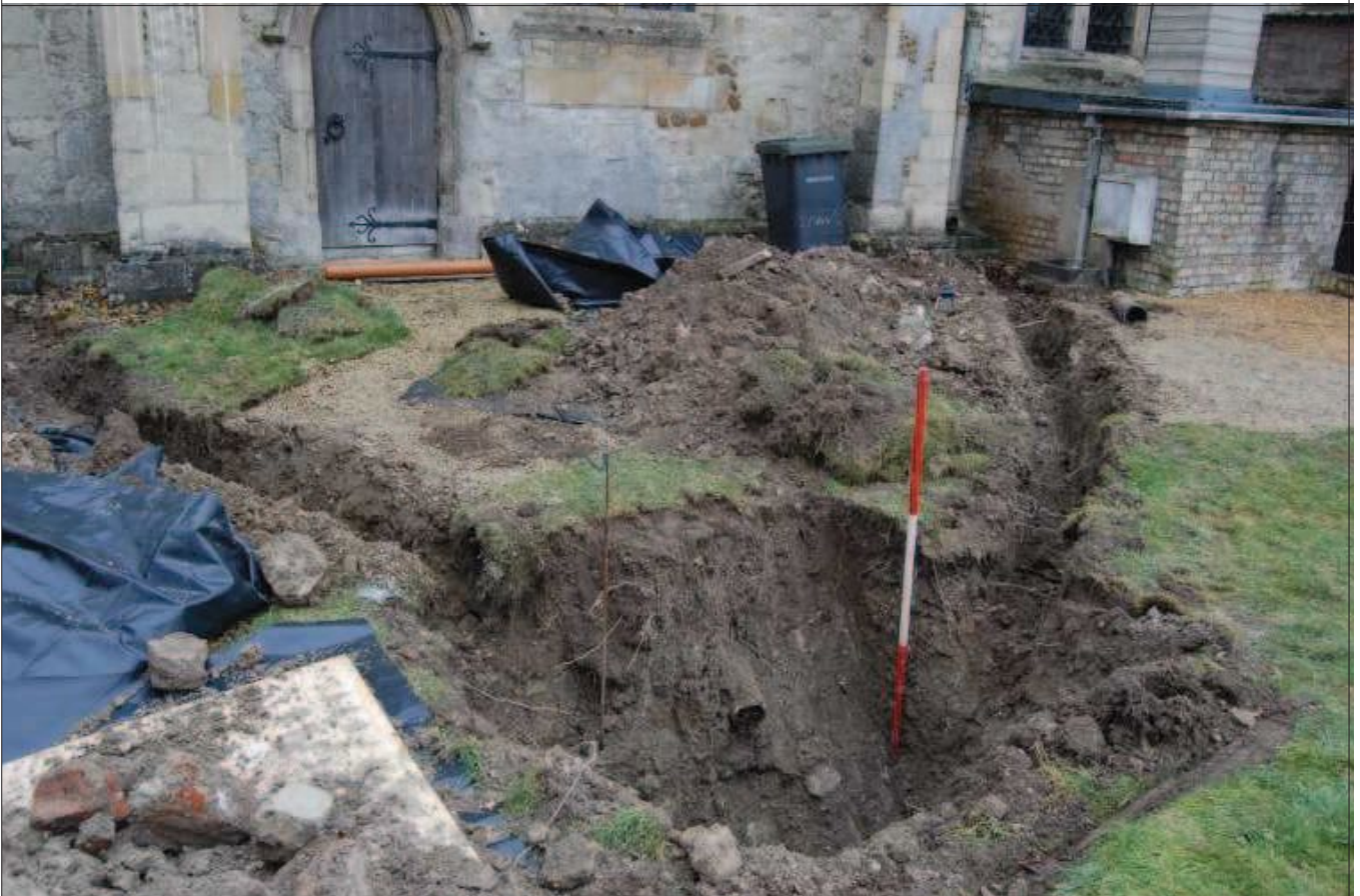
Plate 6: Soakaway 1 looking SW
