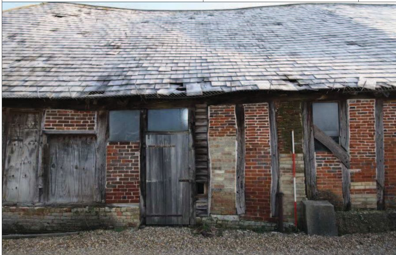
Plate 5: Detail shot of Bays 3 - 4 west exterior elevation
