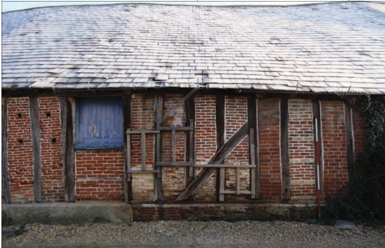
Plate 7: Detail shot, Bays 6 - 7, west elevation
