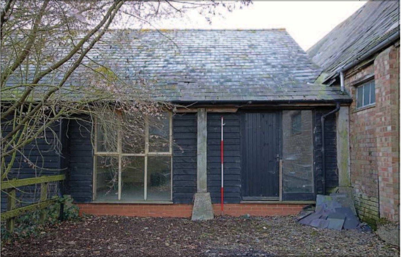
Plate 15: East barn, north elevation, looking S
