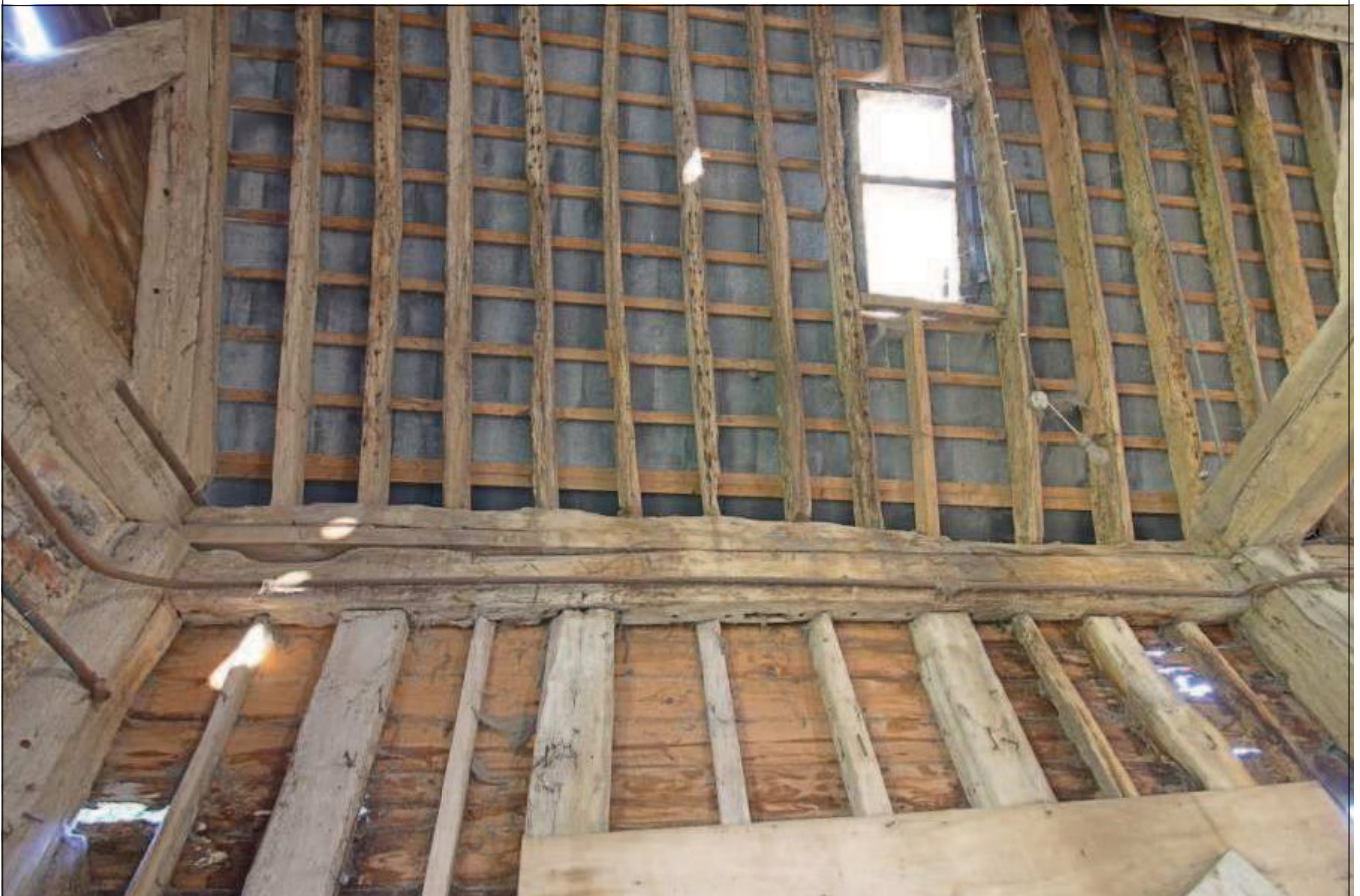
Plate 24: Bay 1, east elevation, underside of wall plate showing dowel holes
