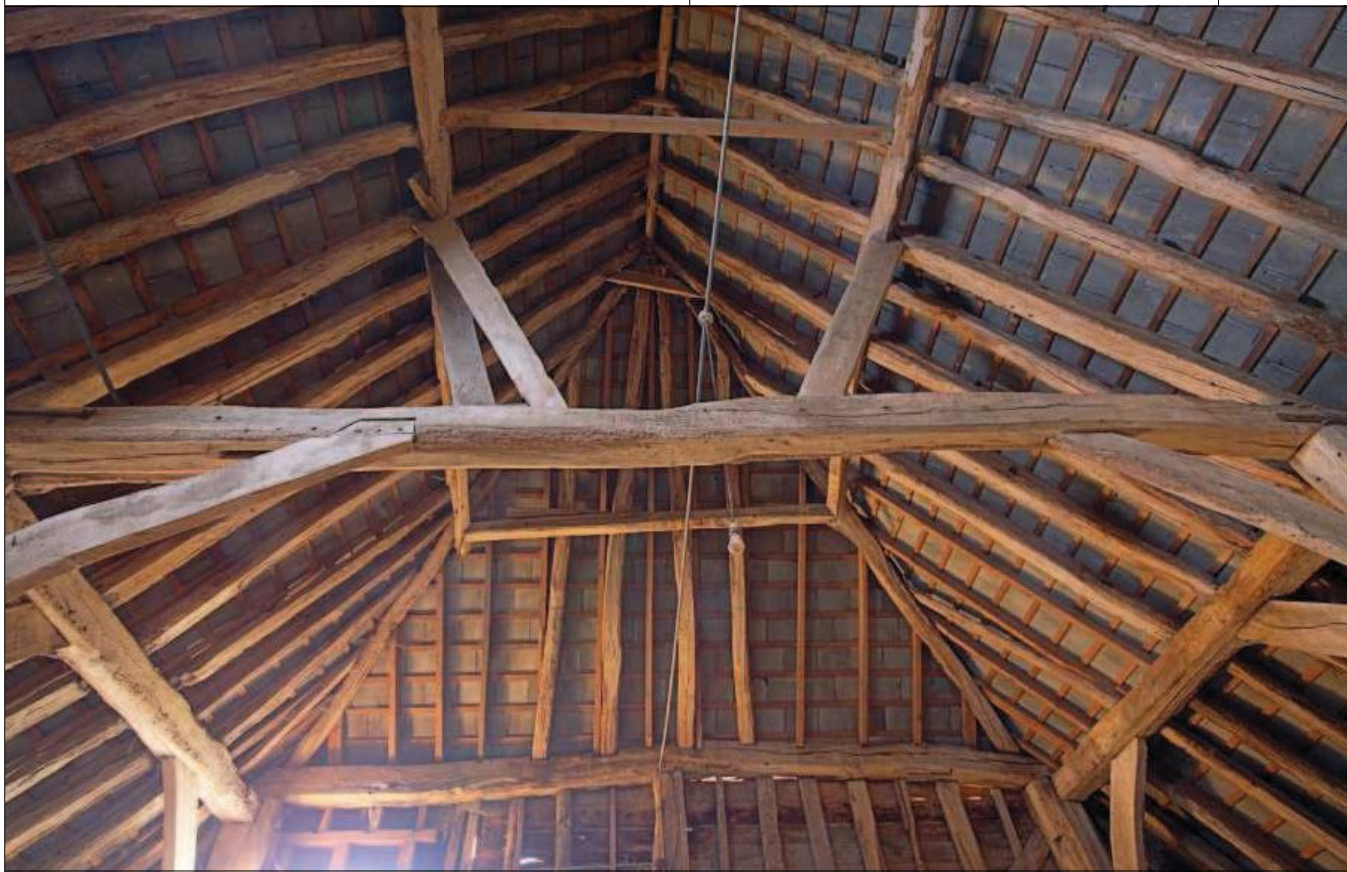
Plate 21: Hipped roof space above south gable
