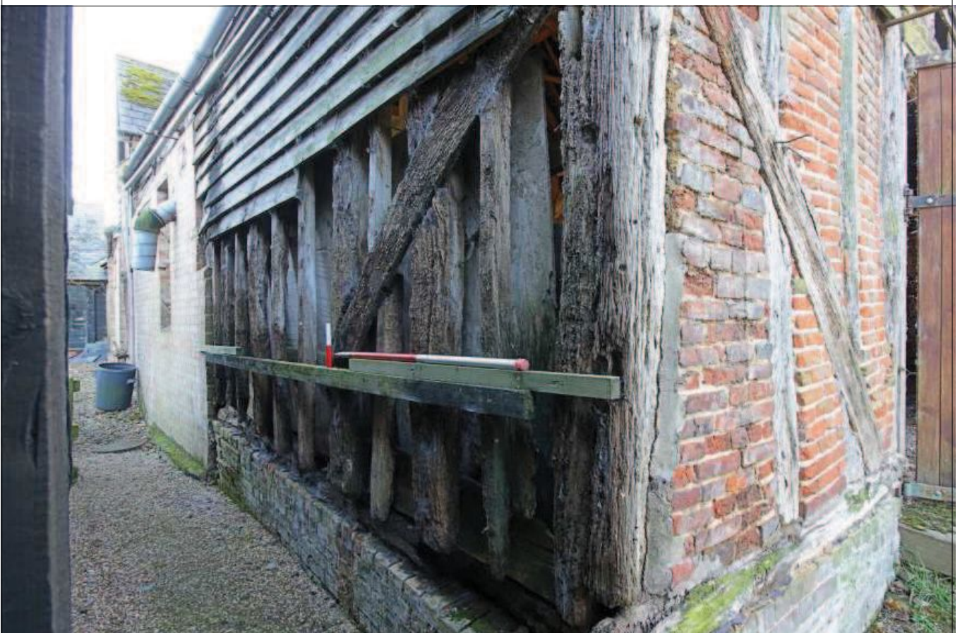
Plate 12: East exterior elevation, Bay 1, looking SSW
