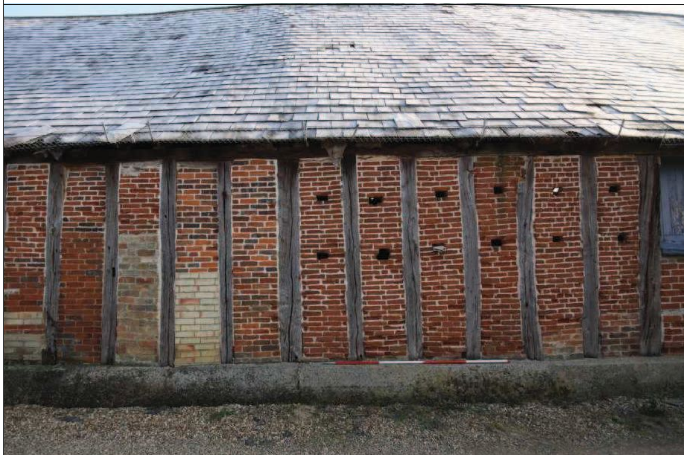
Plate 6: Detail shot of Bays 4-5, west elevation
