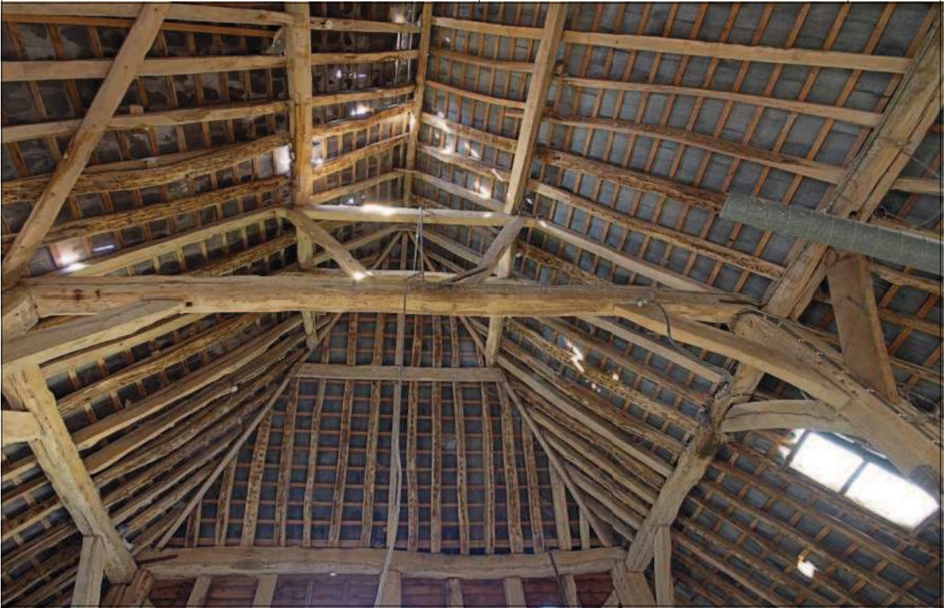
Plate 19: Hipped roof space above north gable
