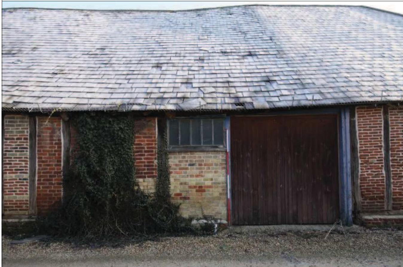
Plate 8: Detail shot, Bays 7 - 8, west elevation
