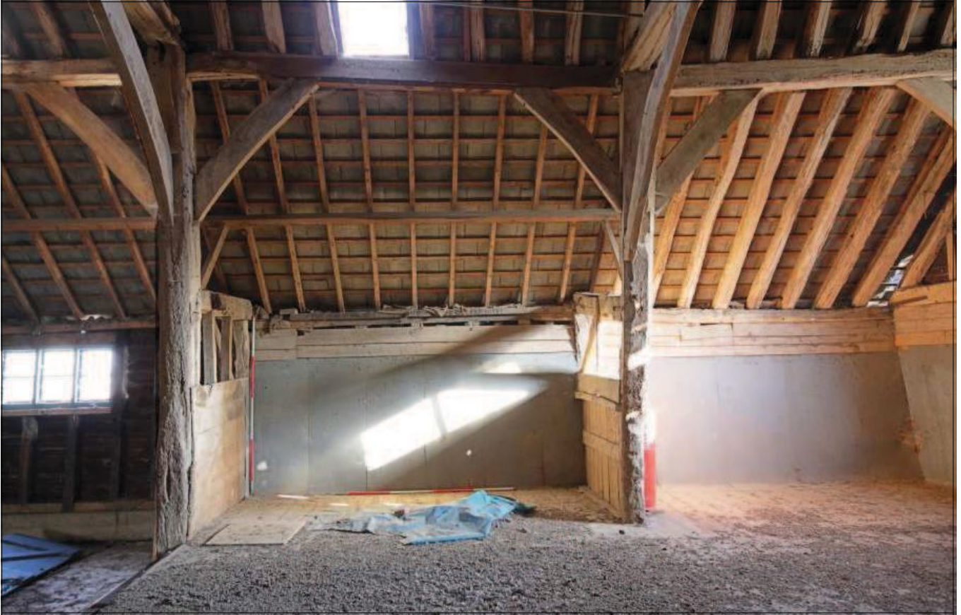
Plate 23: Wooden threshing floor, Bays 9 - 10, looking E
