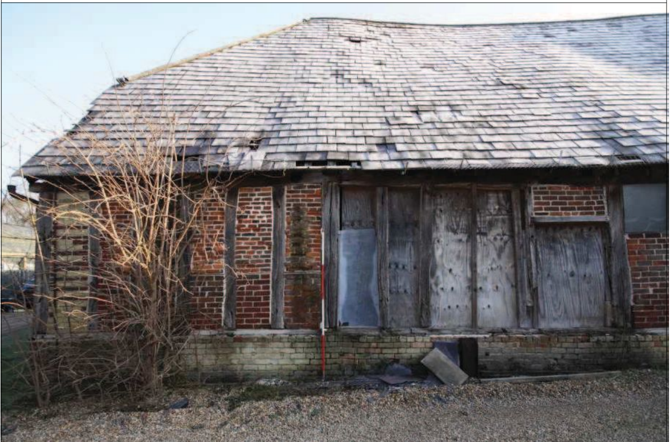
Plate 4: Detail shot - Bays 1 - 2, west exterior elevation
