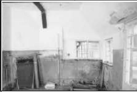
248/20-21: Annexe, main room, W end W interior elevation
