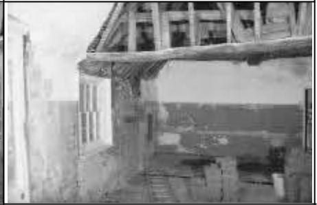
248/28-29: Annexe, main room, E end looking NE
