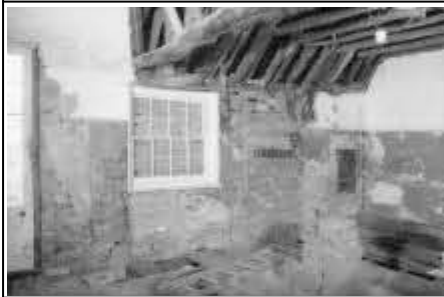
248/30-31: Annexe, main room, E end looking NE
