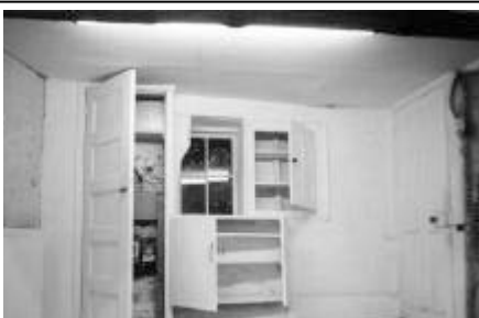
CP8: Annexe, former kitchen, S interior elevation
