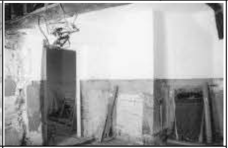
248/22-23: Annexe, main room, W end SW corner
