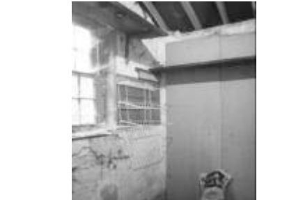
CP5: Lean-to, interior from SE
