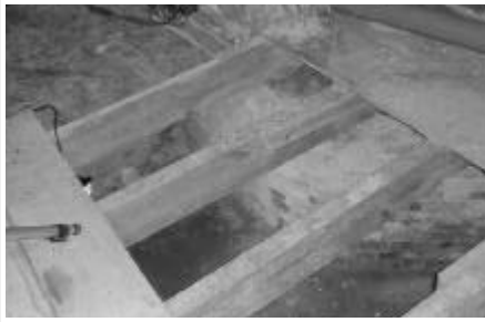
DP1: Annexe, chimney base looking SW
