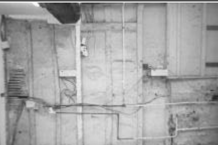
CP7: Annexe, former kitchen, W interior elevation
