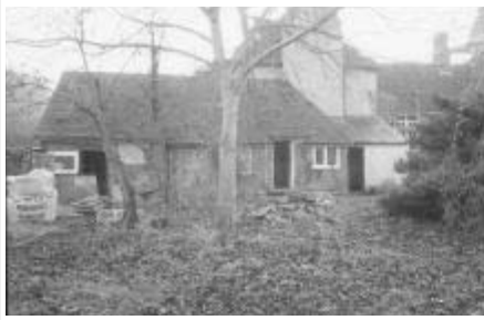
MF4: Annexe and lean-to from N
