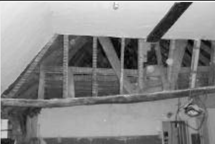
DP4: Annexe, main room tie-beam looking E
