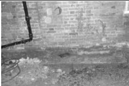
DP11: Annexe, former chimney base against N elevation from N
