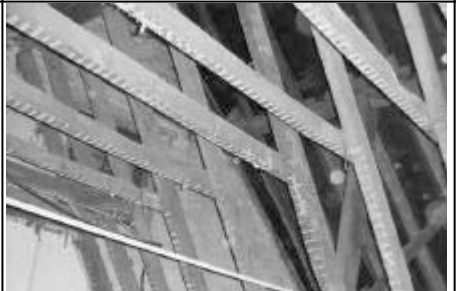
DP9: Annexe, former kitchen ceiling structure looking SE
