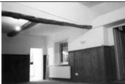
CP11: Annexe, main room looking SE
