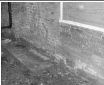
DP10: Annexe, former chimney base against N elevation from NW
