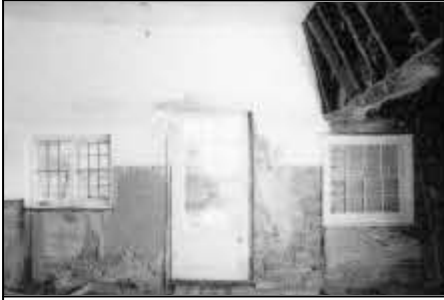
248/18-19: Annexe, main room, W end N interior elevation
