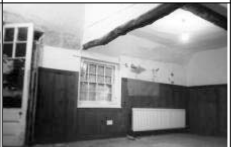
CP12: Annexe, main room looking NE
