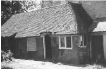
CP1: Annexe, N & W elevations from NW
