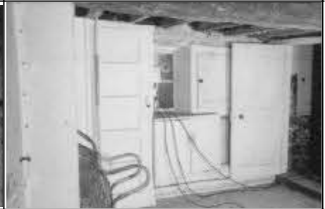
248/34-35: Annexe, former kitchen, S interior elevation
