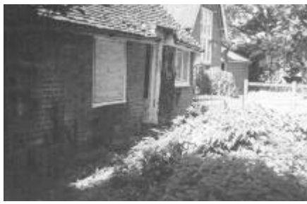
CP2: Annexe, N elevation from NE
