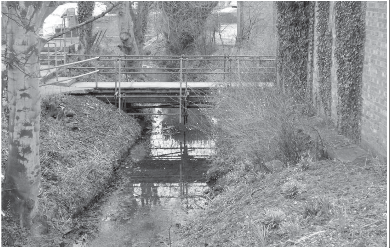
Plate 4: Footbridge over the River Bulbourne looking E
