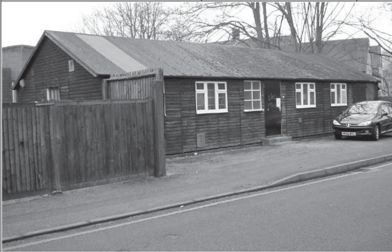
Plate 6: Building 3 looking S
