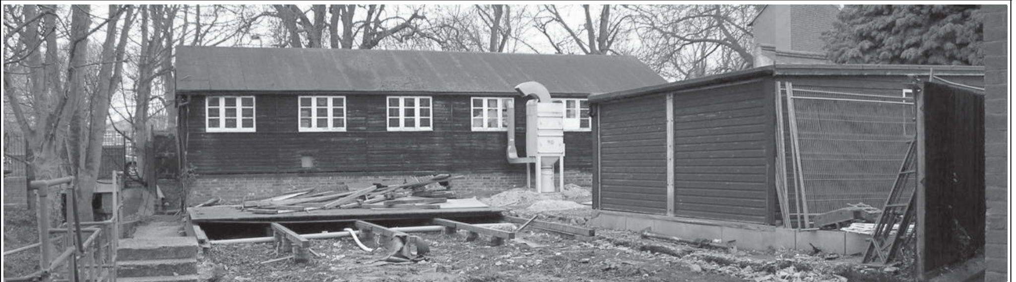
Plate 11: Area to N of River Bulbourne looking NW
