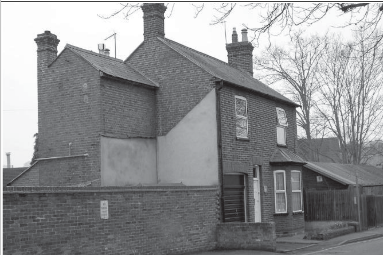
Plate 7: Building 4 (Caretaker's House) looking S
