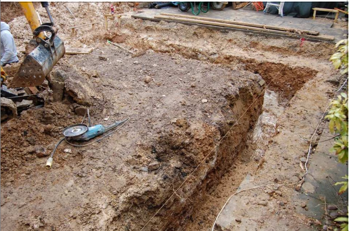
Plate 2: Geological deposits revealed in footing trench, looking northwest.
