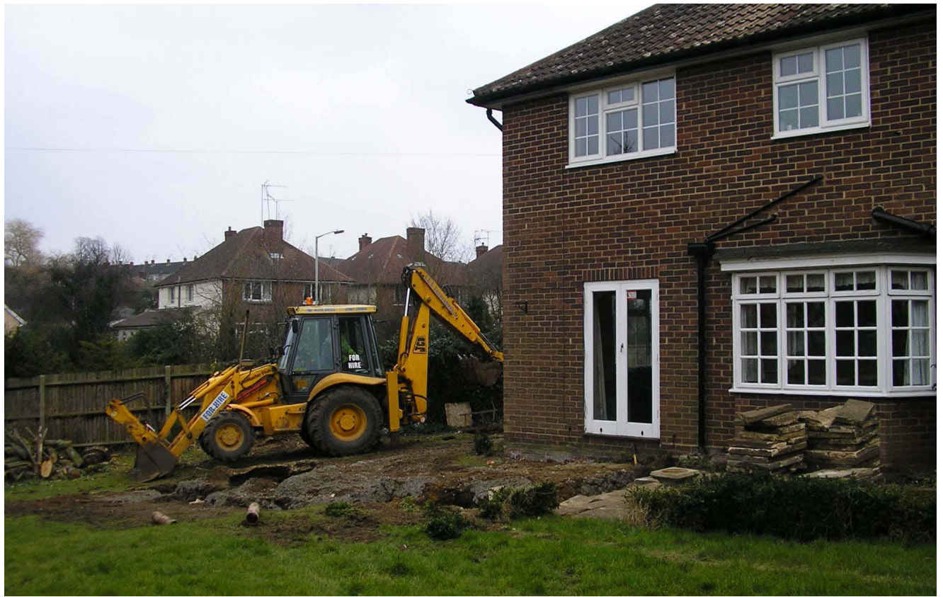
Plate 1a: Excavating footings trenches
