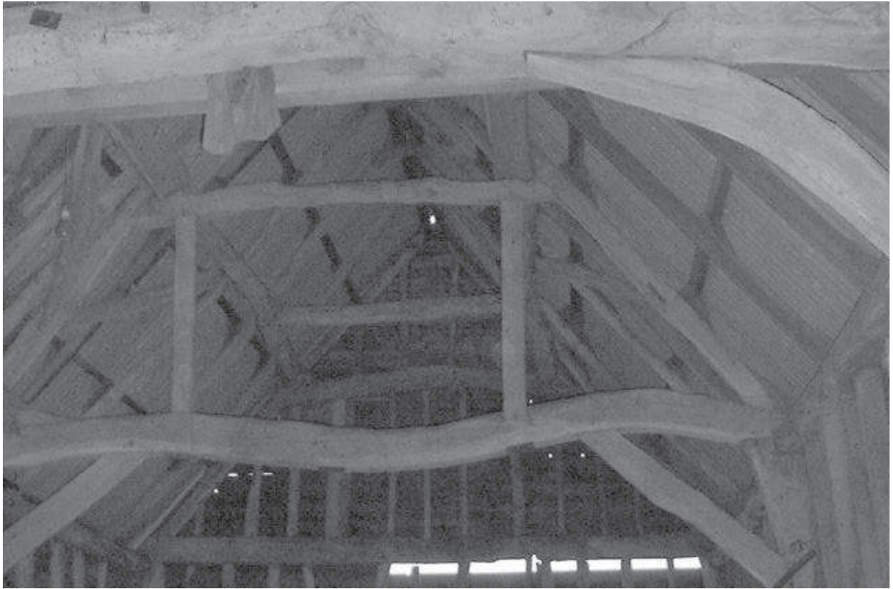
Building 1: queen post roof, looking east
