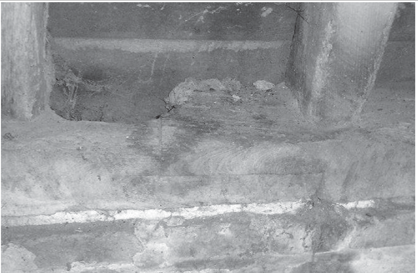
Building 1: edge-halved scarf joint with square abutments
