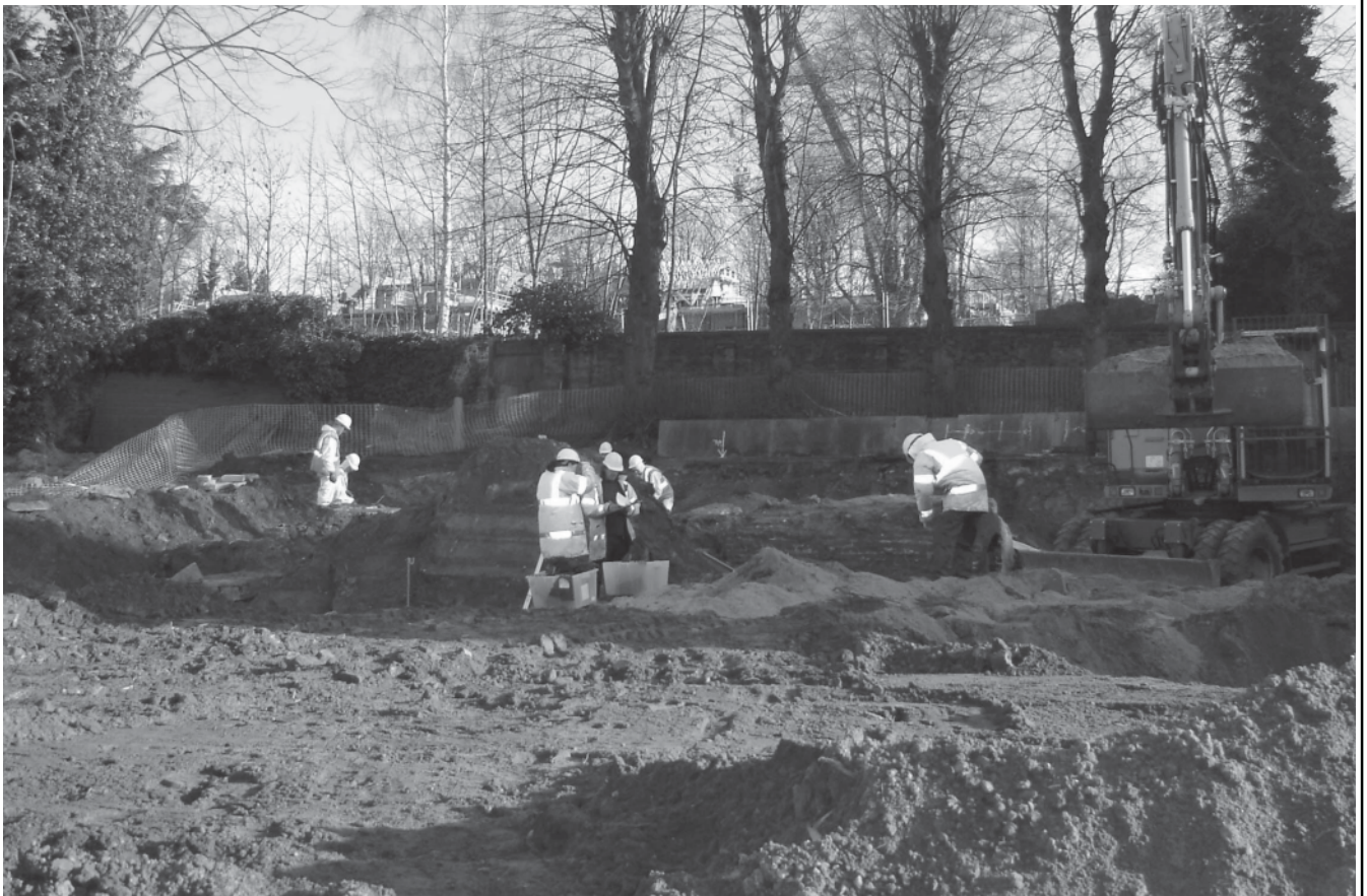
Plate 4: General view of site, looking E
