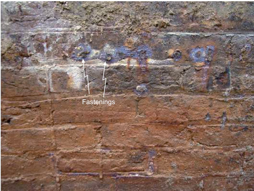
Plate 2b: Close up of fastenings for collar
