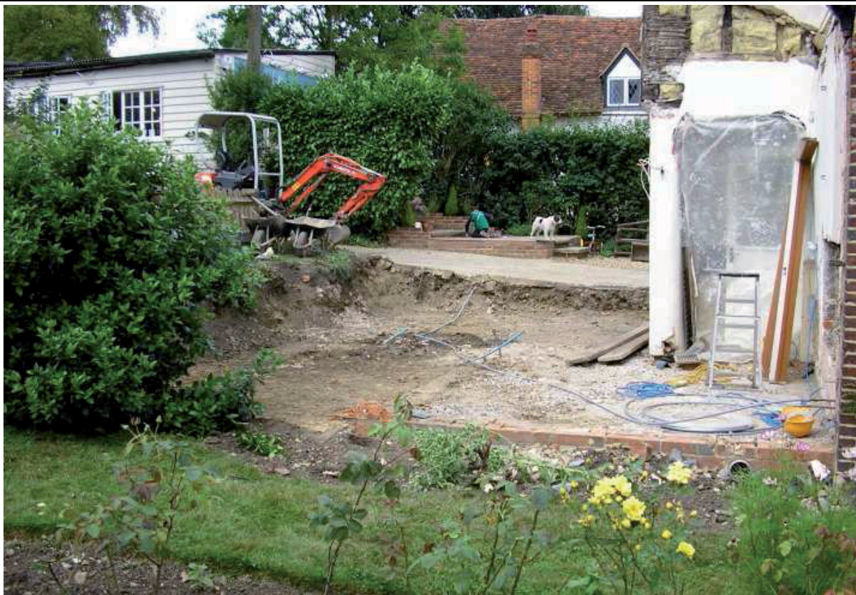
Plate 1: Ground reduction - building footprint, looking north east
