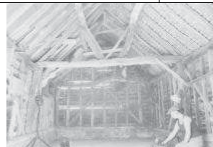
Frame 3: Barn, roof truss and N internal elevation
