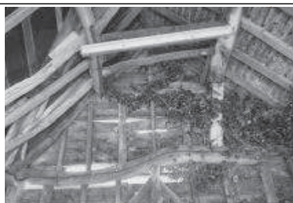
Frame 7: Barn, N roof truss
