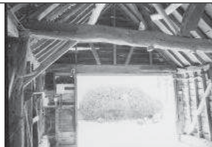
Frame 10: Barn, S internal elevation
