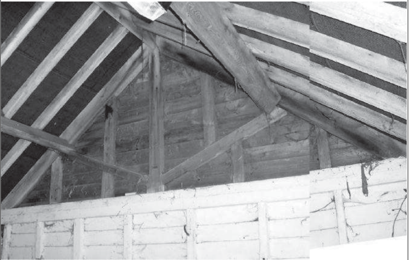
Plate 9: Stables: roof truss
