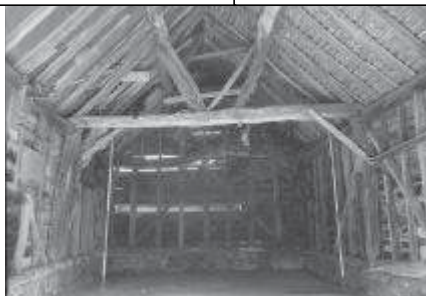
Frame 2: Barn, roof truss and N internal elevation
