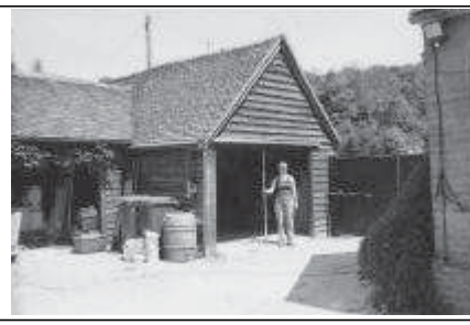
Frame 15: Barn, S & E elevations
