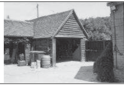
Frame 14: Barn, S & E elevations
