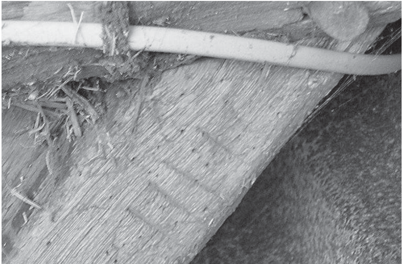
Plate 5: Carpenter's mark on western middle principal rafter
