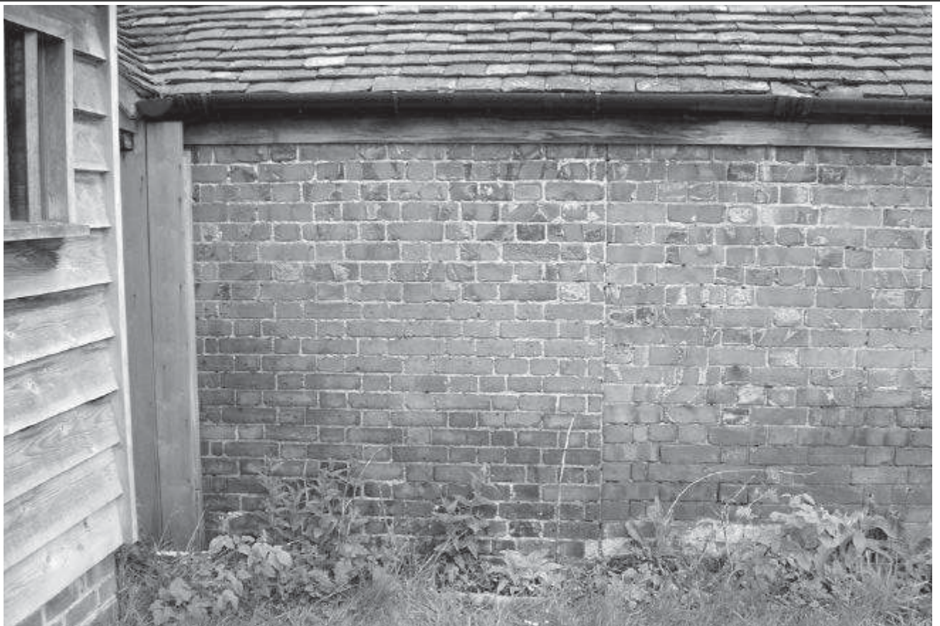
Plate 8: Stables, blocked through way
