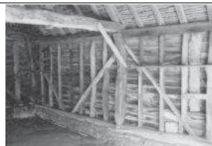
Frame 12: Barn, E internal elevation
