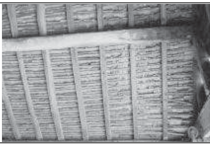
Frame 13: Roof, showing torching
