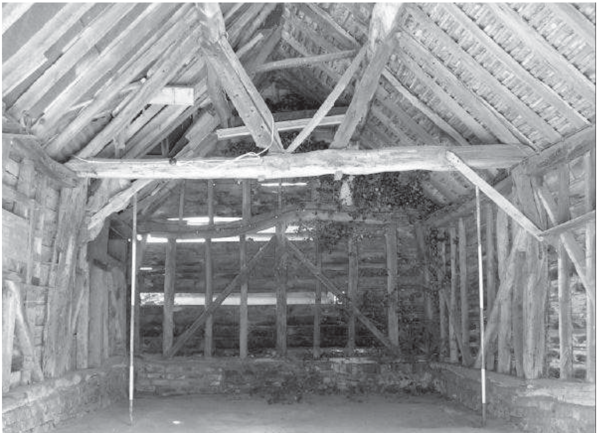
Plate 4: Barn, interior looking N
