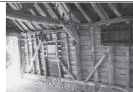
Frame 9: Barn, E internal elevation
