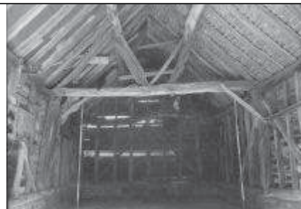
Frame 1: Barn, roof truss and N internal elevation
