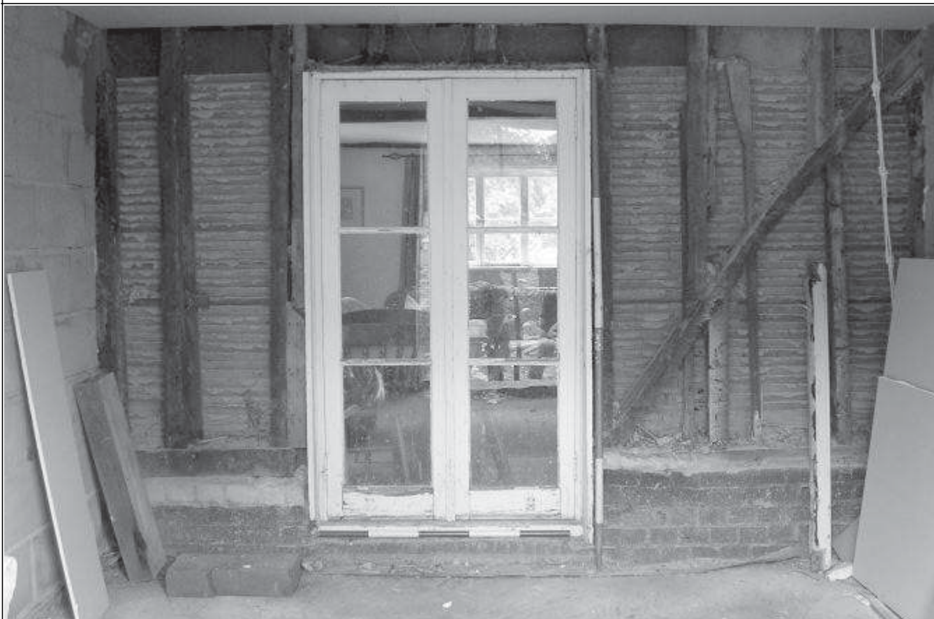
Plate 2: External southern elevation after removal of render
