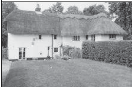
Frame 4: S elevation looking N
