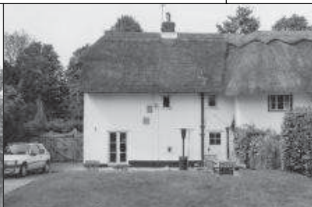
Frame 3: S elevation looking N
