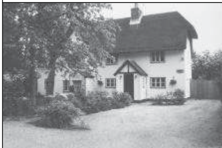
Frame 1: N elevation looking S
