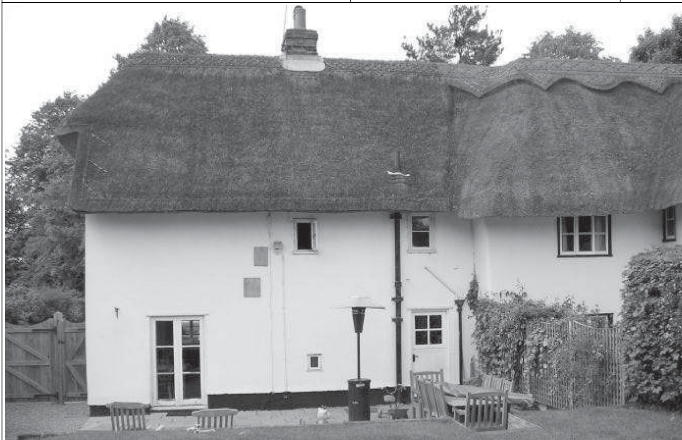
Plate 1: 'Shipwrights Cottage' rear elevation looking N
