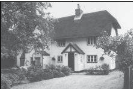
Frame 2: N elevation looking S
