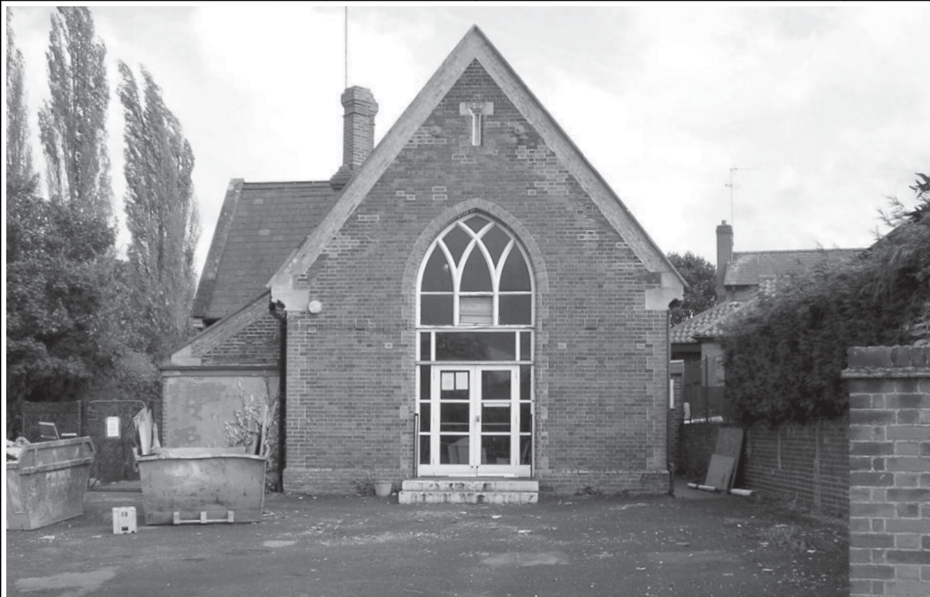
Plate 3: Building 1, western gable end
