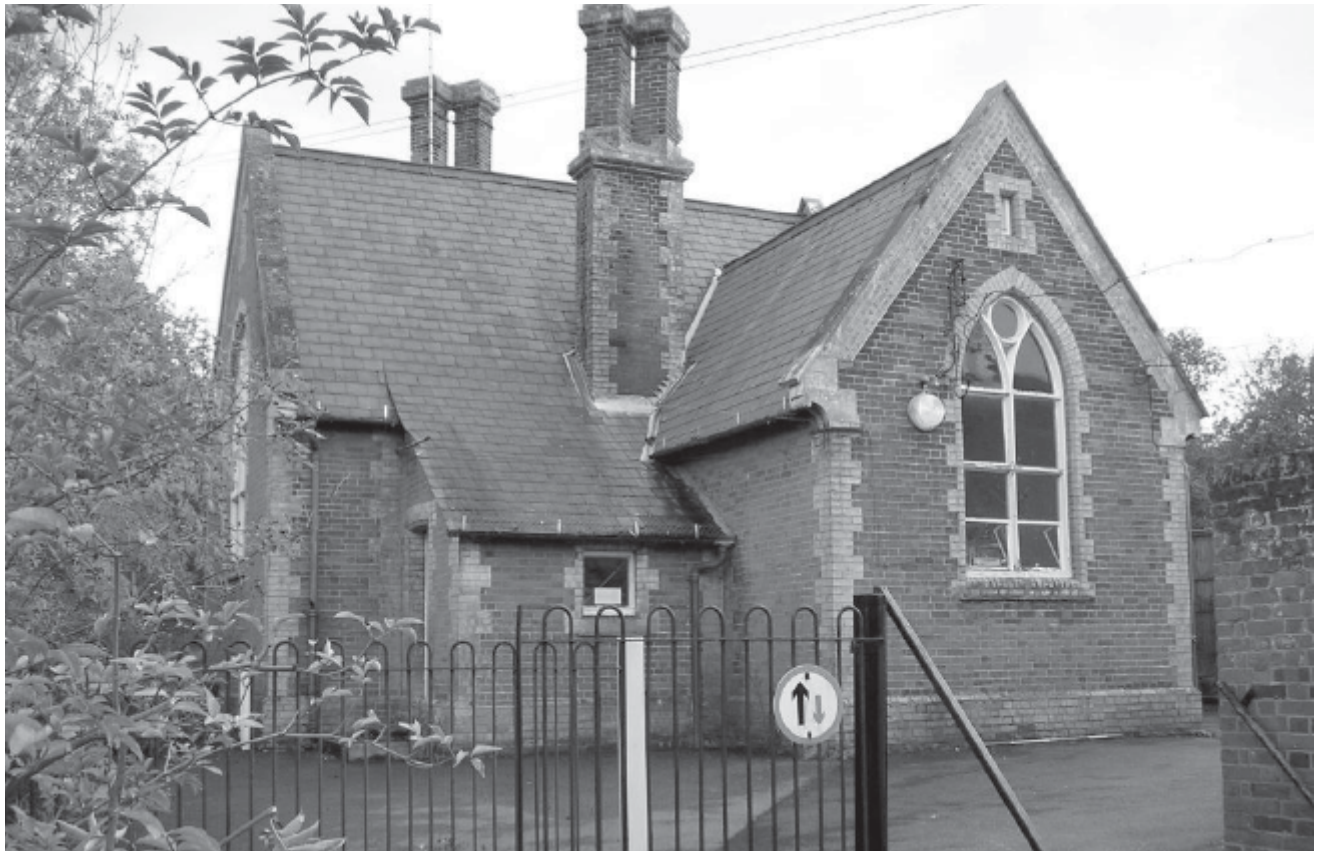
Plate 10: Building 2, western elevation
