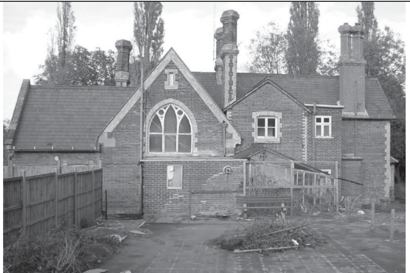
Plate 11: Building 2, southern elevation
