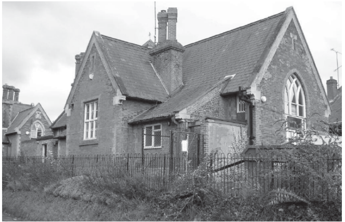
Plate 1: Building 1, northern and western elevations
