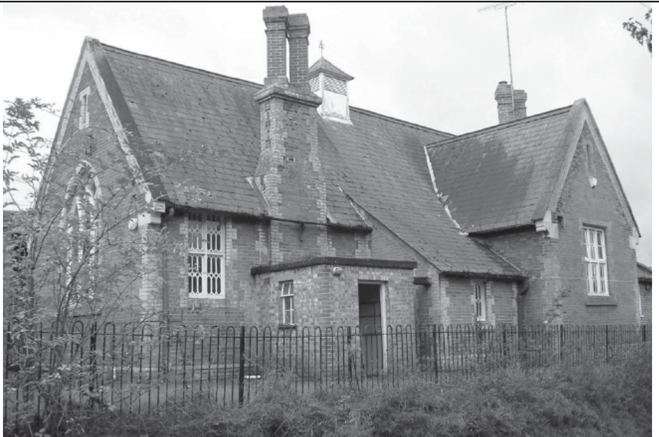
Plate 2: Building 1, northern and eastern elevations
