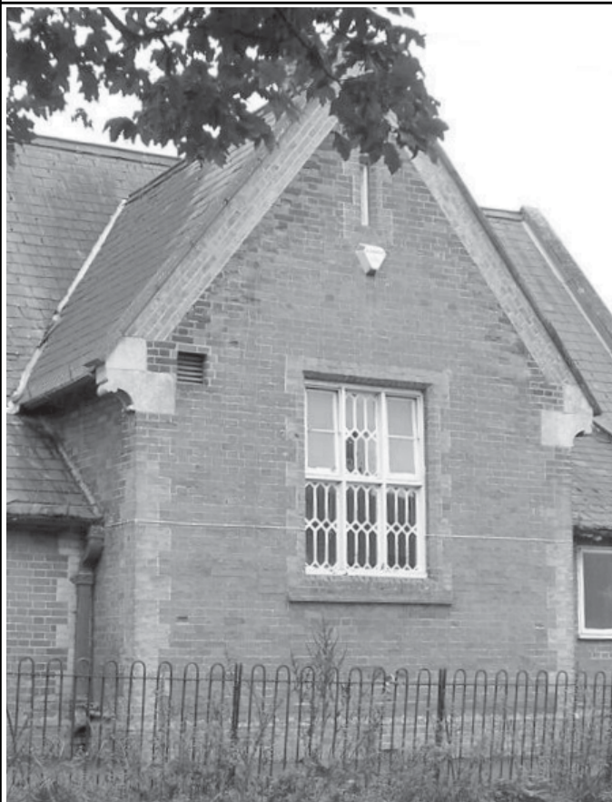
Plate 4: Building 1, central extension
