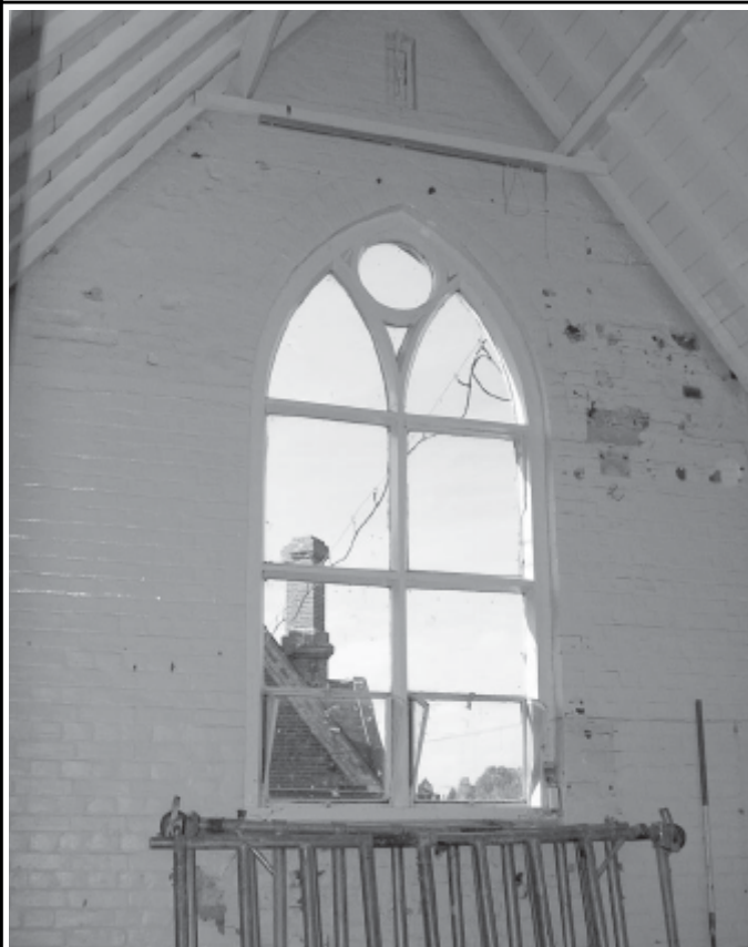
Plate 15: Building 2, ante-room window
