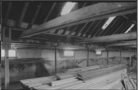
Frame 9: Interior, facing WNW
