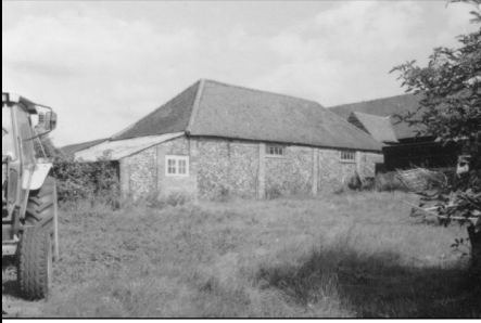
Frame 1: E exterior elevation, facing NW
