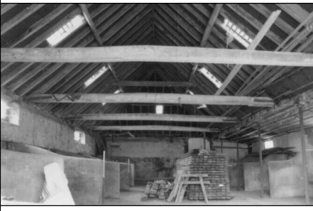
Frame 14: Interior and roof, facing S
