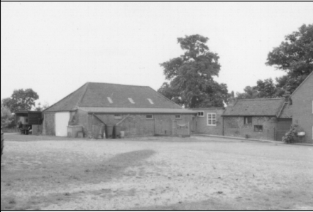
Frame 5: W exterior elevation and bakery range, facing SE
