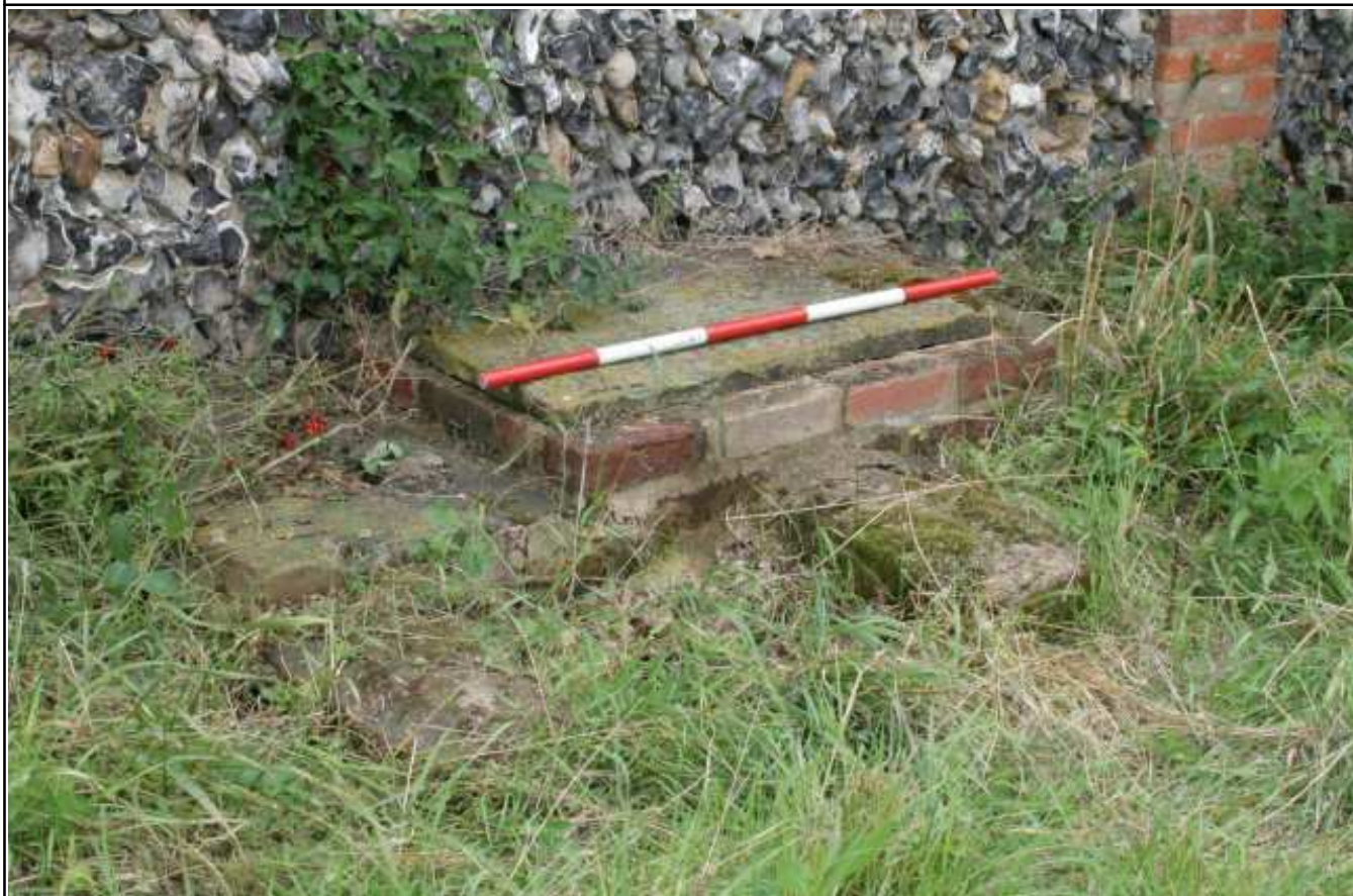
Plate 4: Exterior. East elevation, drain
