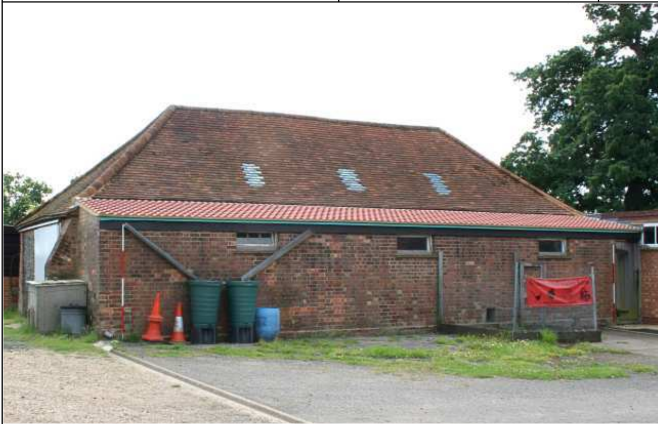
Plate 3: Exterior. West elevation
