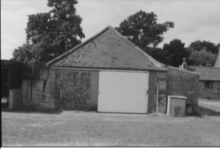
Frame 2: N exterior elevation facing S
