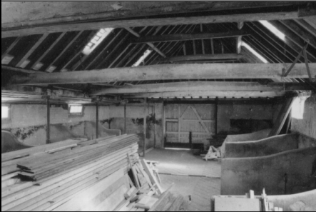
Frame 7: Interior, facing NNW
