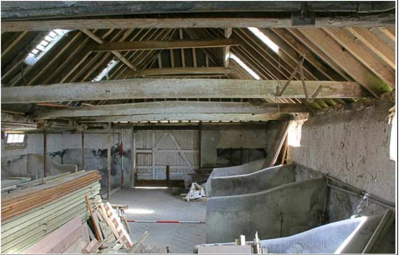
Plate 5: Interior. View looking north
