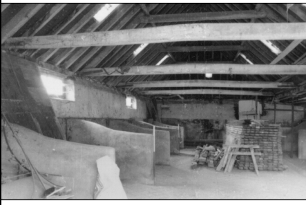
Frame 13: Interior, facing SE
