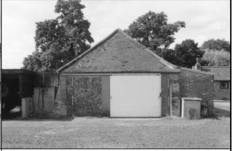
Frame 3: N exterior elevation facing S
