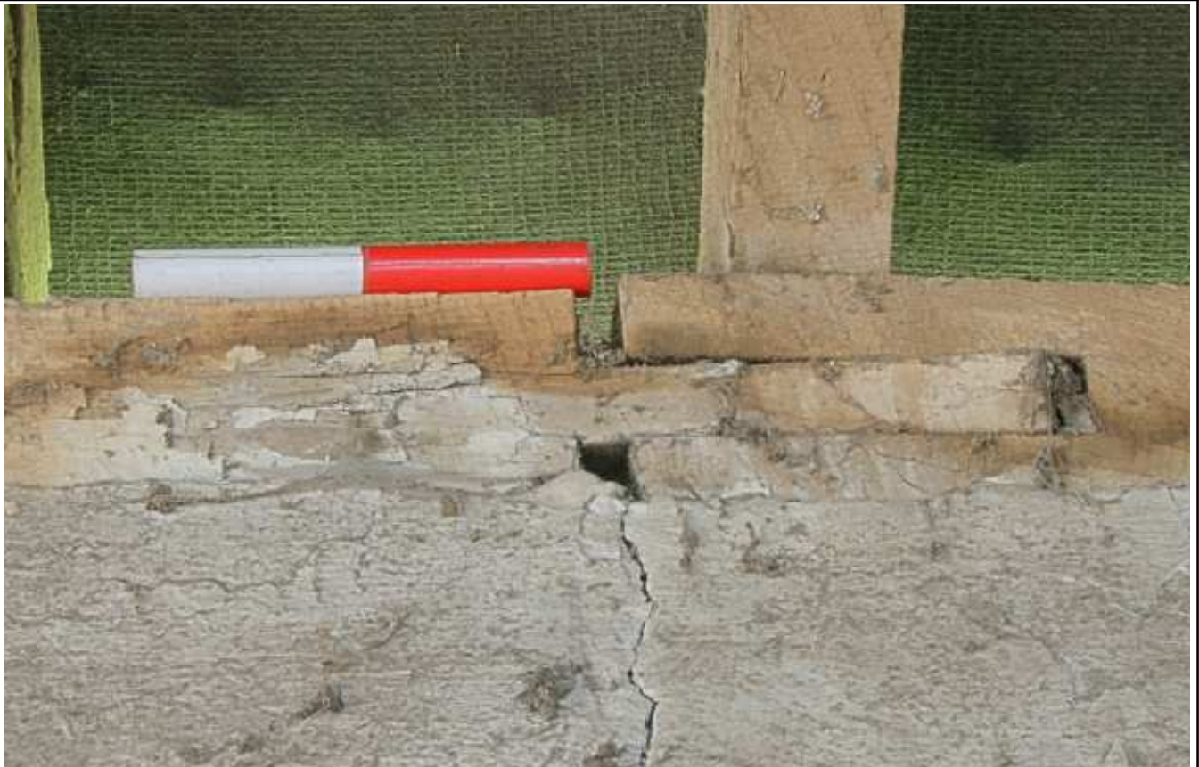
Plate 9: Interior. East elevation, wall plate joint in stall 8
