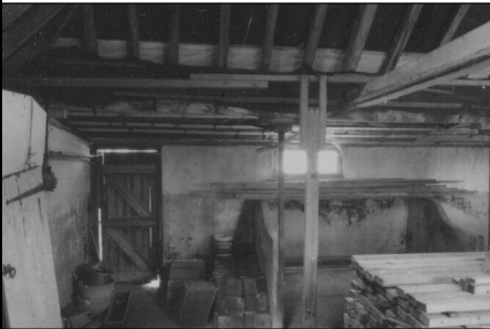
Frame 10: Interior, W elevation S end, facing W
