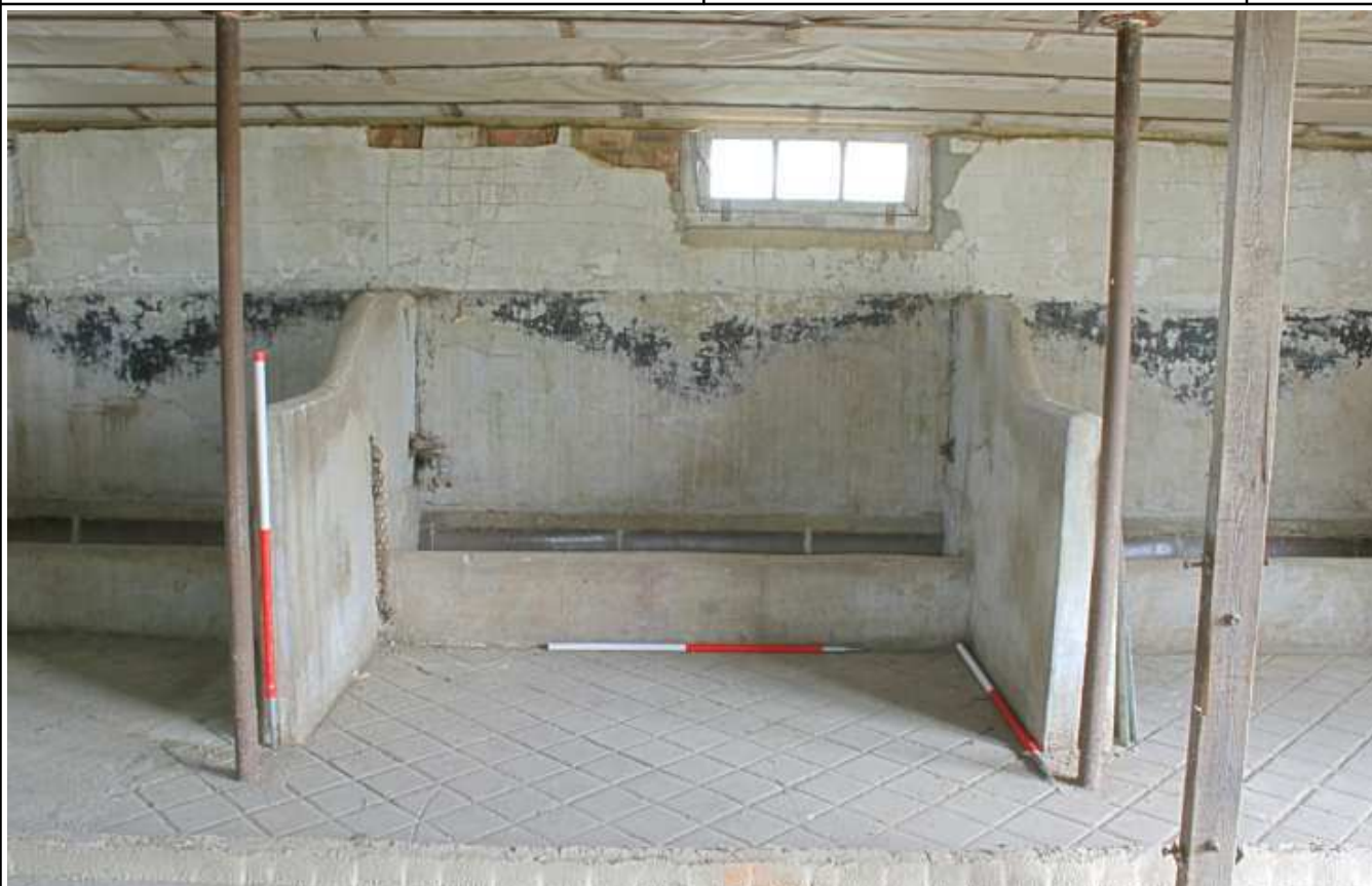
Plate 7: Interior. Stall 2 looking west
