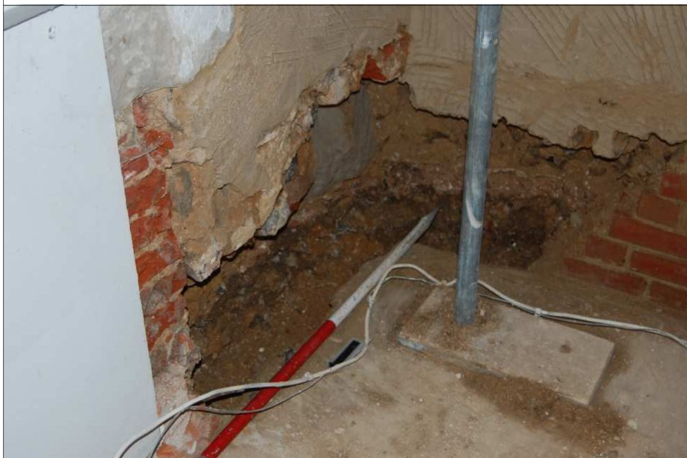
Plate 2: Underpinning east corner, looking southeast.
