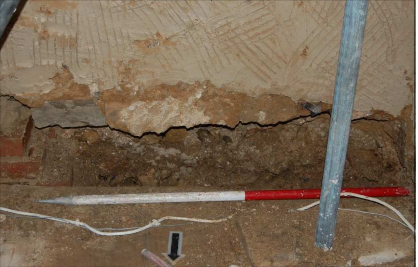
Plate 3: Underpinning west corner, looking south.
