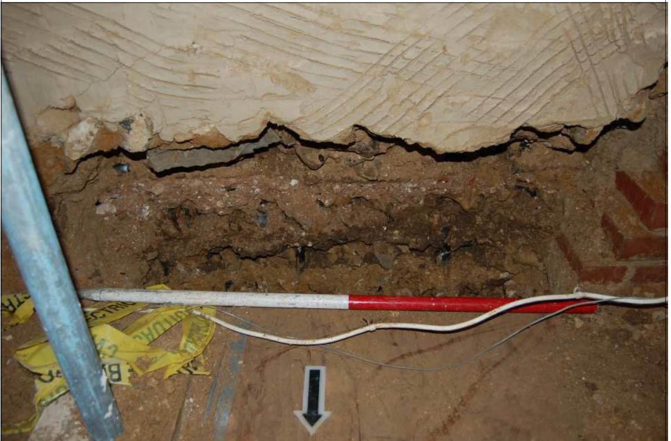
Plate 4: Underpinning under stone arch, looking south.
