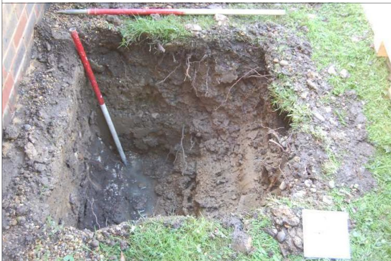
Plate 2: TP2 looking west
