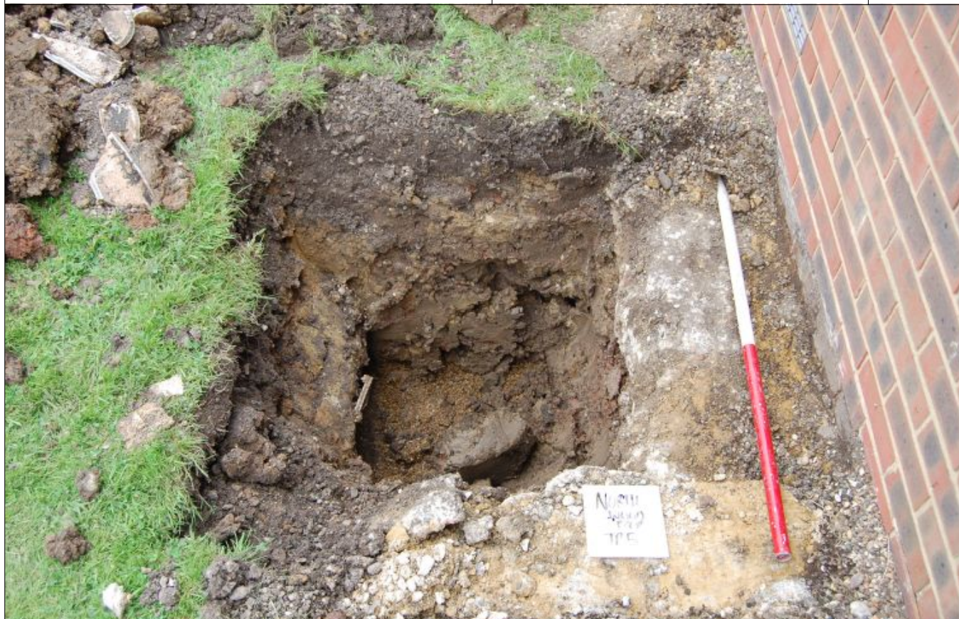
Plate 5: TP5 looking east
