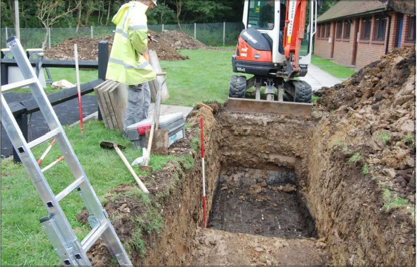
Plate 7: Trench 1 during excavation, looking east
