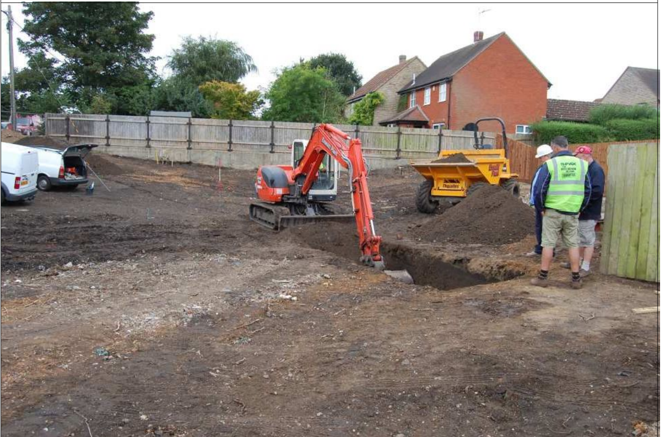
Plate 2: General site view, looking west
