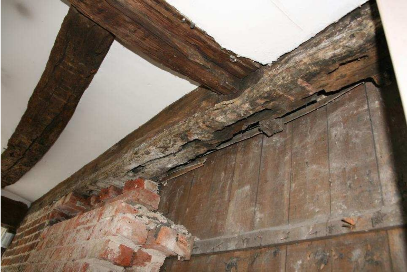
Plate 07 - Storey plate in E elevation of No2, showing mortice holes
