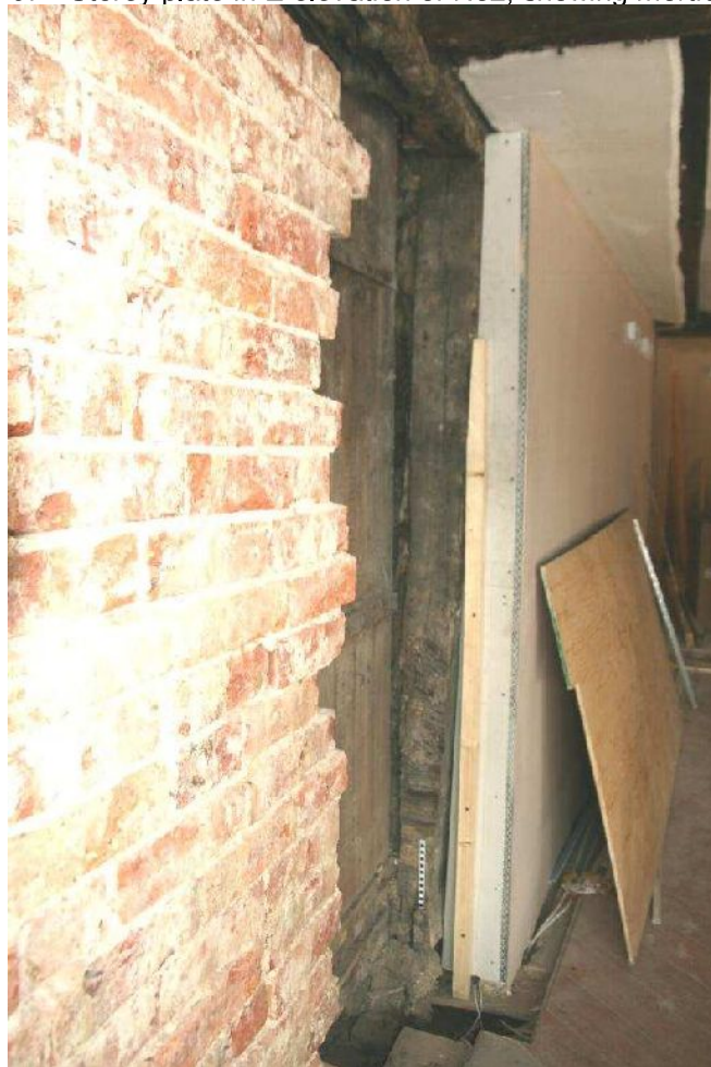
Plate 08 - In situ studwork adjacent to opening in E elevation of No2
