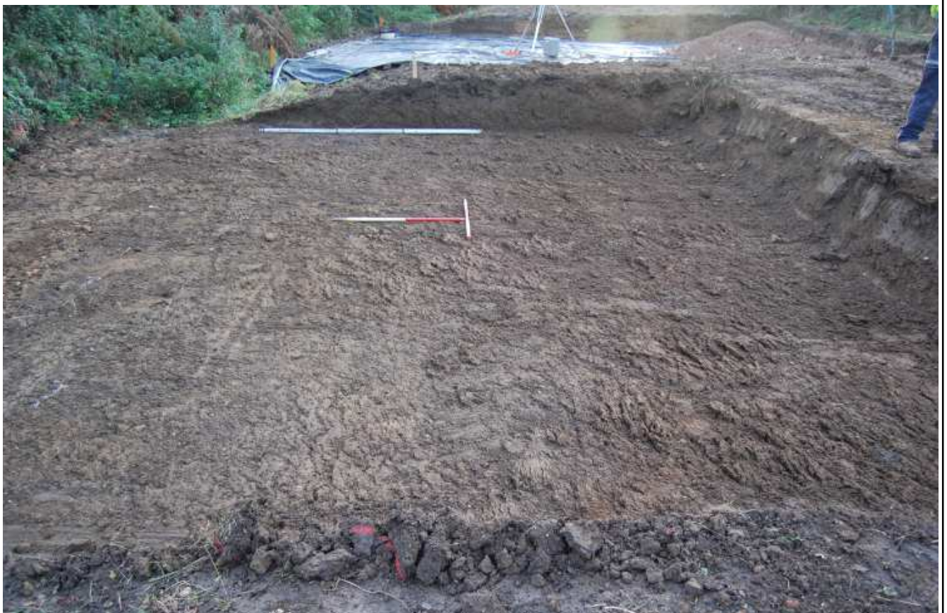
Plate 4: Plot 1 garage, looking W
