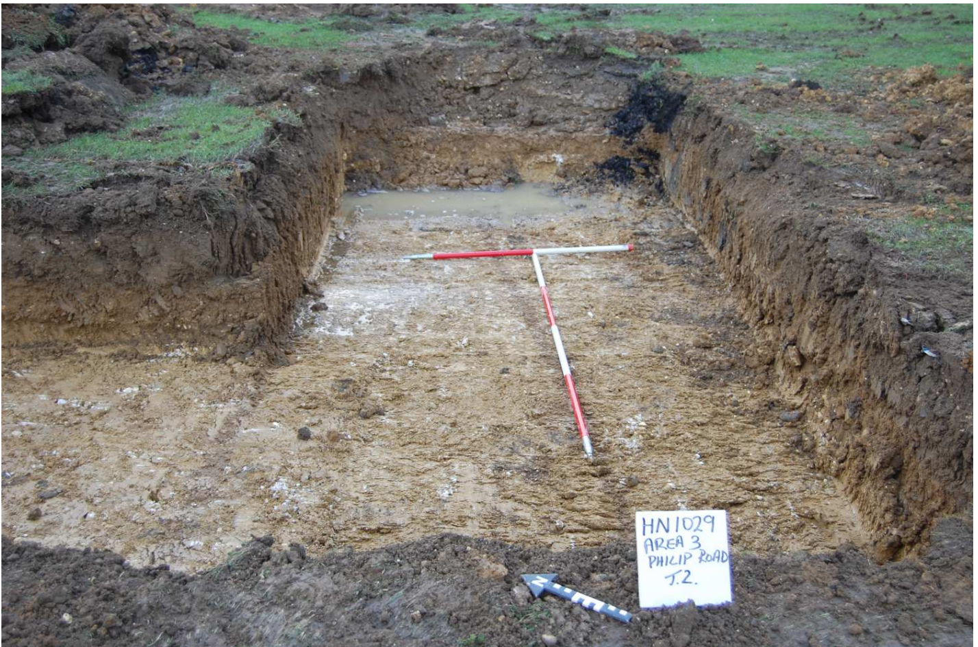
Plate 08 - Philip Road, Tr2, looking E
