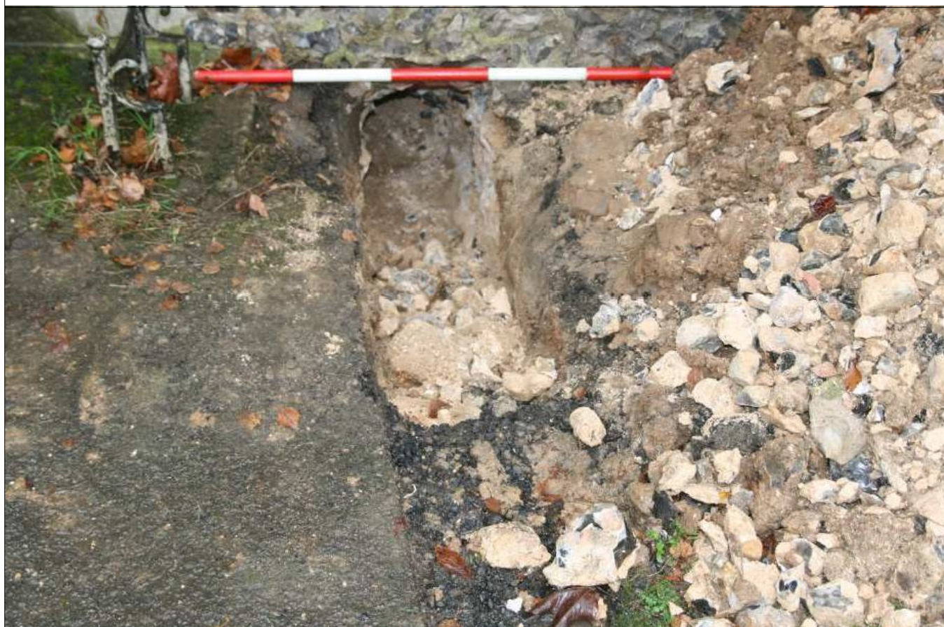
Plate 7: Access hole 1, from the exterior
