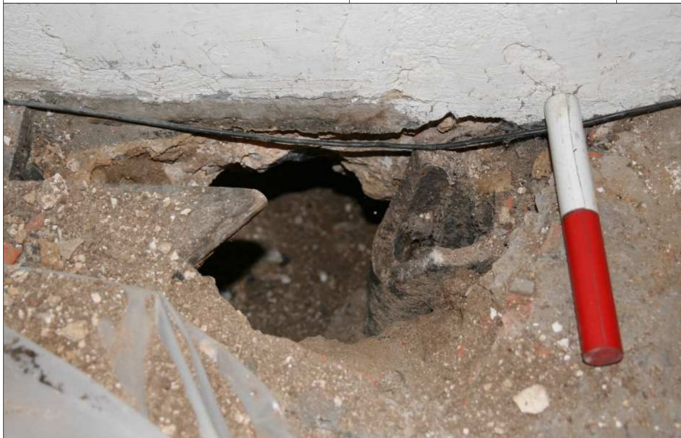
Plate 6: Access hole 1, from the interior
