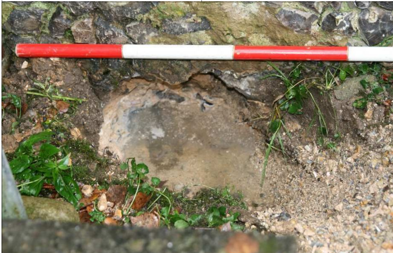
Plate 8: Access hole 2 from the exterior, looking south
