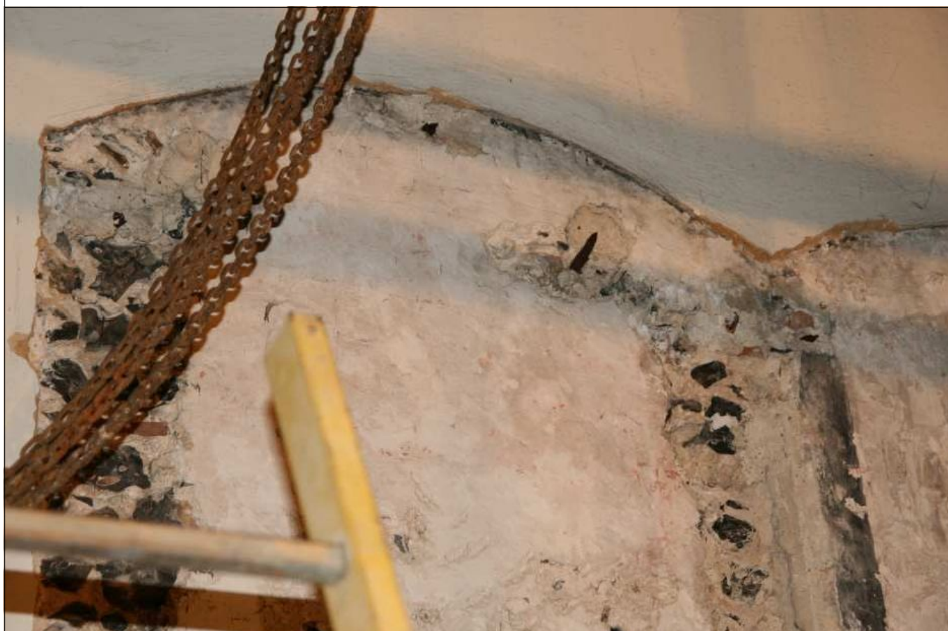
Plate 4: Detail of the exposed flintwork below the left hand memorial
