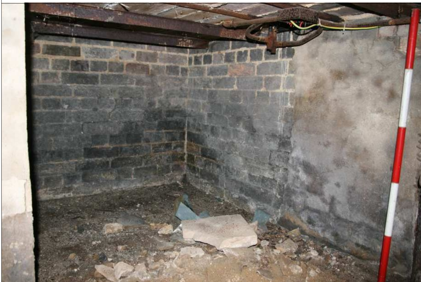
Plate 18: North & east interior elevations to the boiler room, looking NE
