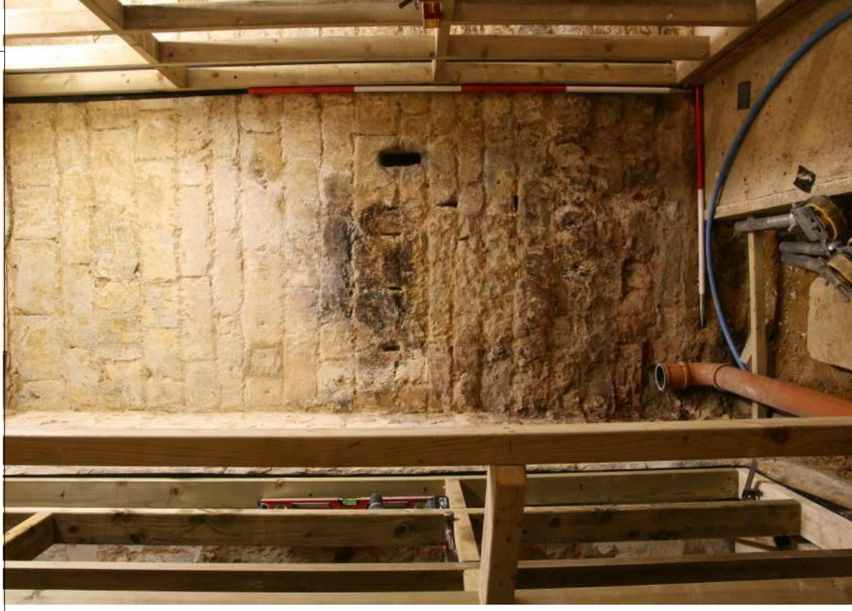
North wall of west tower, looking N
