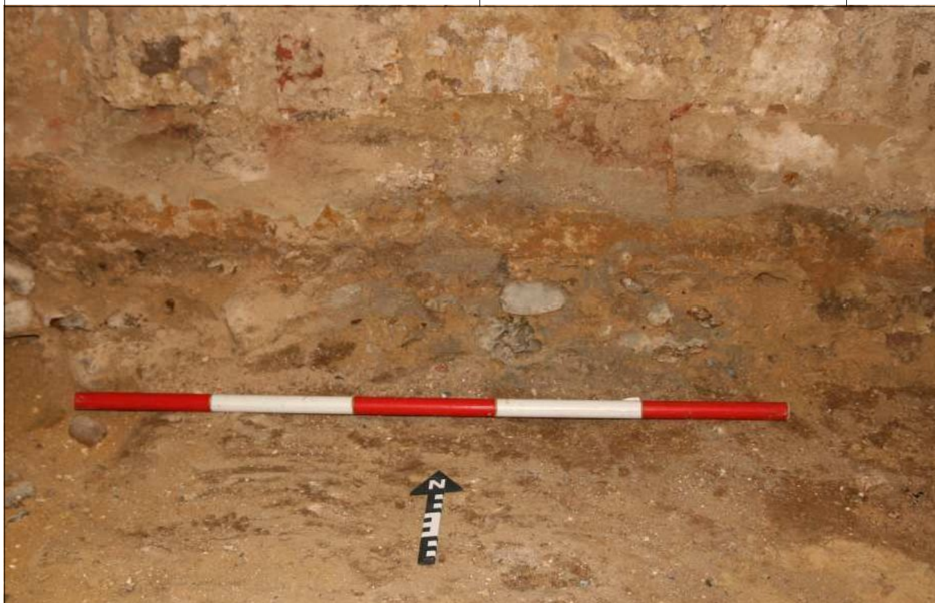
Plate 15: North wall west tower, central section below the stonework showing [24]
