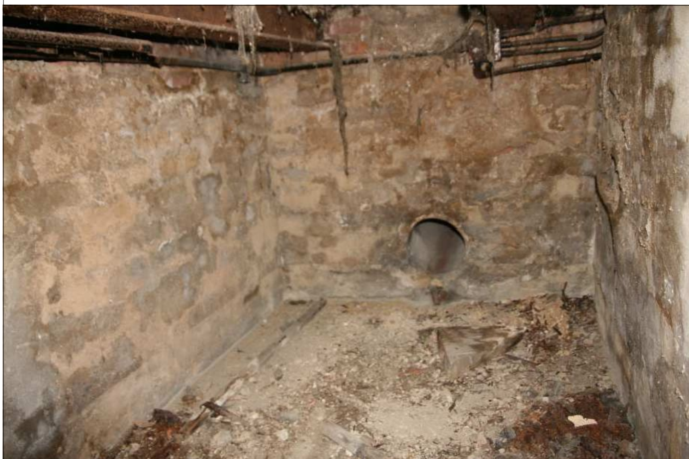
Plate 20: West elevation of structure [2], showing air inlet pipe, looking W
