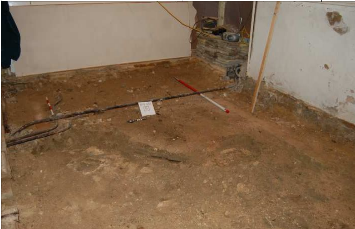
Plate 23: Brick sleeper walls, structure [5], looking east
