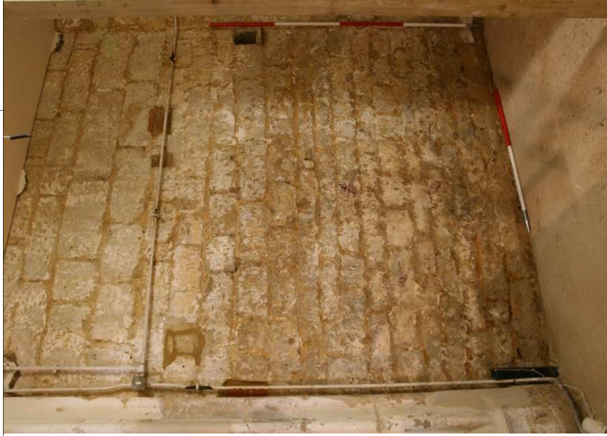
Plate 35: South wall of west tower, looking SW
