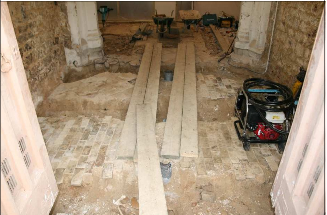
Plate 8: Paved surfaces within west tower, looking east
