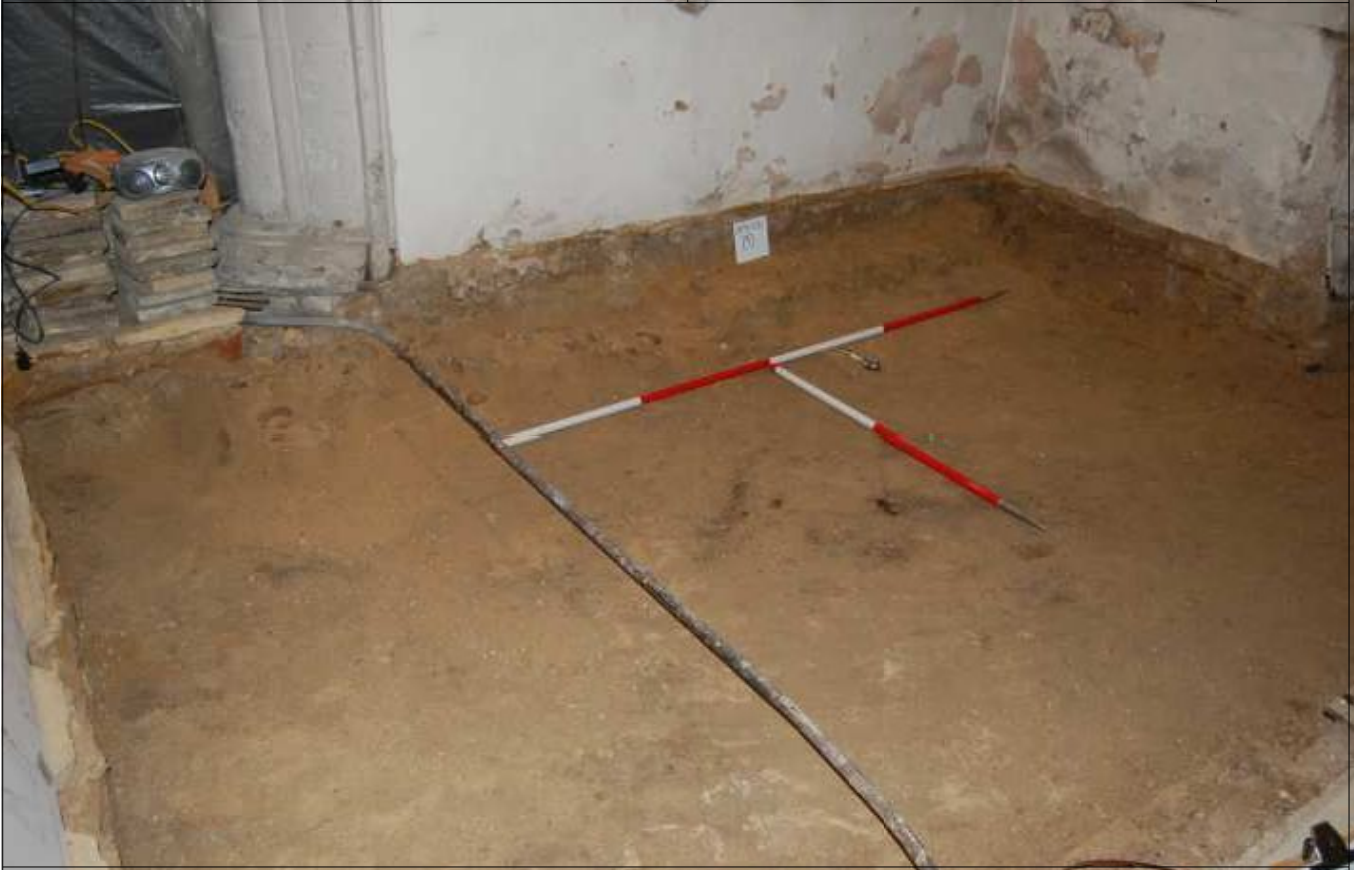
Plate 27: Foundation [4], looking south-west
