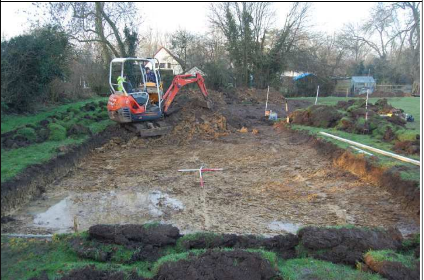
Plate 2: View across the site after ground reduction, looking NW
