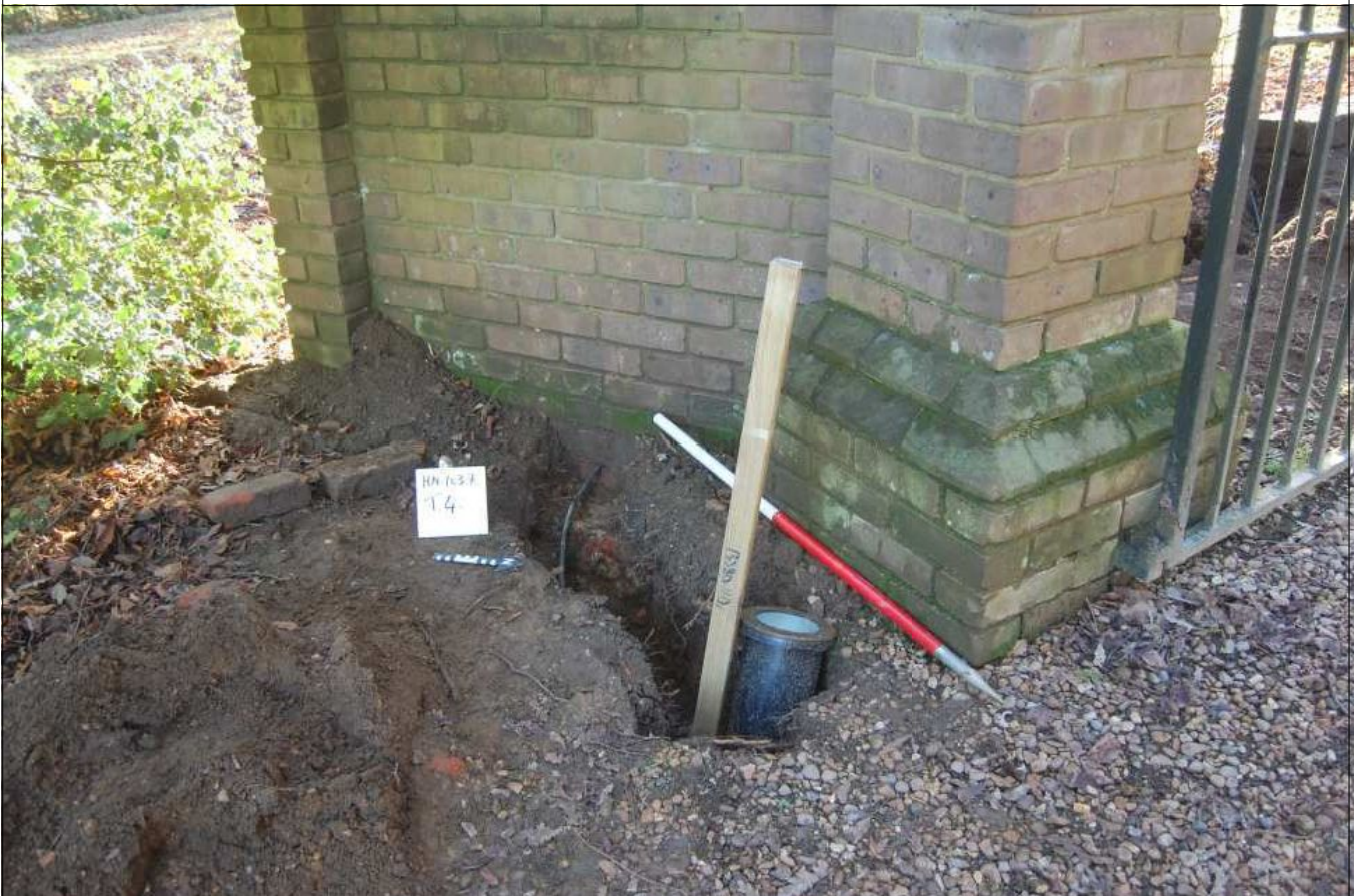
Plate 4: Cable trench 4, looking southwest.
