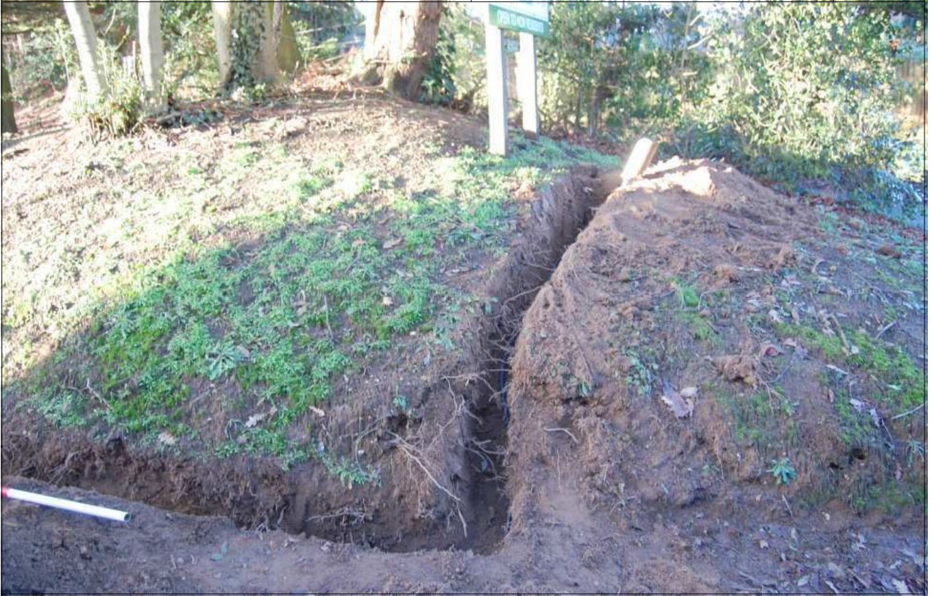
Plate 3: Cable trench 3, looking northwest.
