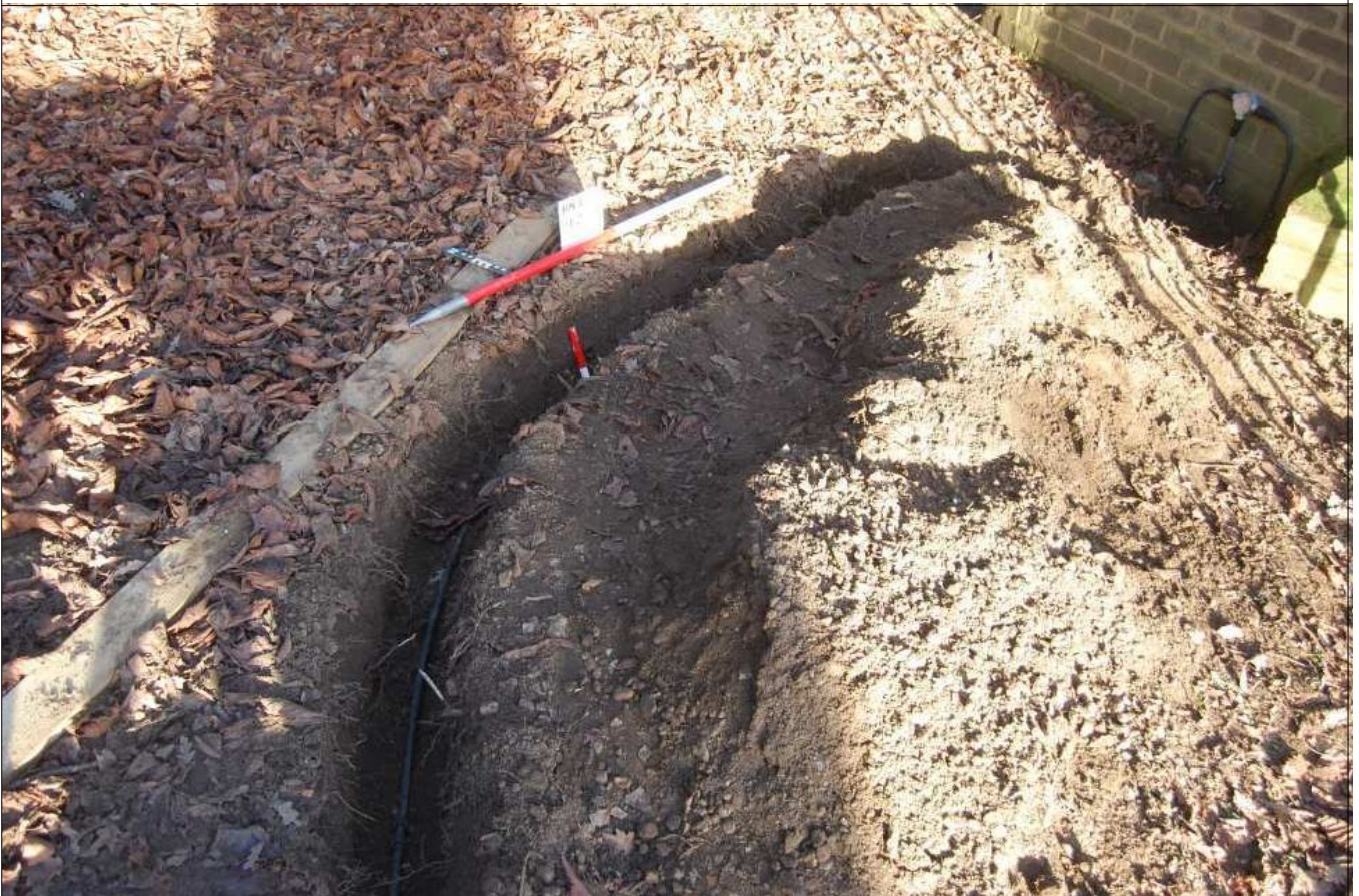
Plate 2: Cable trench 2, looking northeast.
