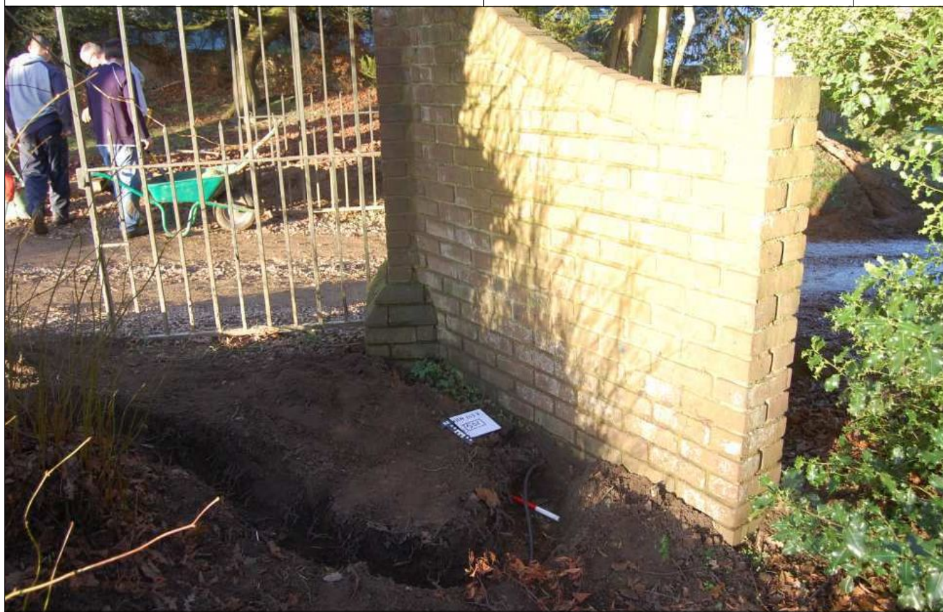
Plate 5: Cable trench 5, looking north.
