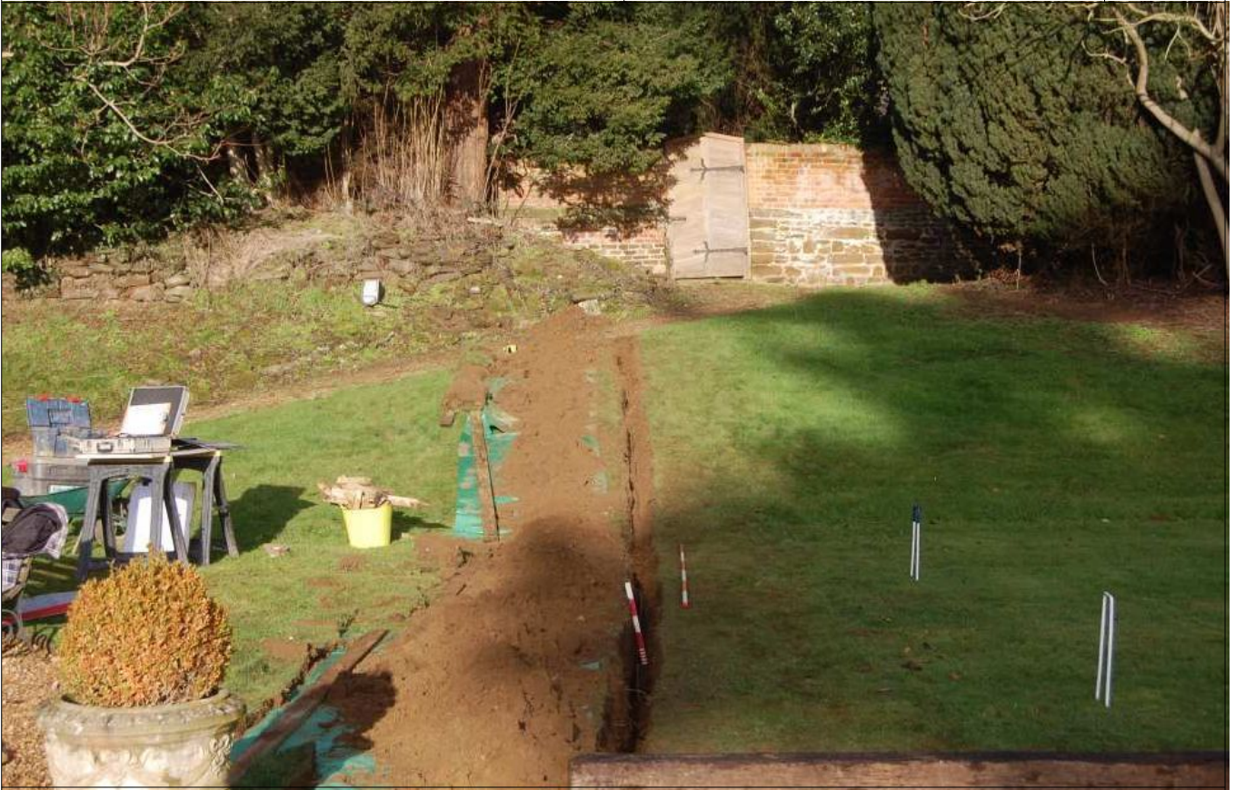
Plate 1: Cable trench 1, looking northwest.
