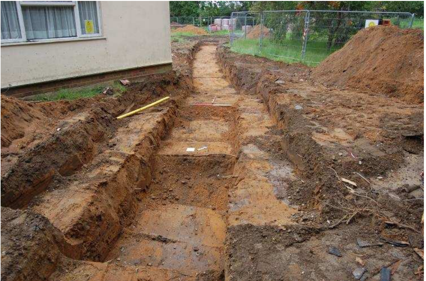
Plate 32 - Tr.23, looking SE
