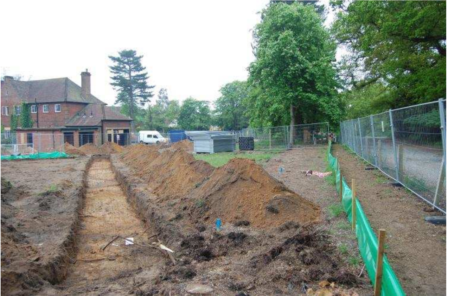
Plate 09 - Tr.6, looking W
