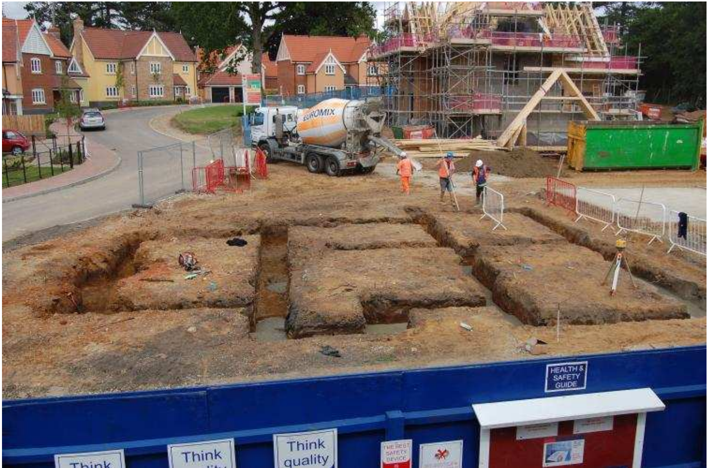
Plate 35 - Foundation trenches to Plot 24, looking N
