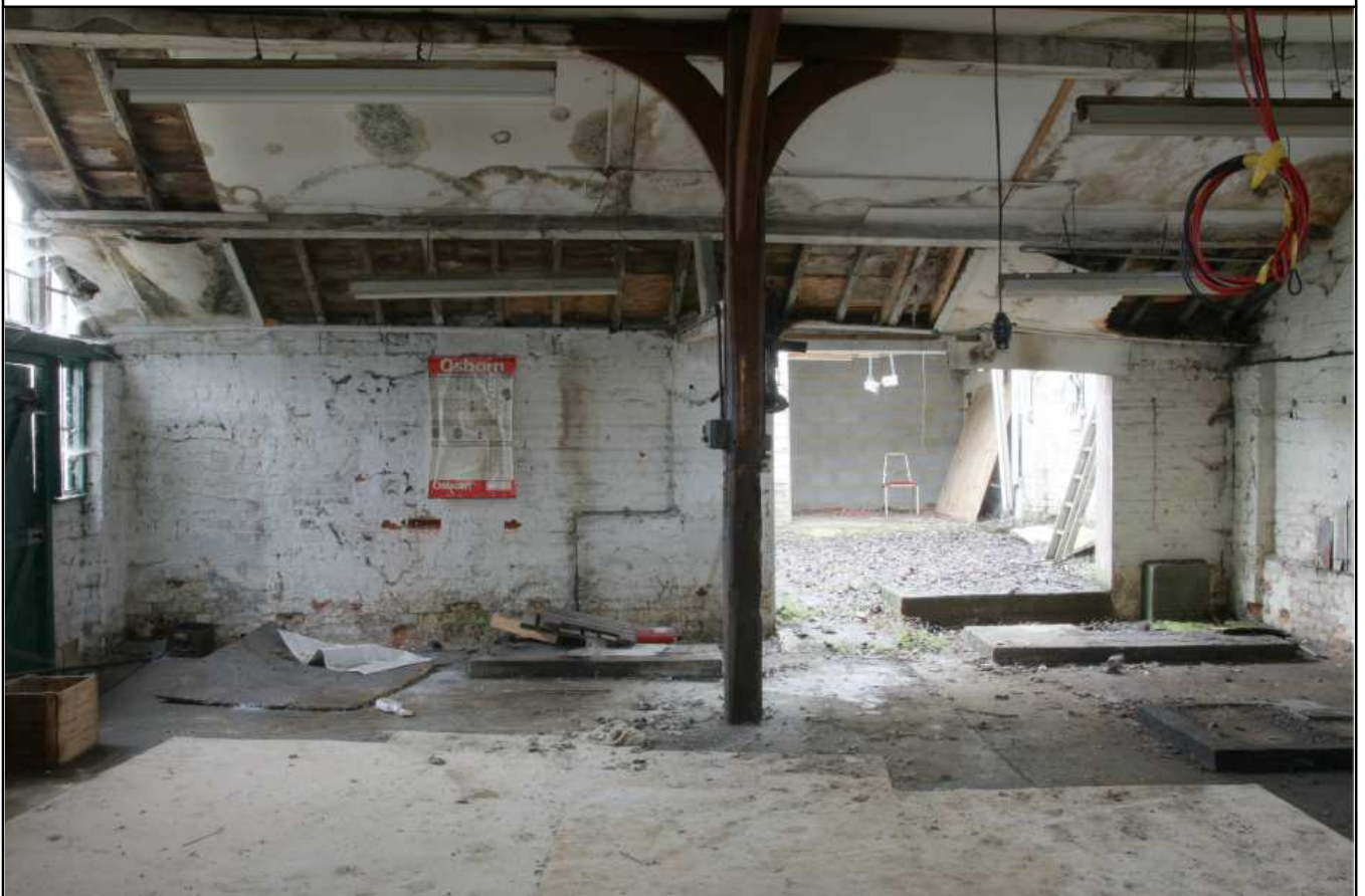
Plate 10: Building 3, looking SE, showing the aisle post
