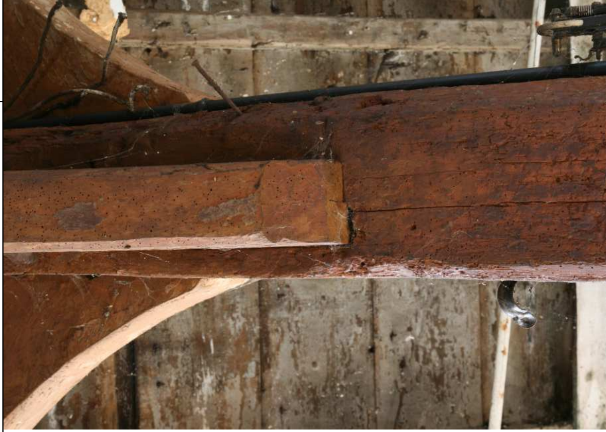
Plate 13: Building 3, detail of SE face of aisle post, showing offset mortice
