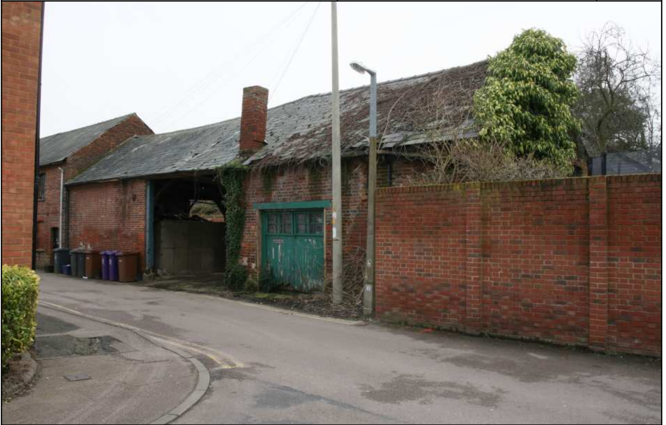
Plate 9: Buildings 2 & 3, NW elevation
