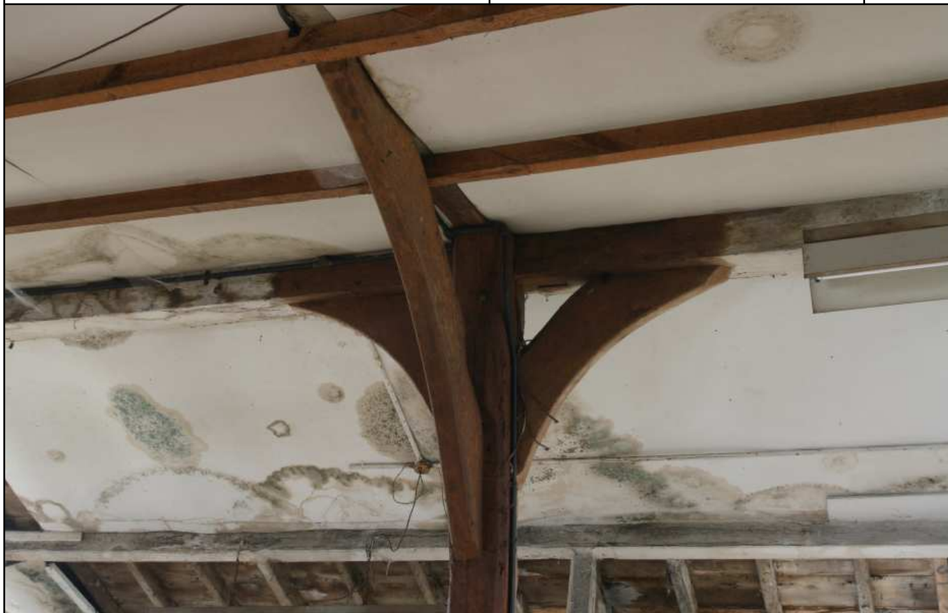
Plate 11: Building 3, detail of jowled post & braces to aisle post
