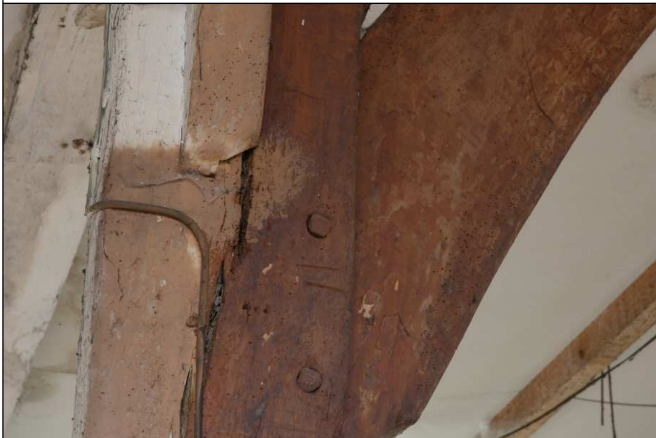
Plate 12: Building 3, detail of carpenter's marks on NE face of aisle post
