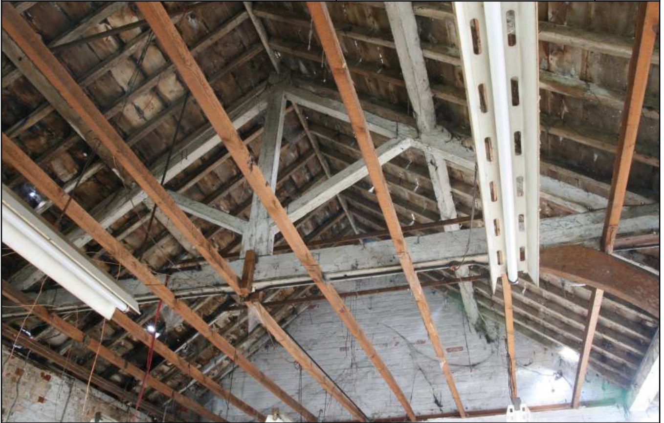
Plate 15: Building 3, roof structure, looking NE
