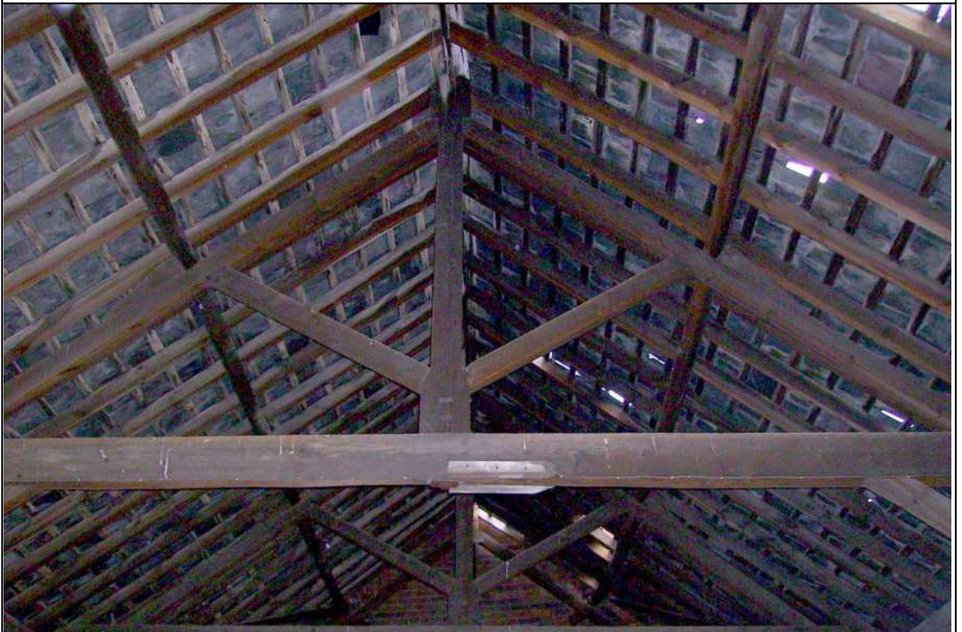
Plate 16: Building 2, roof structure, looking E
