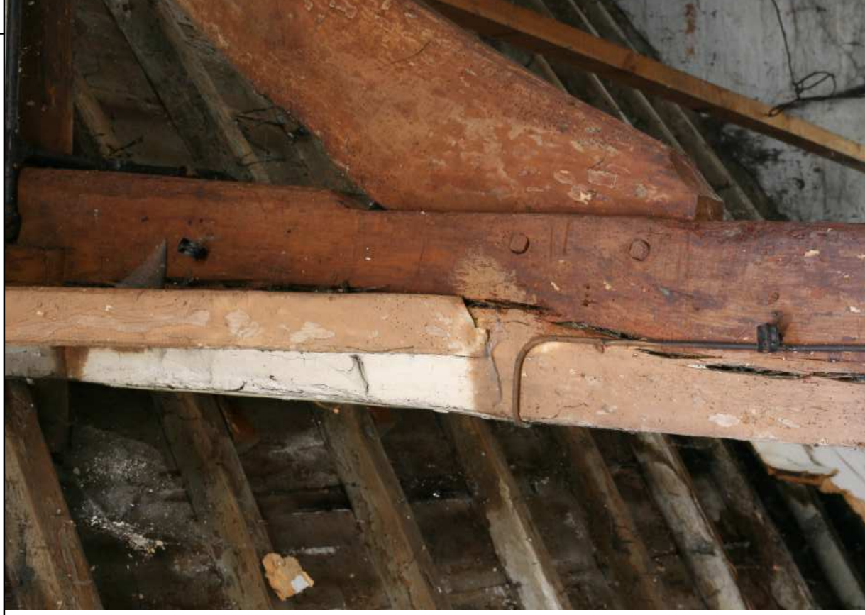
Plate 14: Building 3, detail of NW face of aisle post, showing offset tenon
