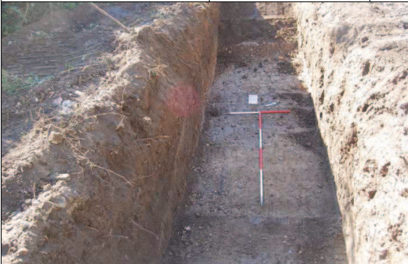
Plate 15: Trench 8b, looking NW
