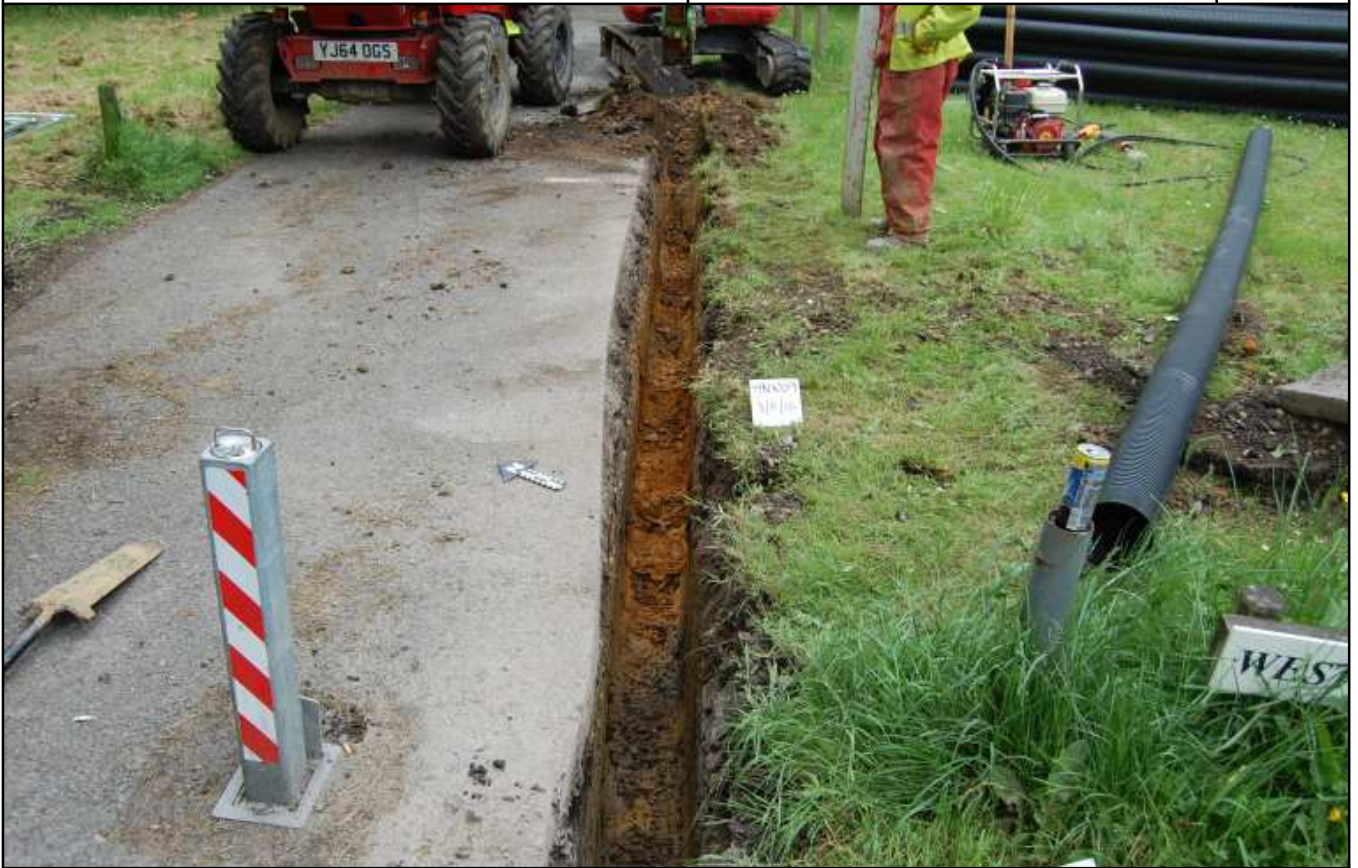
Plate 3: Cable trench: In footpath, southern end, looking northeast
