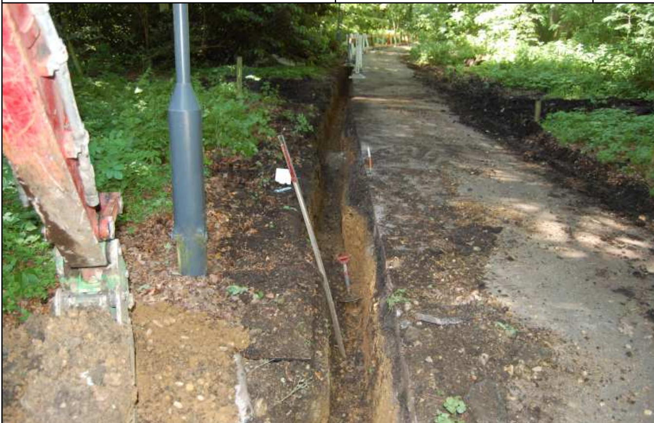
Plate 7: Cable trench, northern section, looking southeast
