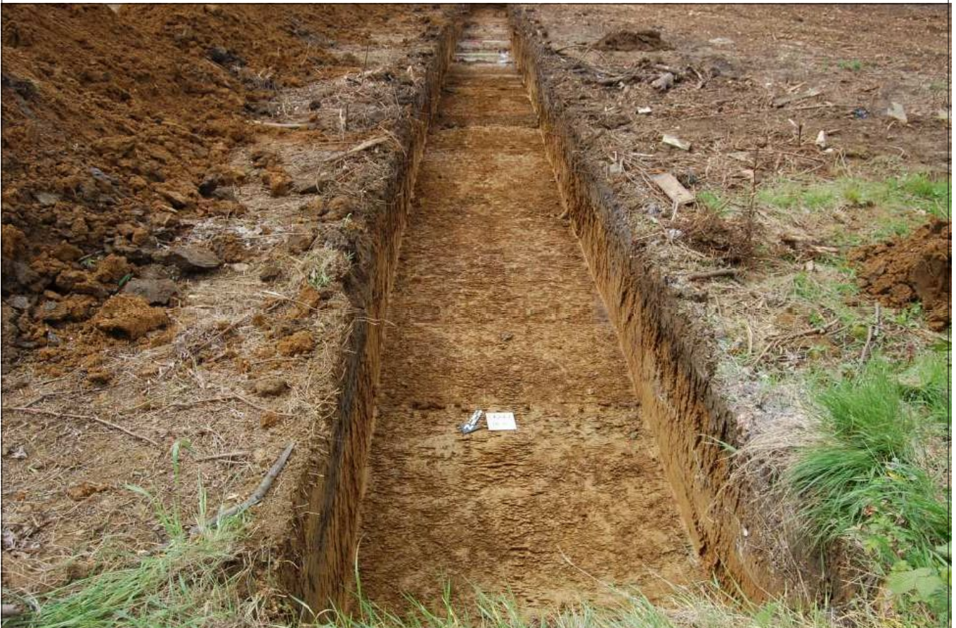
Plate 4: Trench 4, looking southwest.
