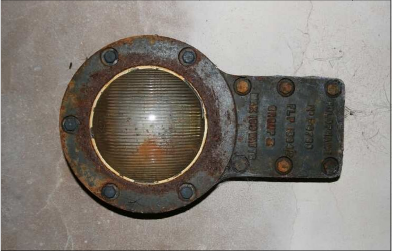
Plate 11: Building 101/7A, detail of light fitting
