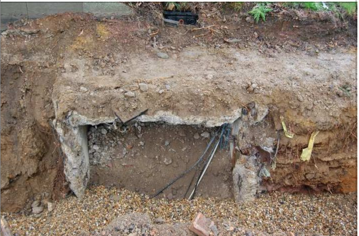
Plate 6: Trench 2, tunnel or duct exposed in the trench, looking SE
