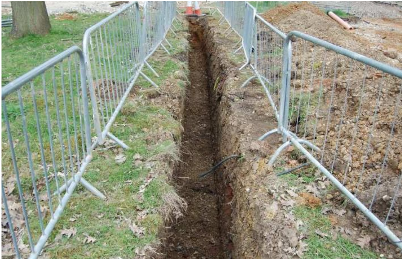
Plate 3: Trench 1, looking NE
