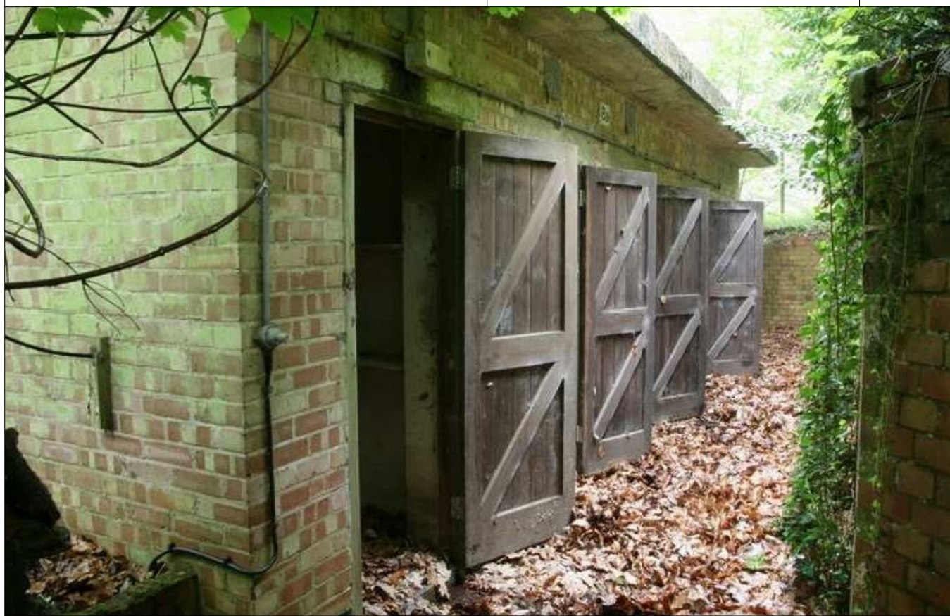
Plate 15: Building 102/8A, detail of the doors, looking SSW
