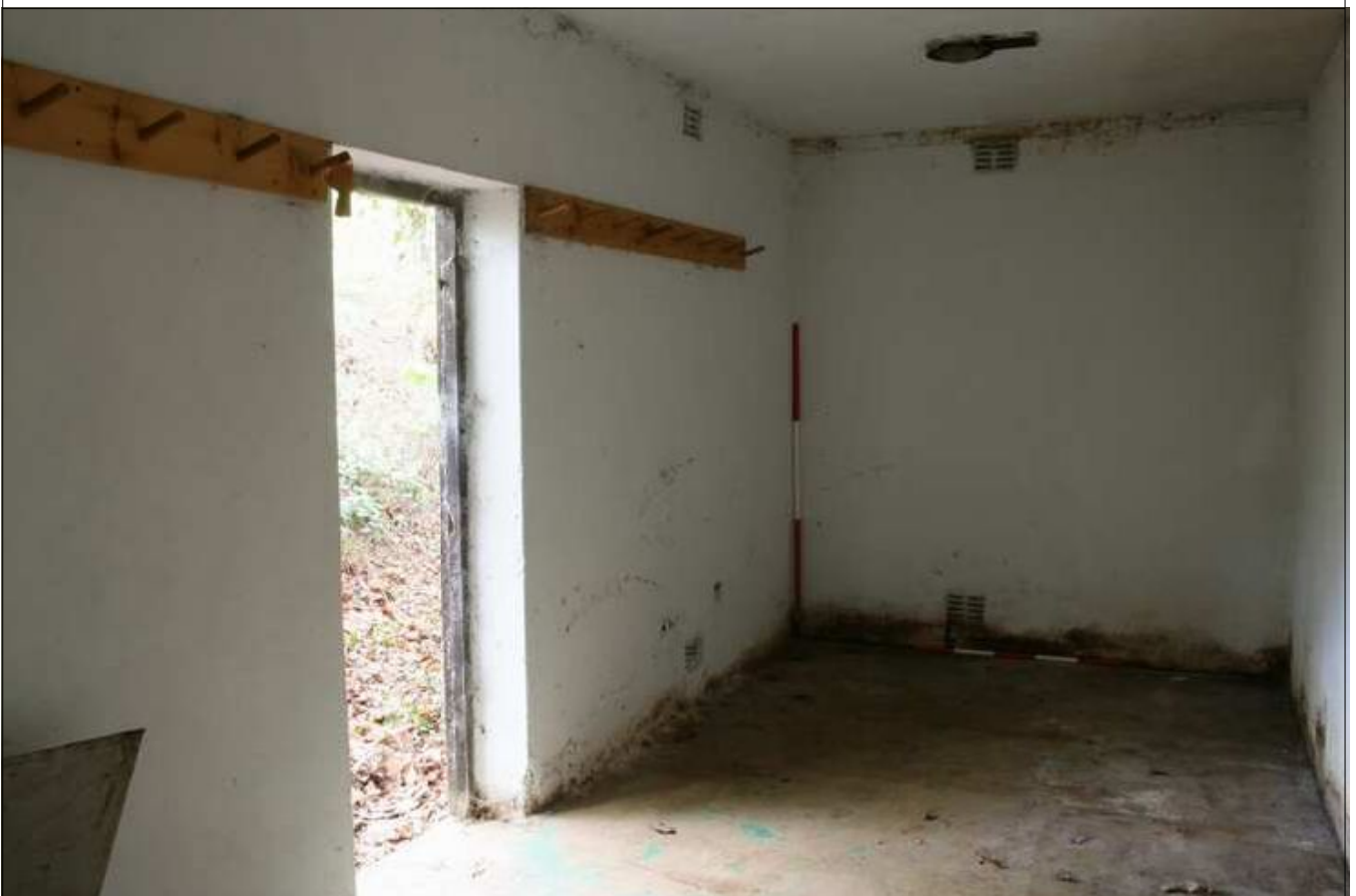
Plate 10: Building 101/7A interior, looking NE
