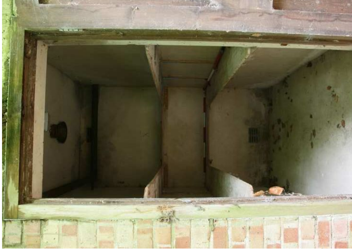
Plate 17: Building 102/8A, looking into Bay 1
