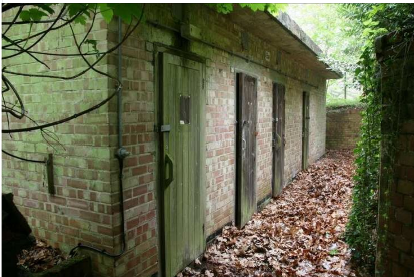
Plate 14: Building 102/8A, NW elevation, looking SSW
