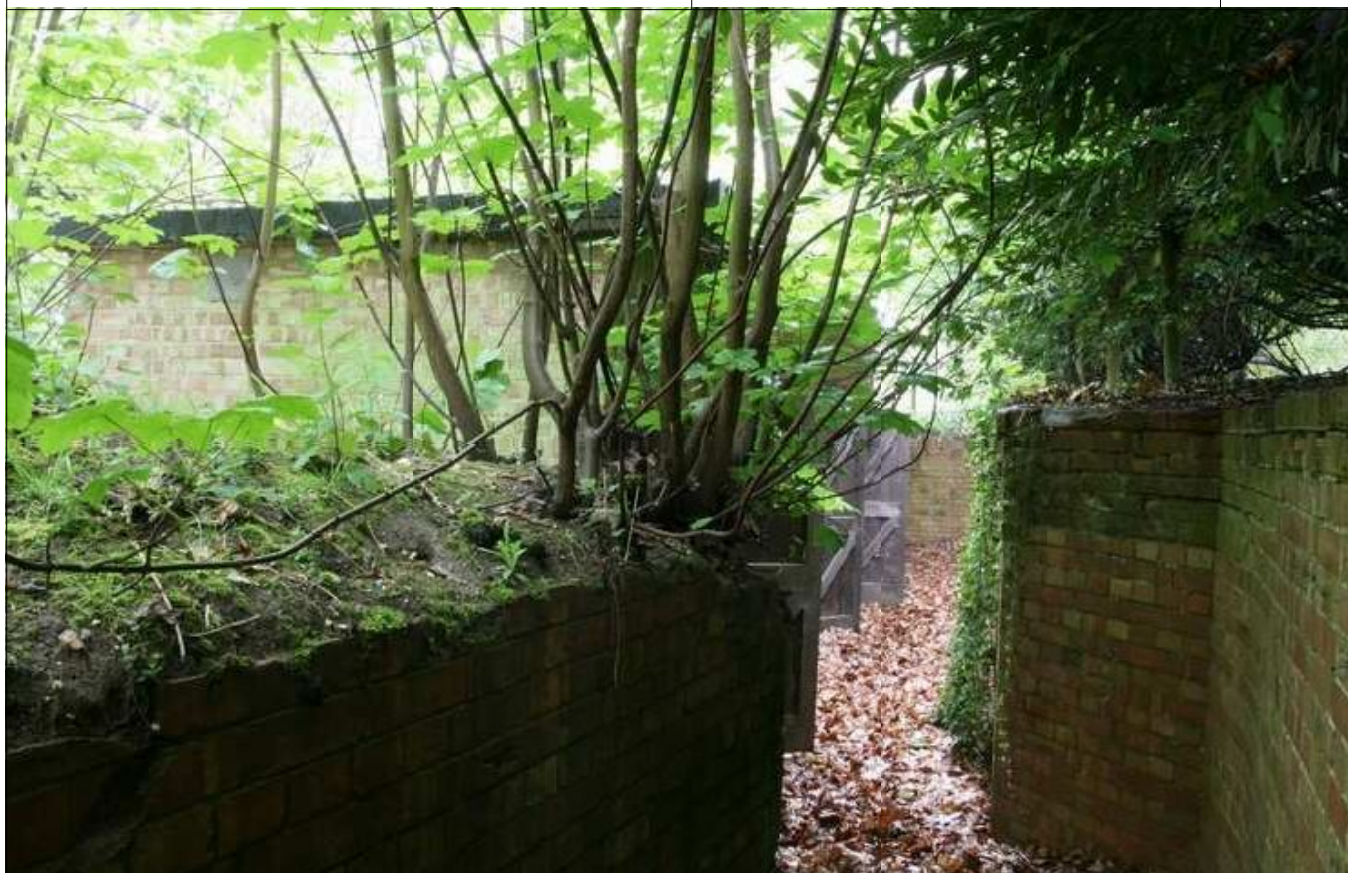
Plate 13: Building 102/8A, detail of retaining wall, looking S
