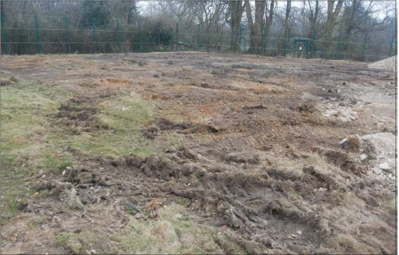
Plate 1: Area of ground reduction prior to start of work, looking NE
