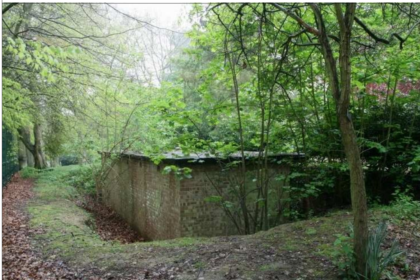
Plate 16: Building 102/8A NE & SE elevations, looking SSW
