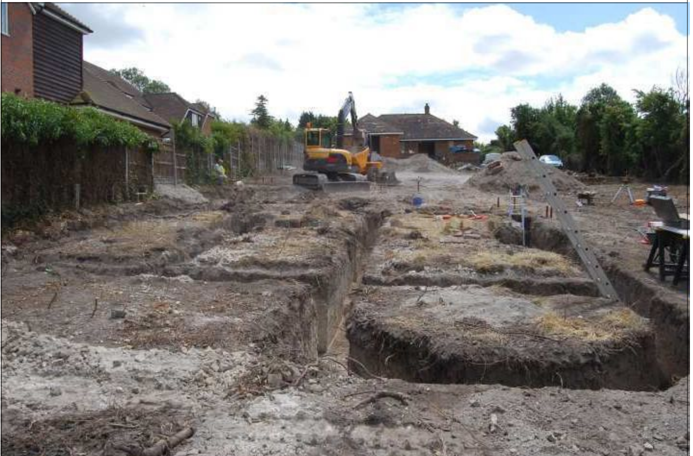
Plate 4: Plot 2, general view, looking SSE
