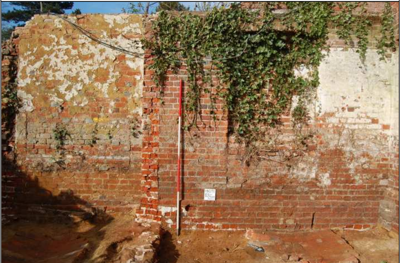
Plate 10: Wall [176], looking south-west
