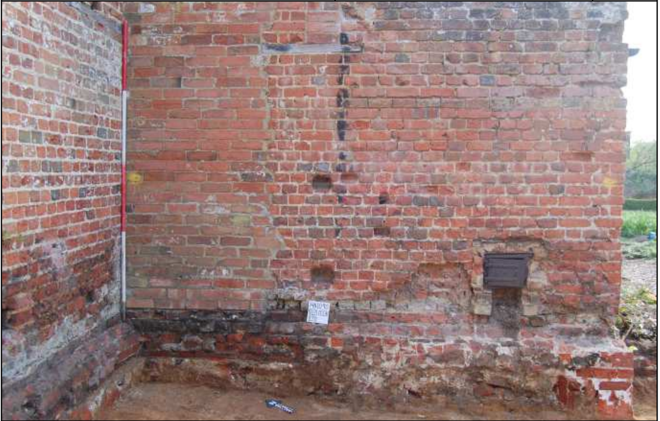
Plate 9: Wall [175], looking north-east
