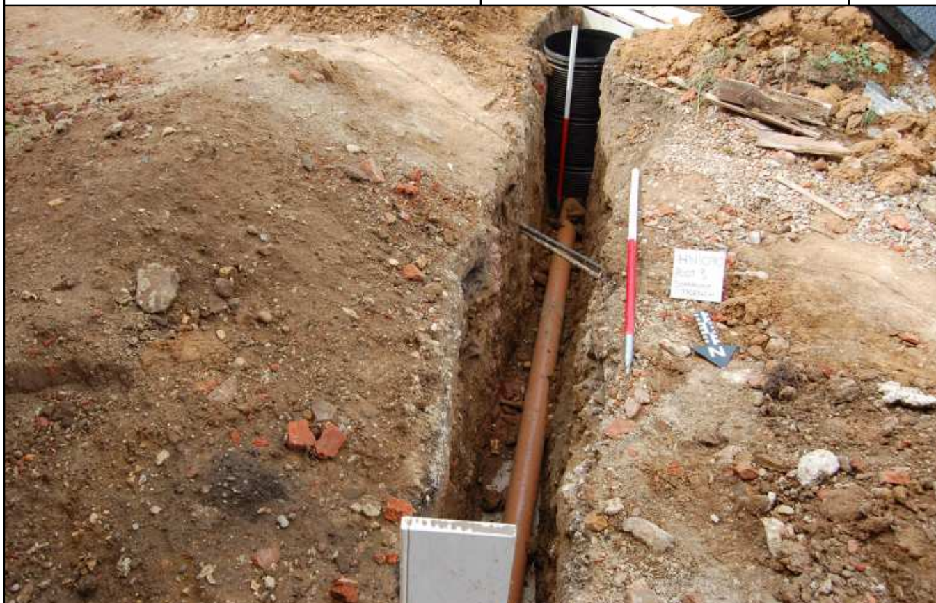
Plate 31: Service trench, Trench 3, looking south
