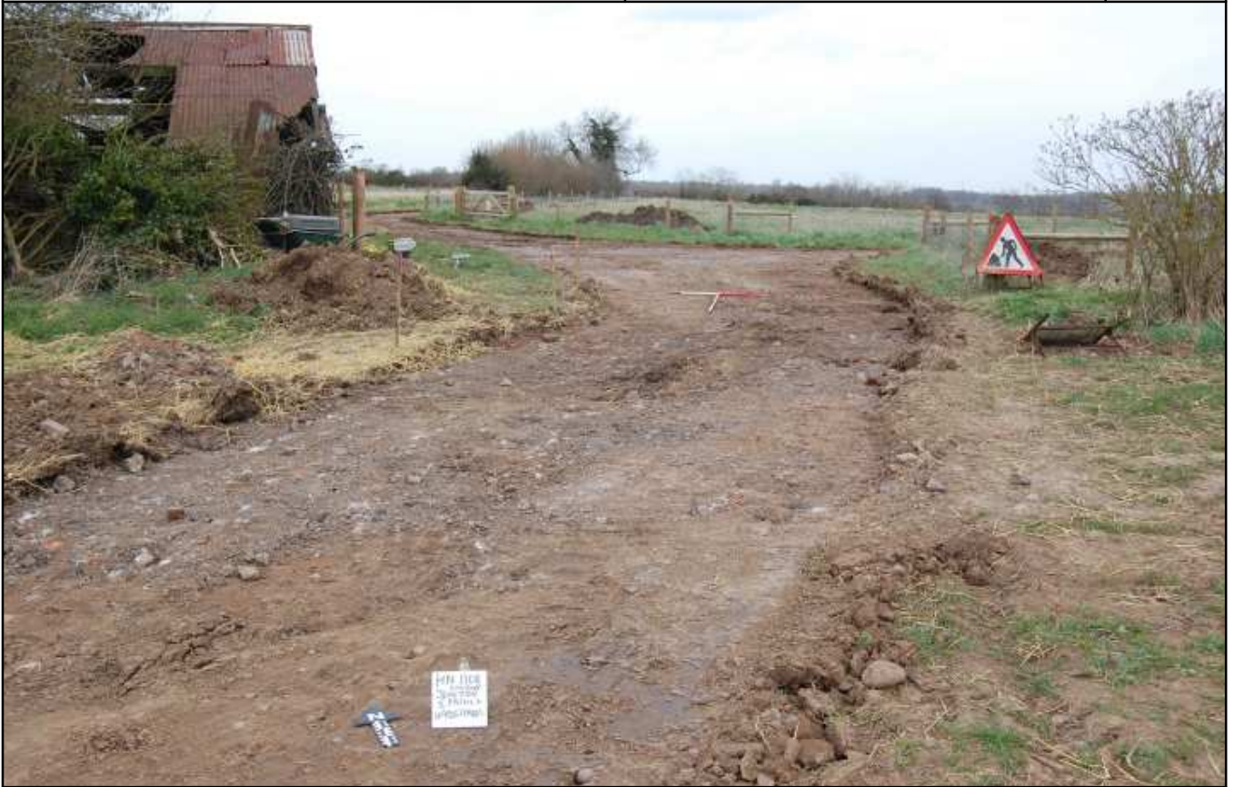
Plate 3: Area of modern intrusion, associated with existing barn, looking N
