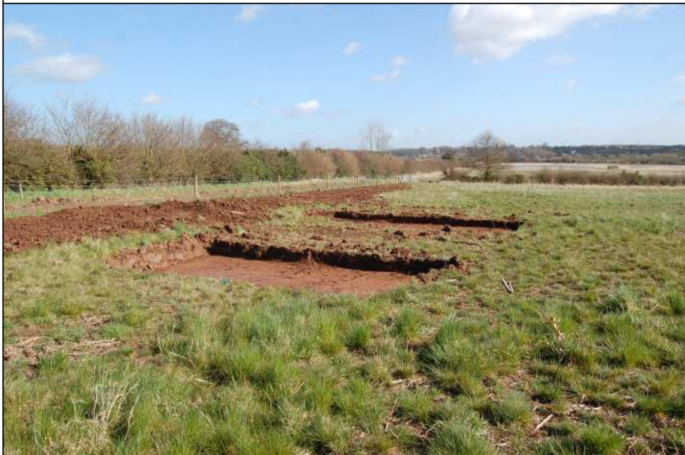
Plate 8: Trenches for art installation bases, looking N
