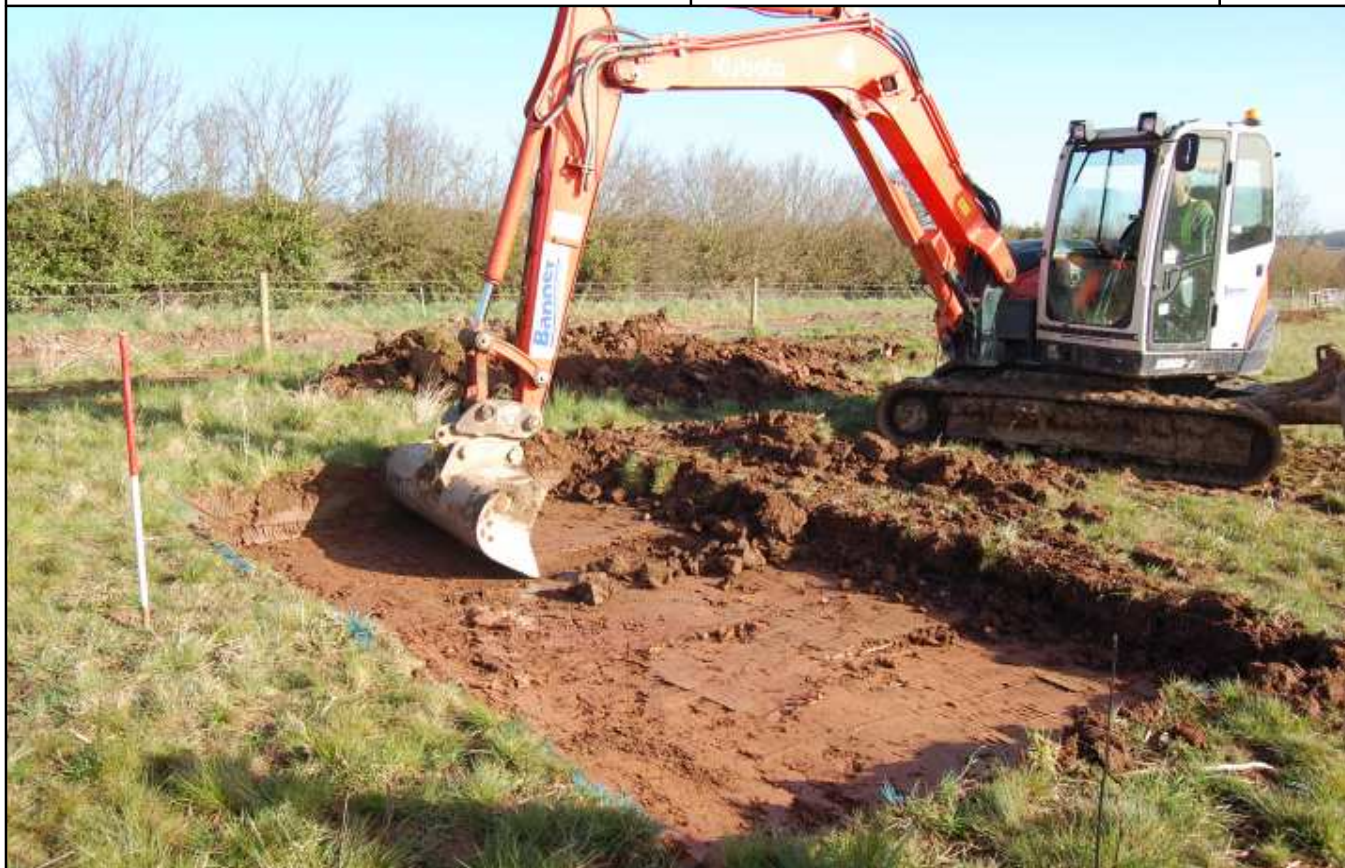
Plate 7: S trench for art installation during excavation, looking NW
