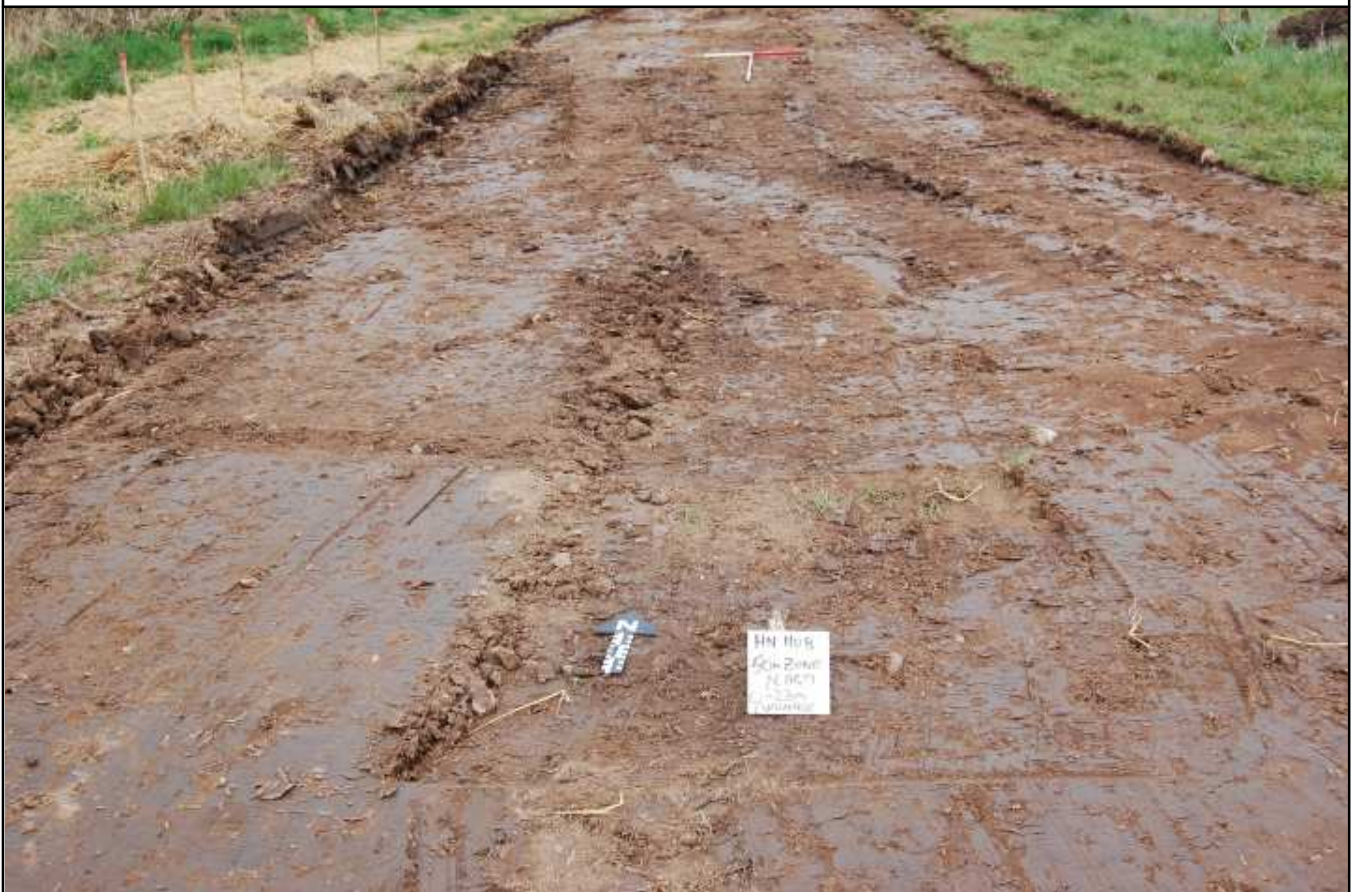
Plate 2: General shot of western arm, looking N
