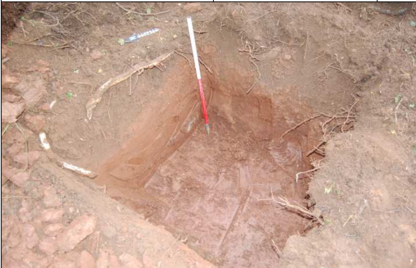
Plate 5: Soakaway trench, looking SE
