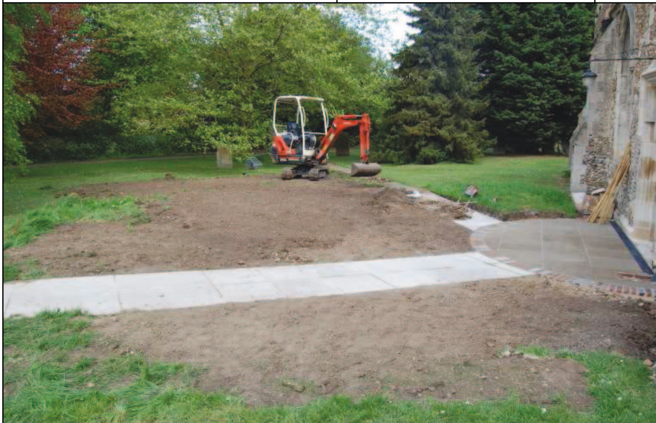
Plate 13: Grading of grassed area around entrance, looking east
