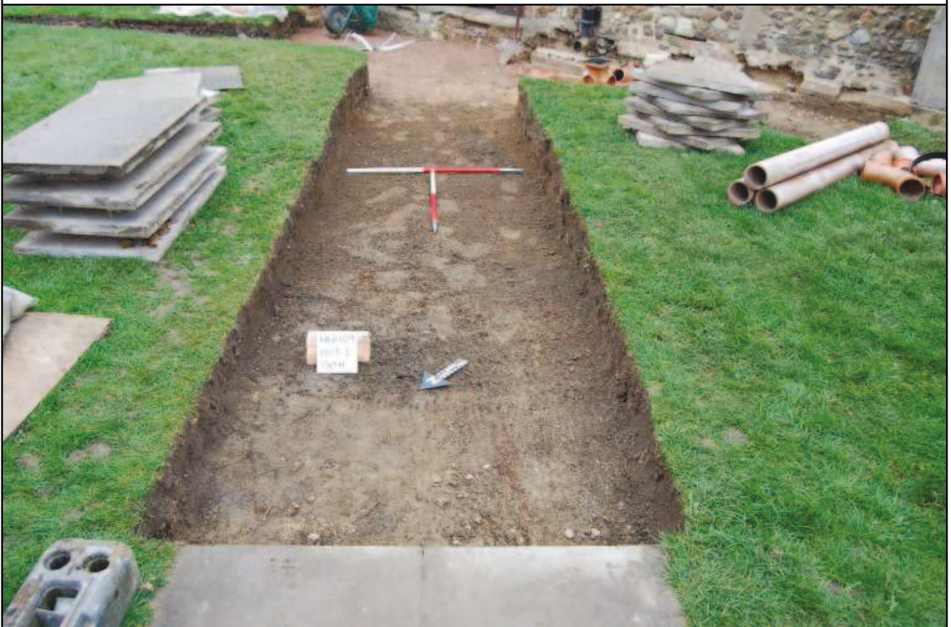
Plate 8: Western path, as reduced, looking south-east
