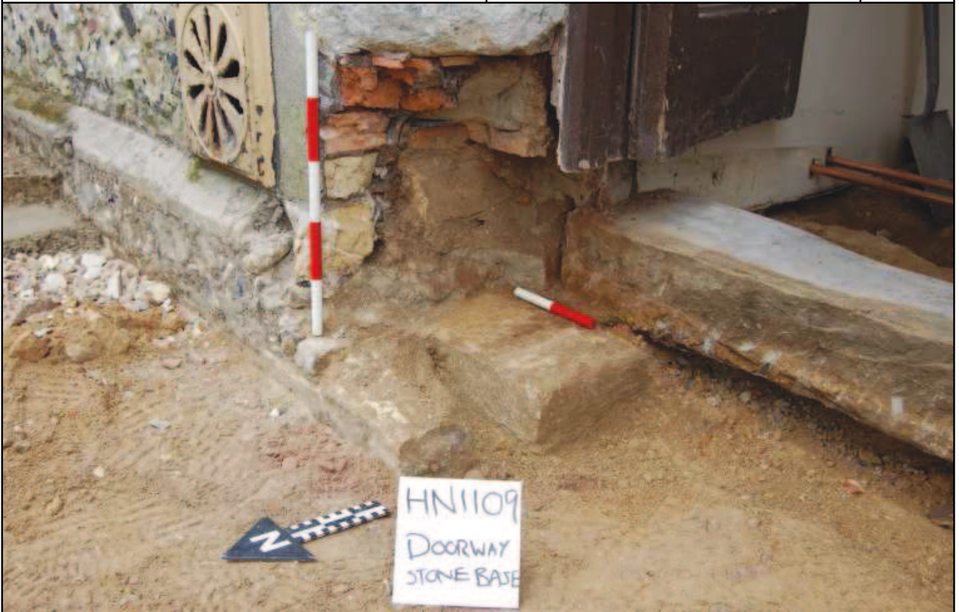
Plate 11: Exposed York stone block, looking south-east
