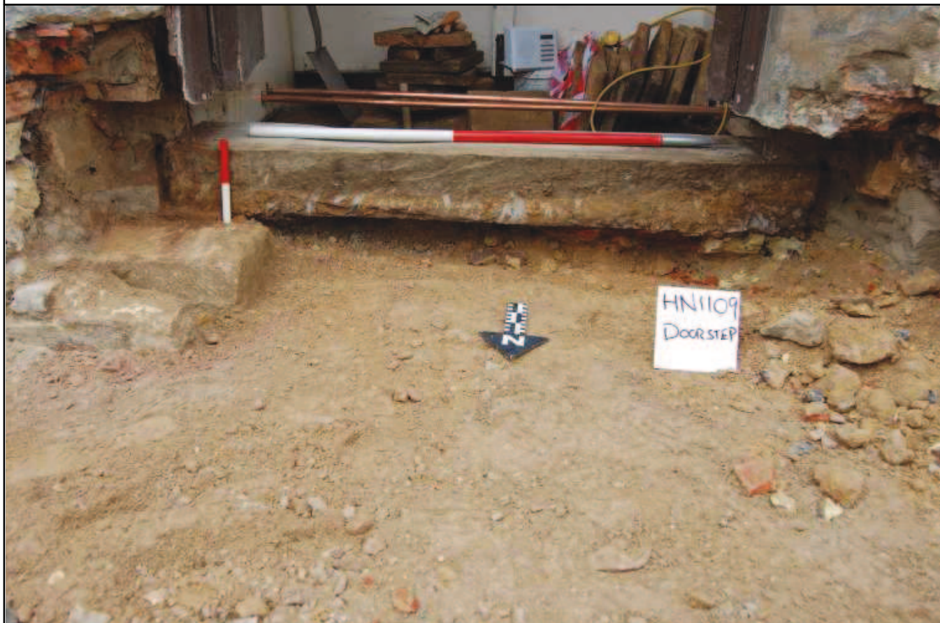
Plate 10: York stone step, showing underpinning material, looking south
