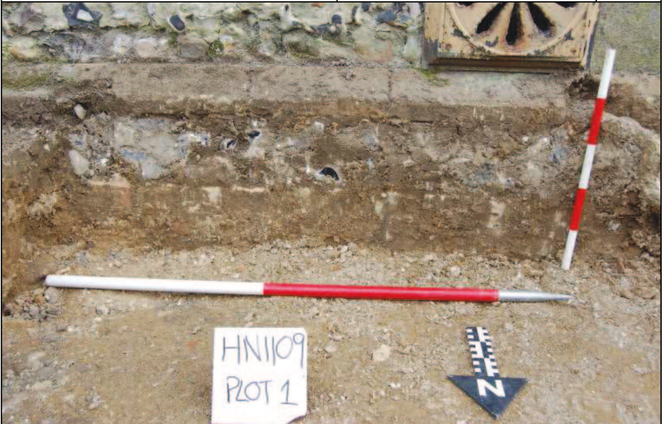
Plate 3: Exposed underpinning to north aisle wall, looking south
