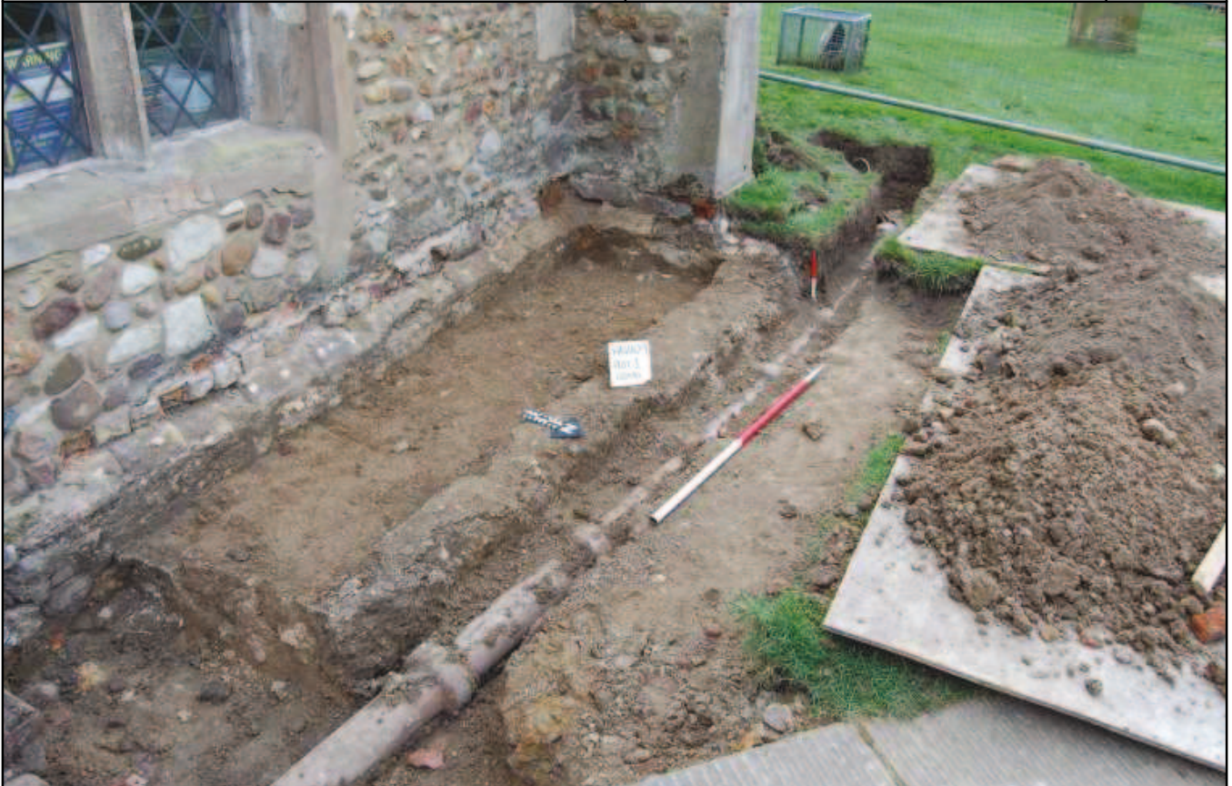
Plate 5: Lowering of existing drain, looking south-west
