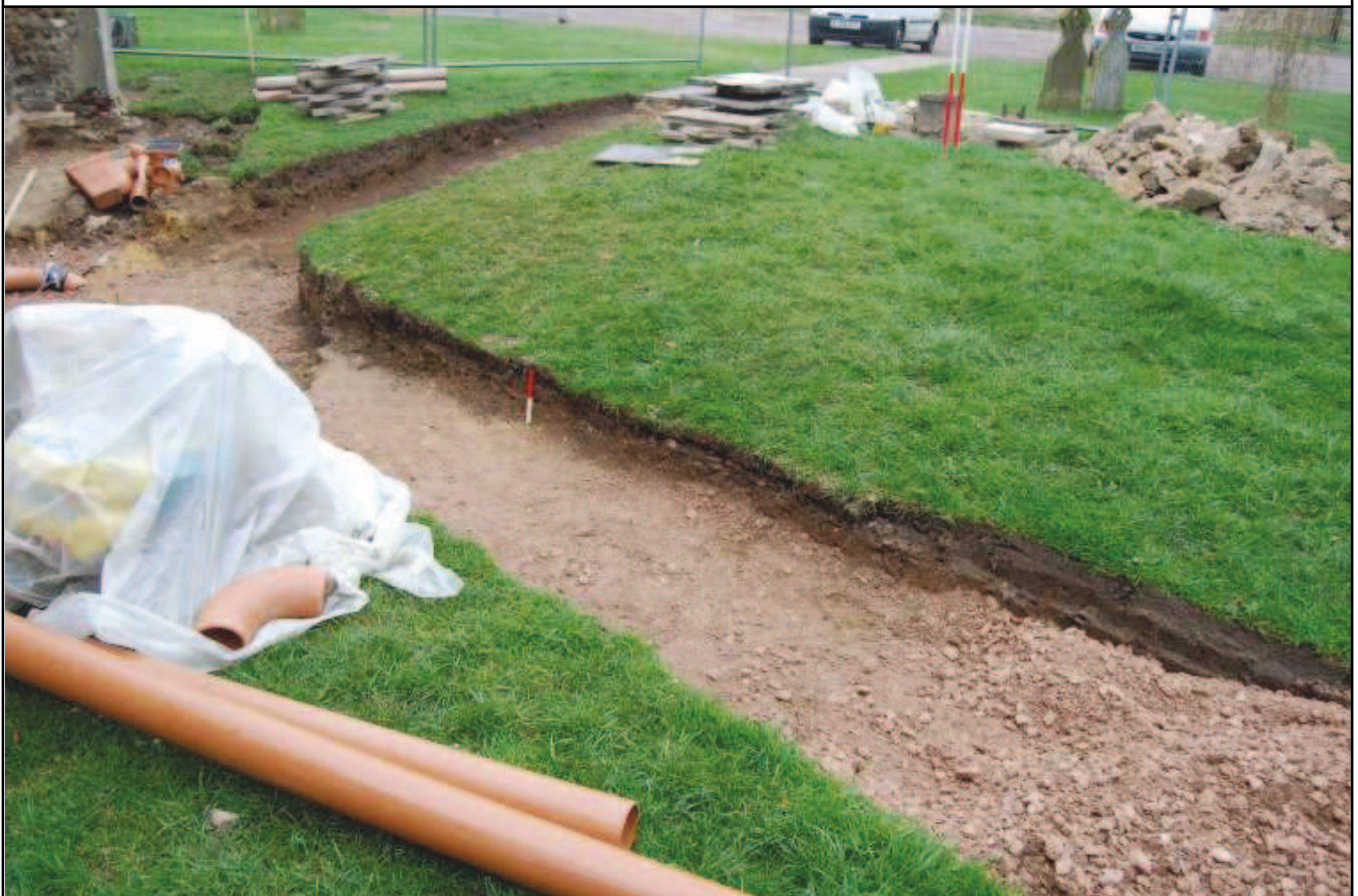
Plate 6: Footpath reduction, looking north-west
