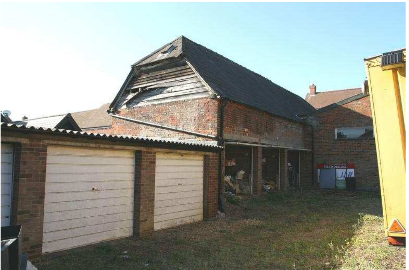
Plate 04 - NE elevation of barn (c) The Heritage Network Ltd.
