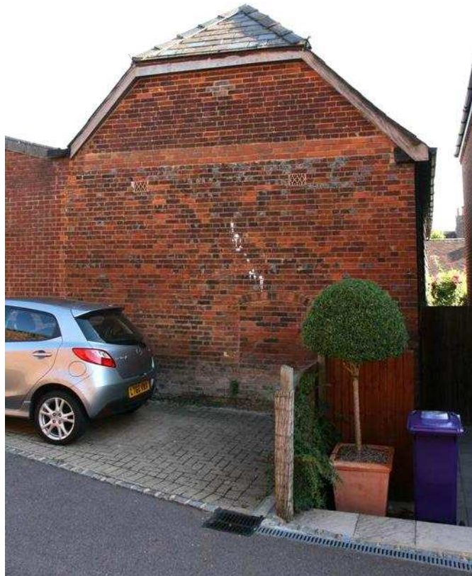
Plate 05 - SW elevation of barn
