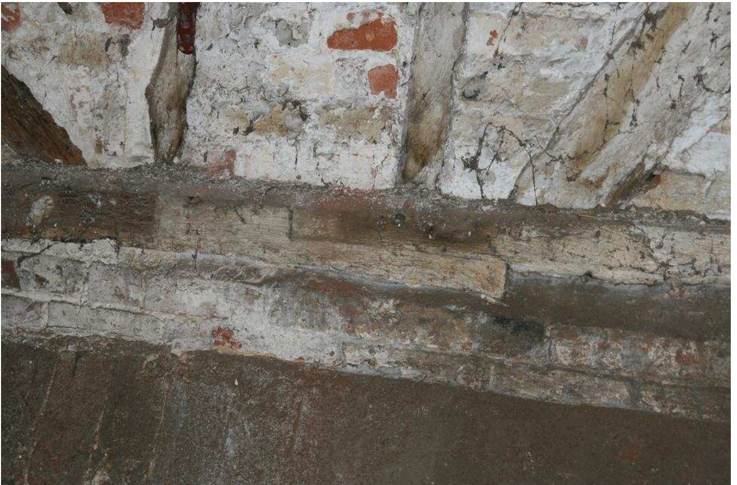
Plate 16 - Detail of scarf joint in sole plate, Bay 2 (c) The Heritage Network Ltd.
