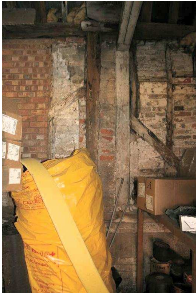
Plate 07 - Introduced post and tie-beam at S end of Bay 1
