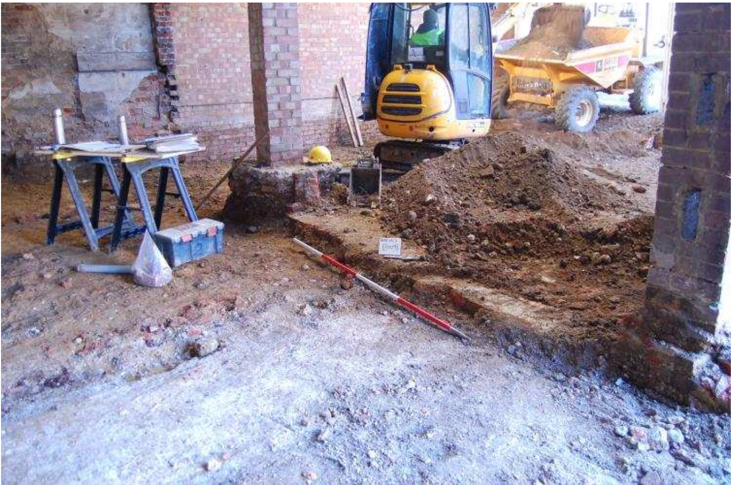
Plate 30 - Wall [1009], looking W (c) The Heritage Network Ltd.
