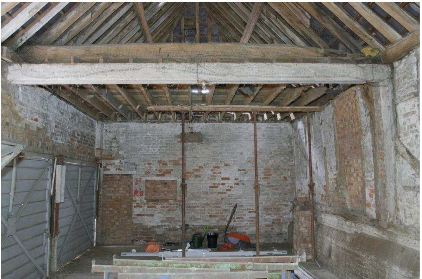
Plate 22 - NE interior elevation, looking NE (c) The Heritage Network Ltd.
