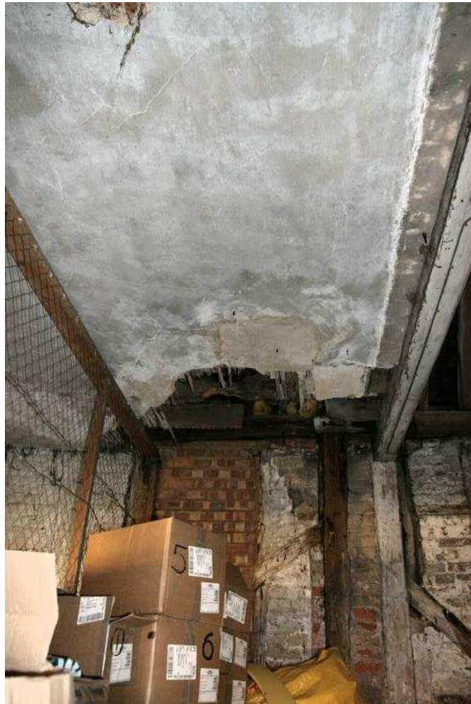
Plate 06 - Suspended ceiling in Bay 1 (c) The Heritage Network Ltd.
