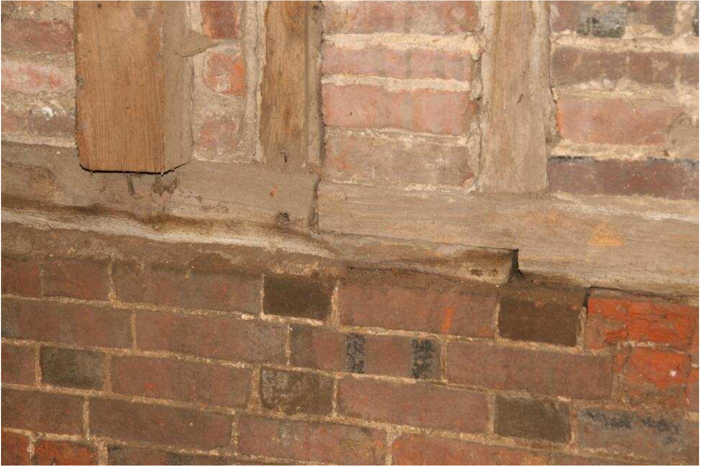
Plate 17 - Detail of scarf joint in sole plate, Bay 4
