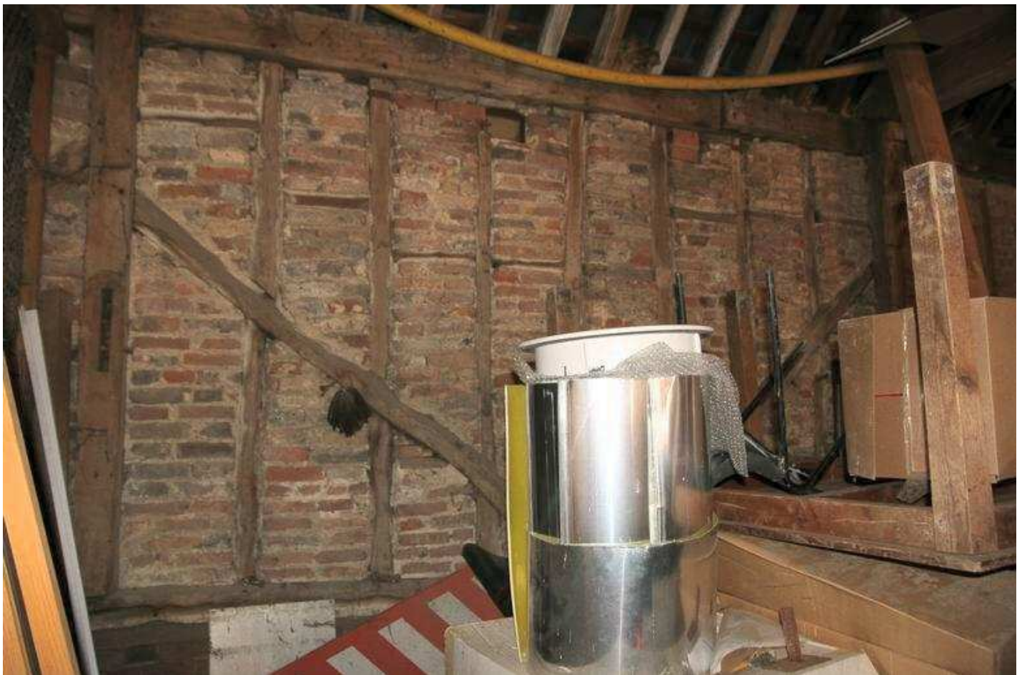
Plate 08 - Timber framing in SE elevation of Bay 3 (c) The Heritage Network Ltd.
