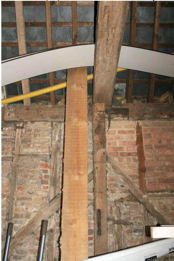
Plate 10 - Principal post and tie-beam between Bays 3 and 4 (c) The Heritage Network Ltd.
