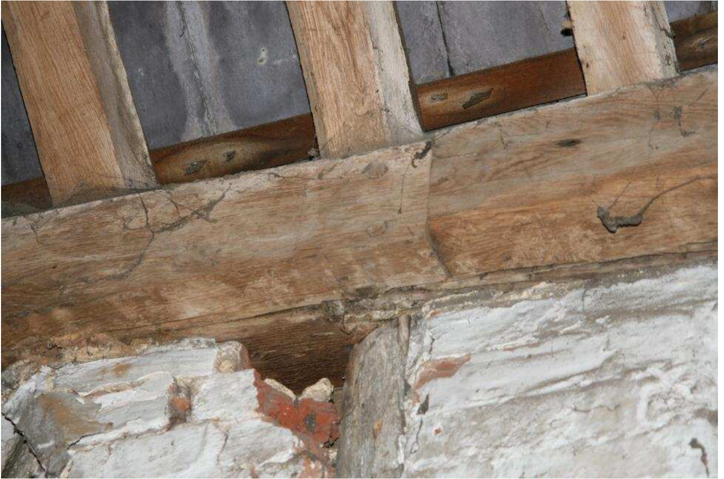
Plate 15 - Detail of joint in wall plate, Bay 3
