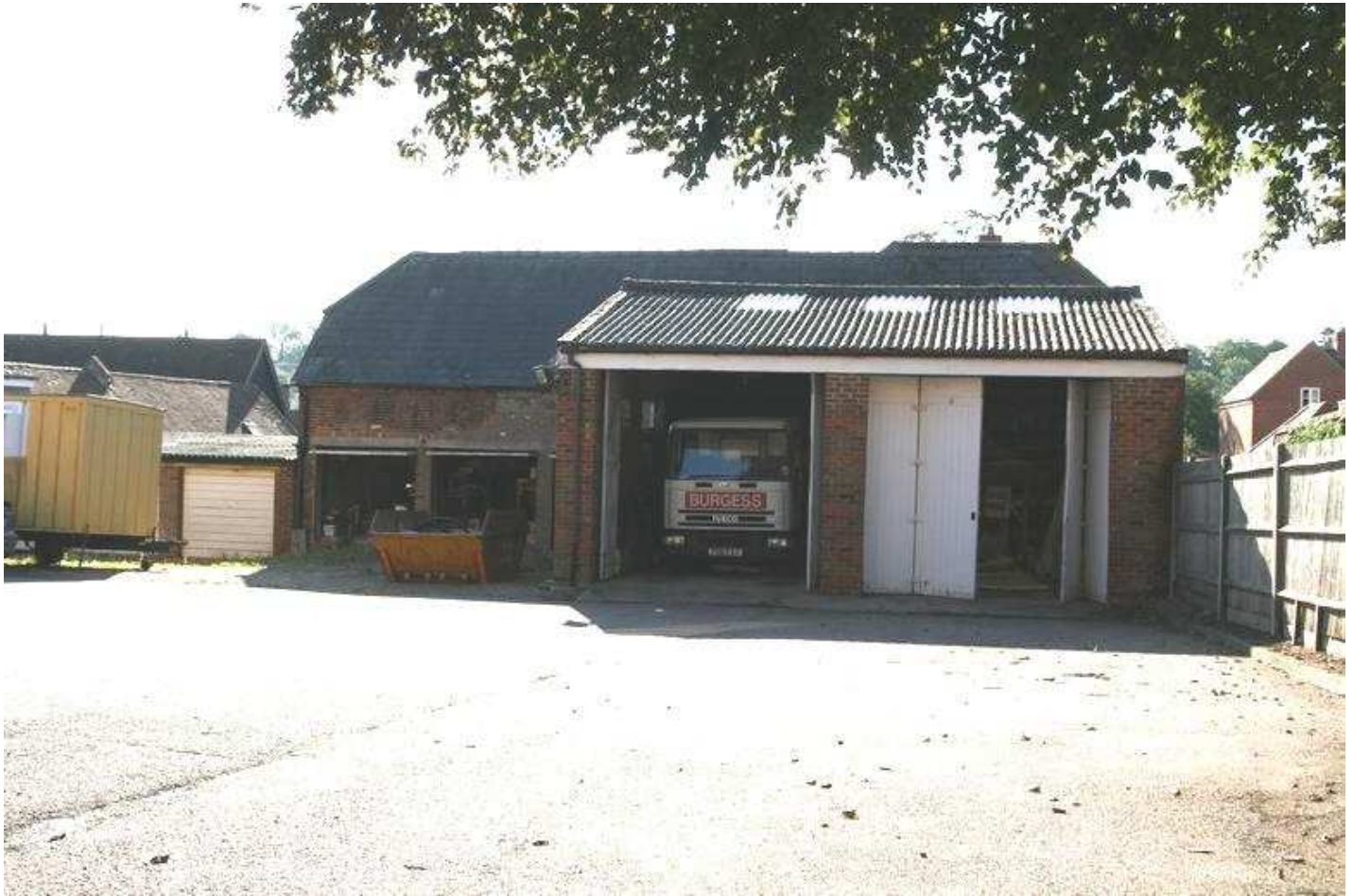
Plate 01 - Buildings along the SE boundary of the site
