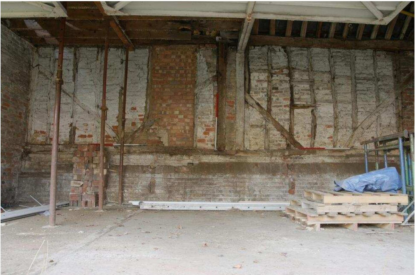
Plate 12 - Bays 1 & 2, SE elevation (c) The Heritage Network Ltd.
