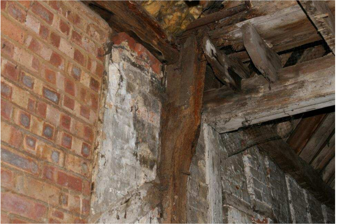
Plate 19 - Detail of the principal posts between Bays 1 & 2
