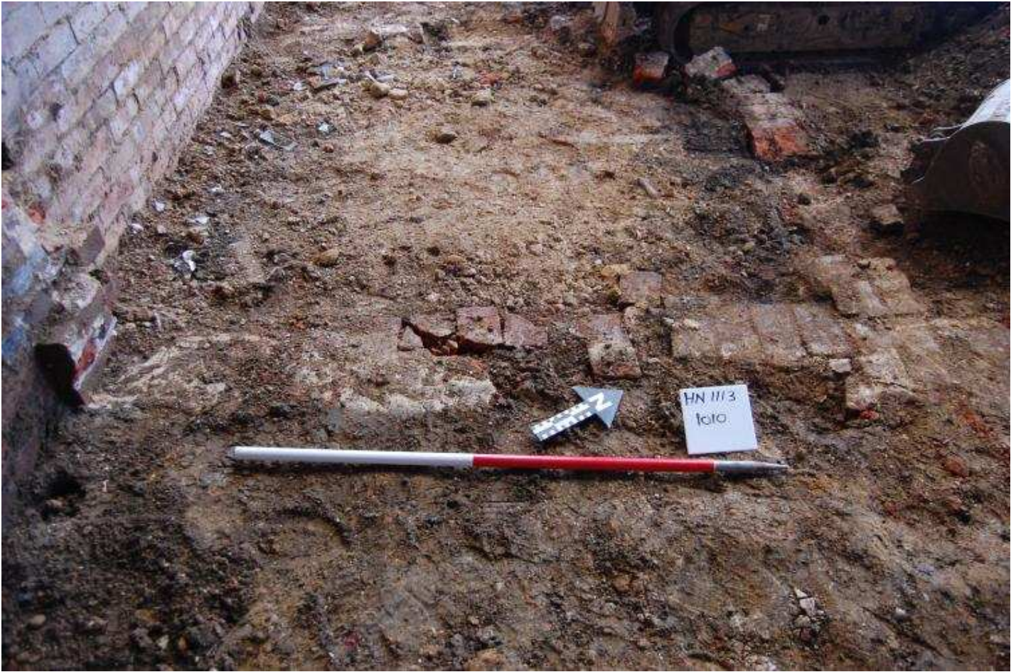
Plate 31 - Wall [1010], looking NW
