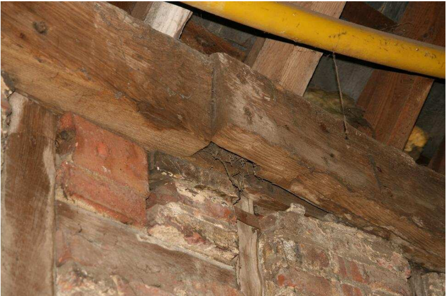
Plate 14 - Detail of scarf joint in wall plate, Bay 2 (c) The Heritage Network Ltd.
