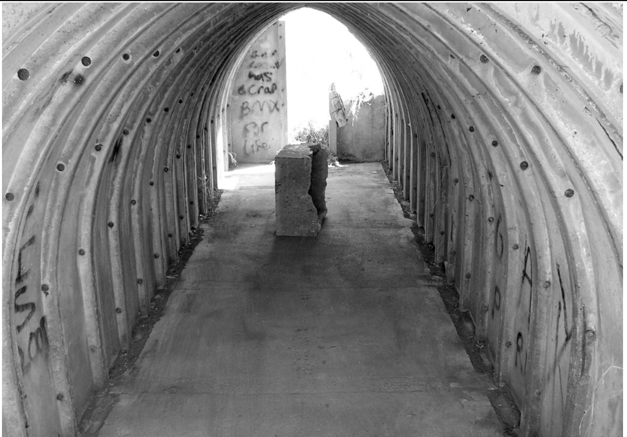
Plate 6: Area 6, Stanton air-raid shelter showing bolted panels and remains of removed escape hatch
