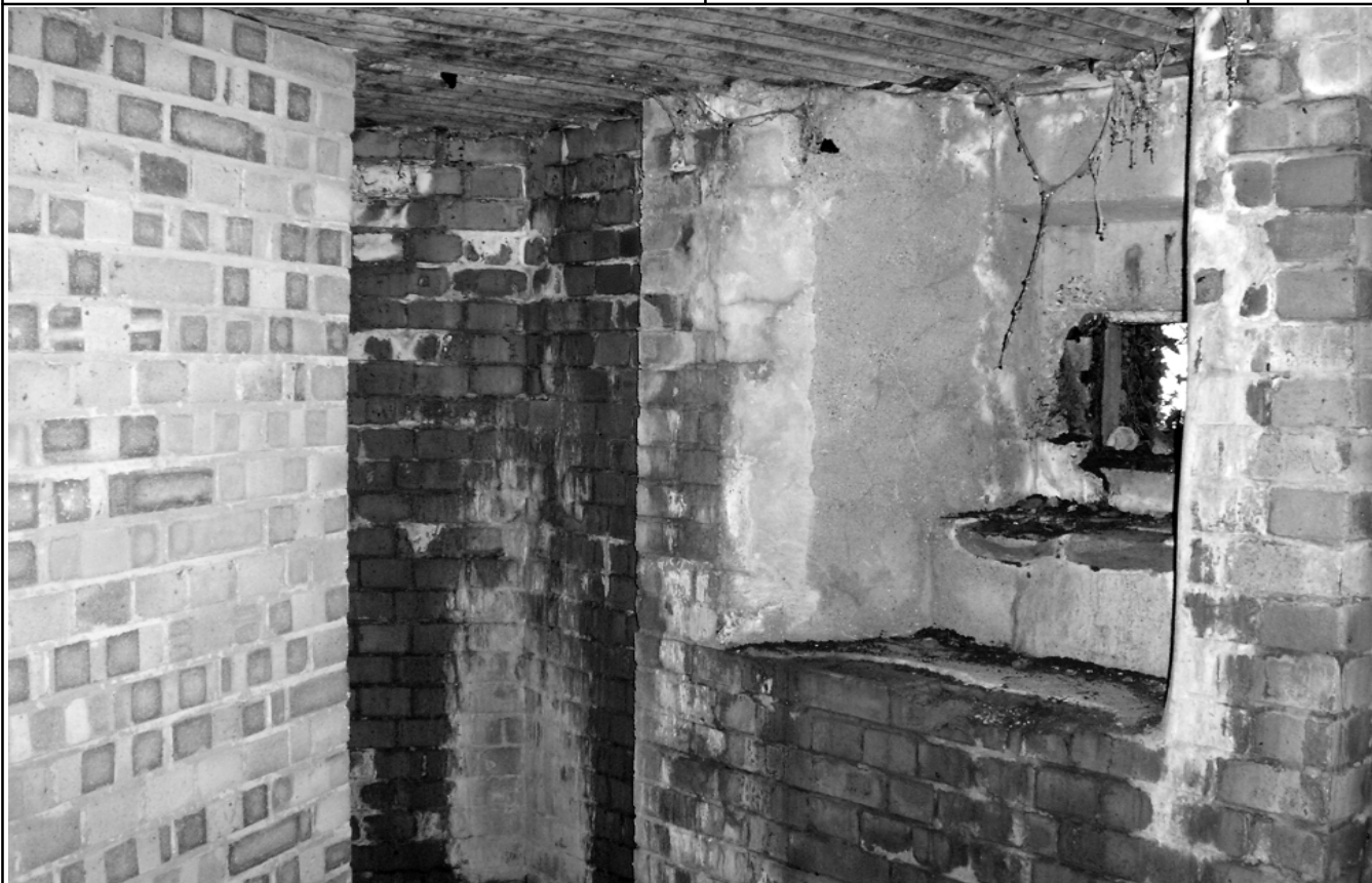
Plate 3: Area 3, Hunsdon-type hexagonal pill-box, Y shaped anti-ricochet partition and corrugated ceiling
