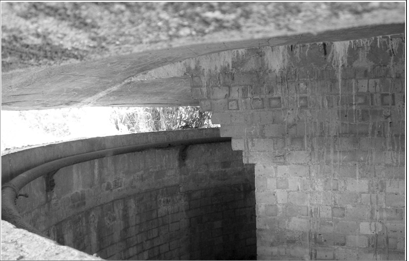
Plate 5: Area 5, cantilever pill-box interior showing metal rail
