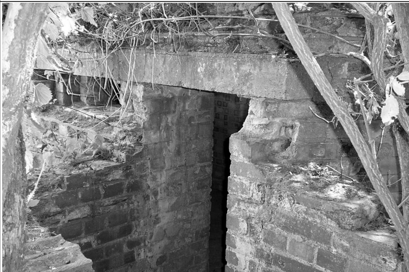
Plate 18: Area 12, Type-22 pill-box entrance
