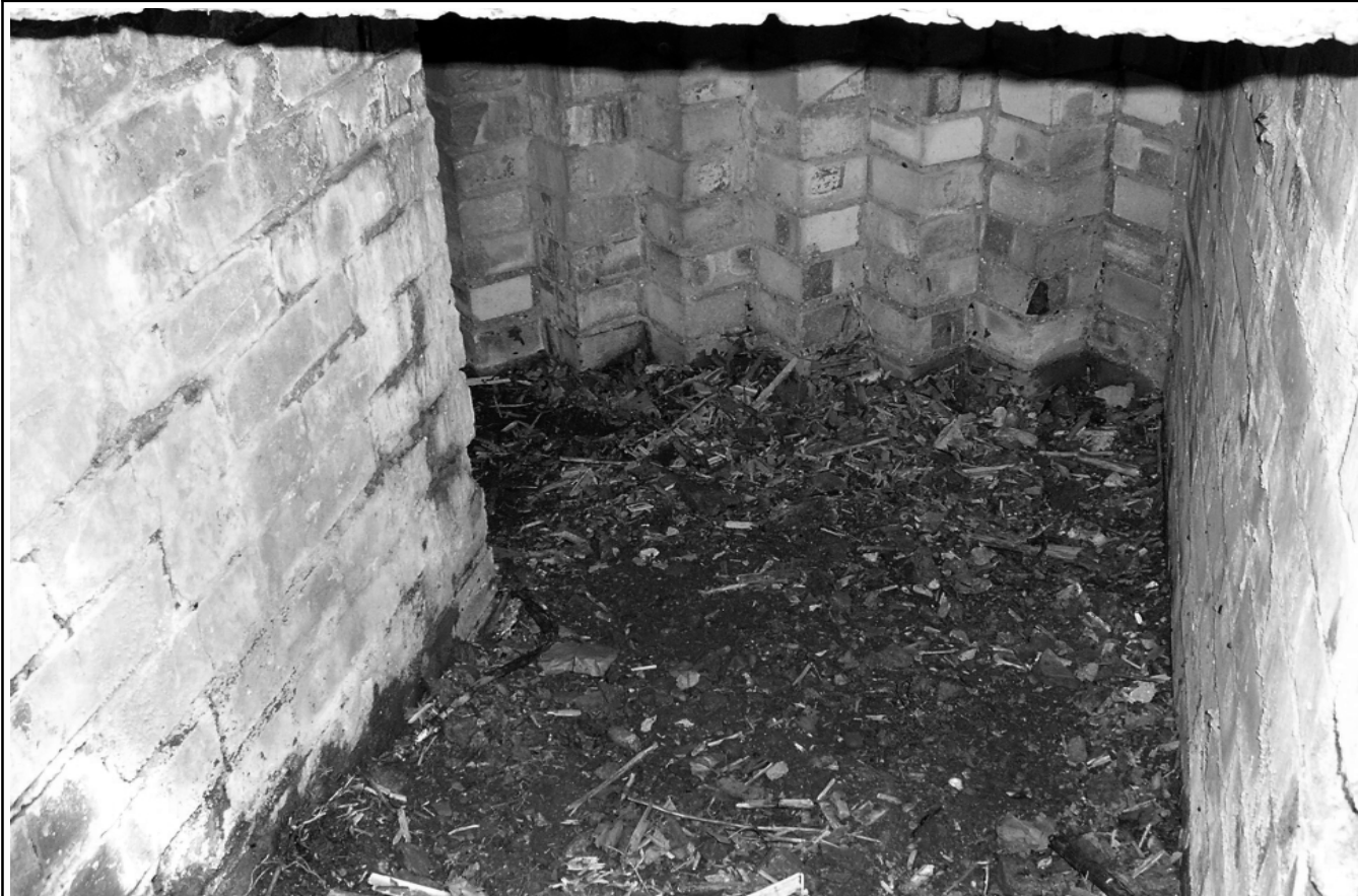
Plate 2: Area 3, Hunsdon-type hexagonal pill-box, entrance way and anti-ricochet wall
