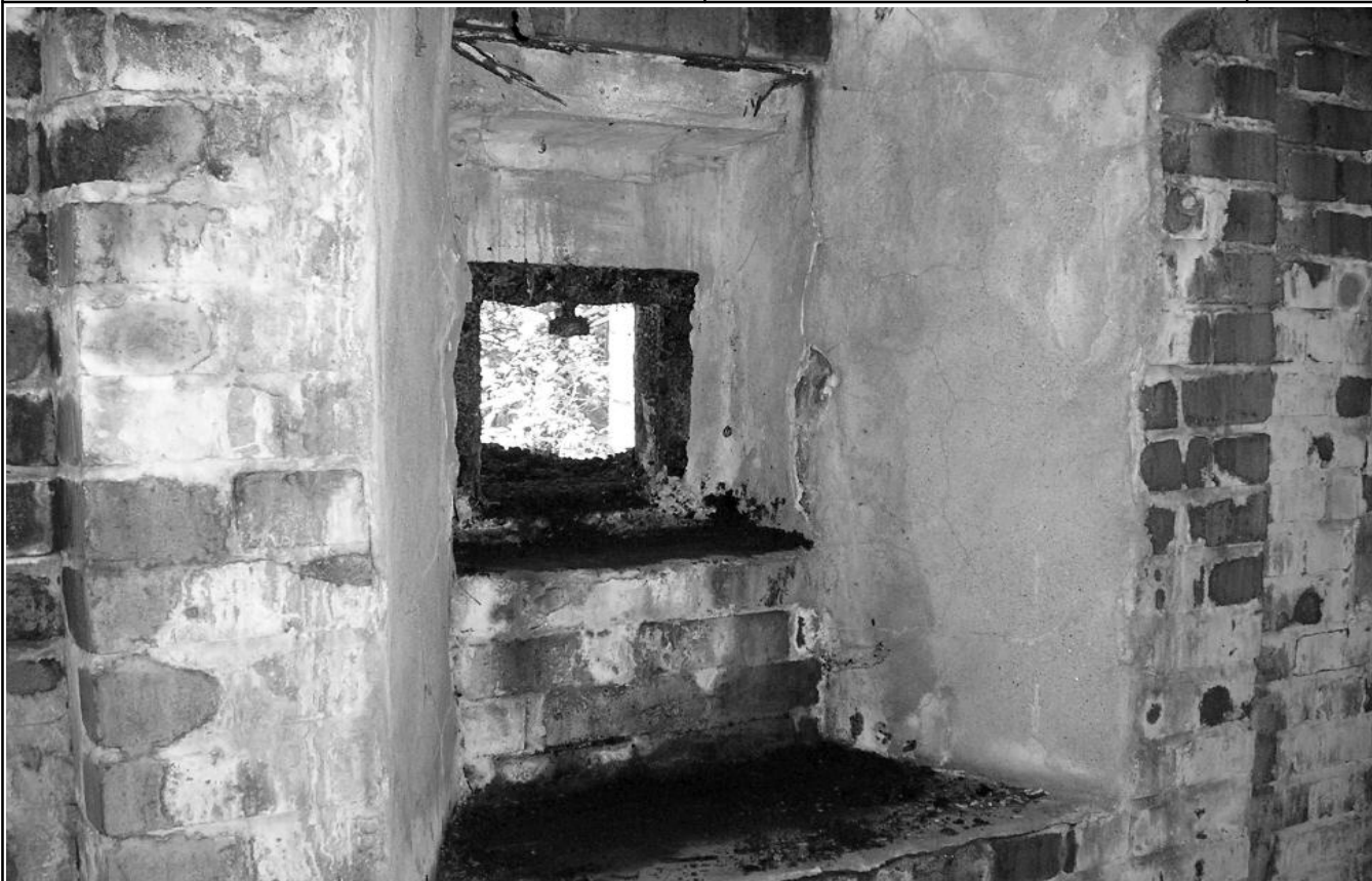
Plate 7: Area 8, Hunsdon-type pill-box interior showing remains of machine gun mounting pivot at top of aperture.
