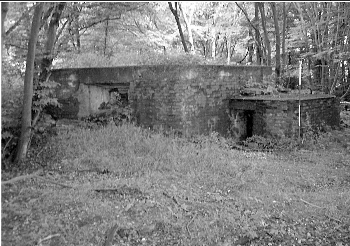
Plate 11: Area 9, Hunsdon-type pill-box, looking north
