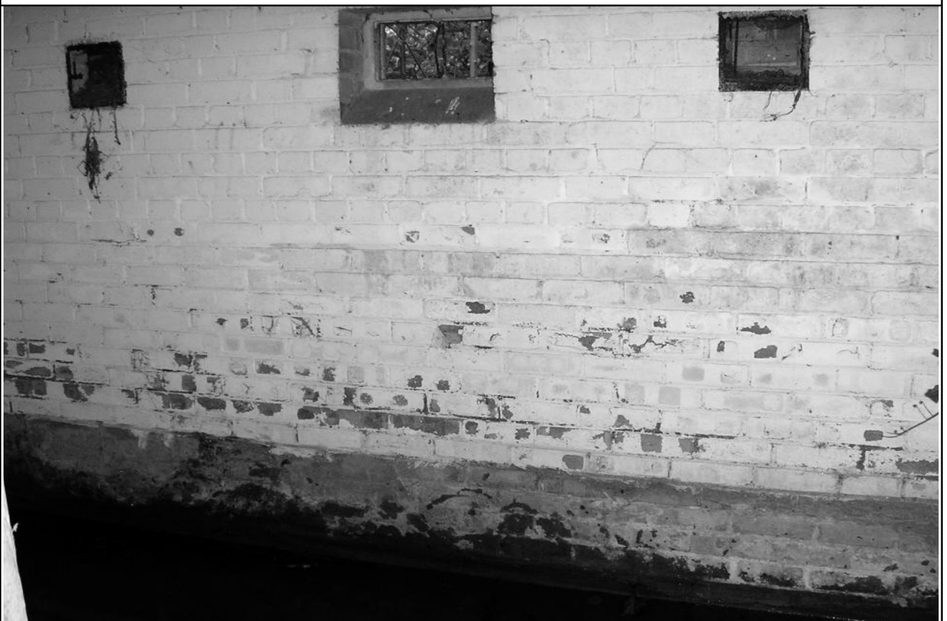
Plate 10: Area 8, ammunition store, northern interior elevation showing window openings
