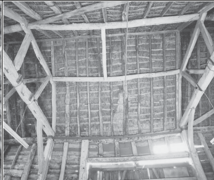
Frame 8: Mid bay, western roof structure
