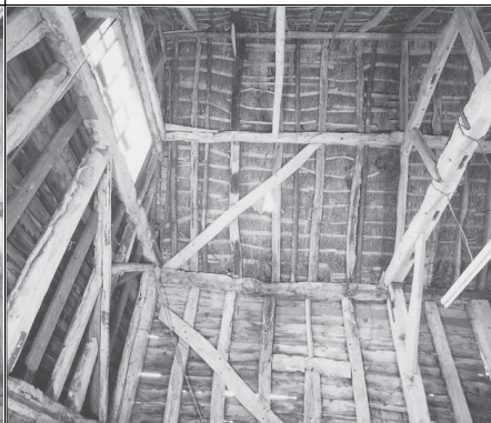
Frame 11: S bay, western roof structure
