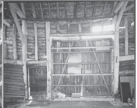
Frame 9: Mid bay, W interior elevation
