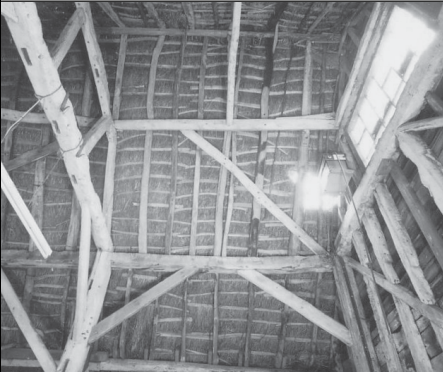
Frame 3/1: S bay, eastern roof structure
