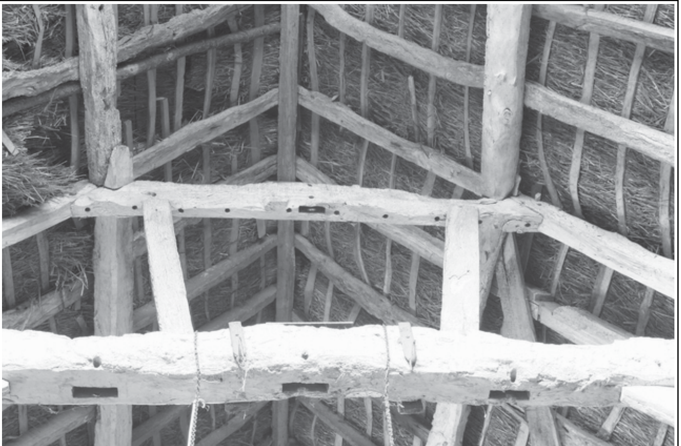
Plate 6: Tie-beam and collar, southern bay, northern frame
