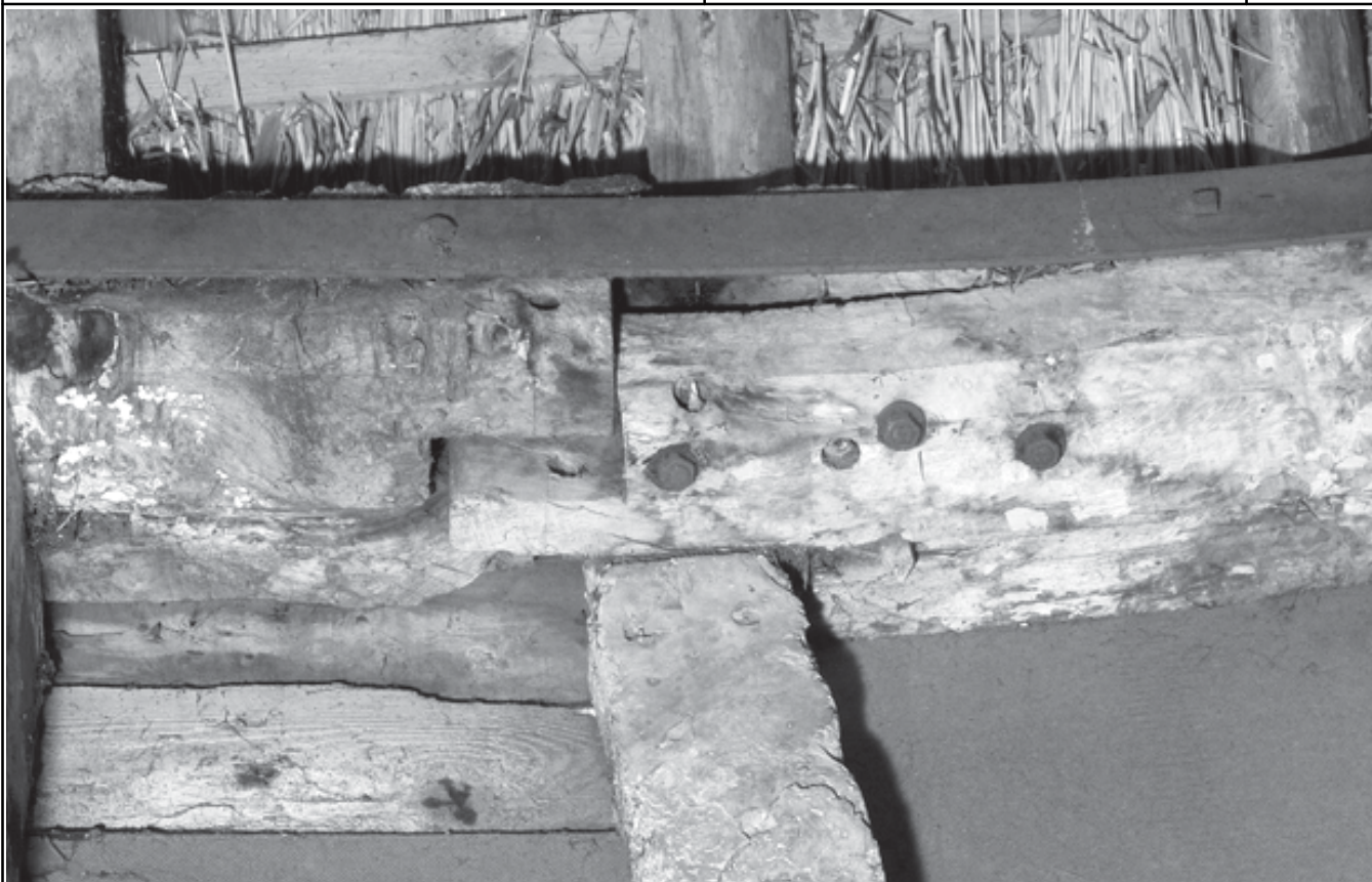
Plate 7: Edge-halved scarf joint in western wall plate
