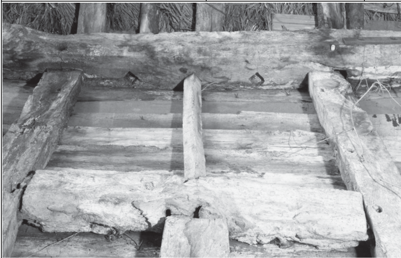
Plate 9: Window opening in southern bay
