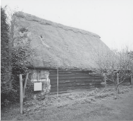
Frame 1: Eastern exterior elevation
