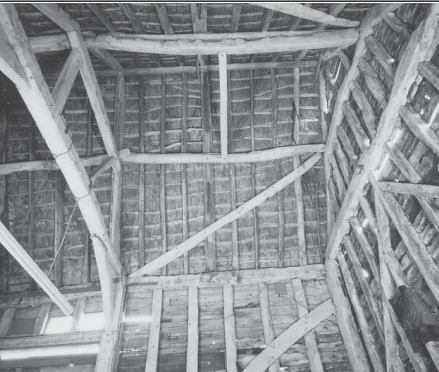
Frame 7: N bay, western roof structure
