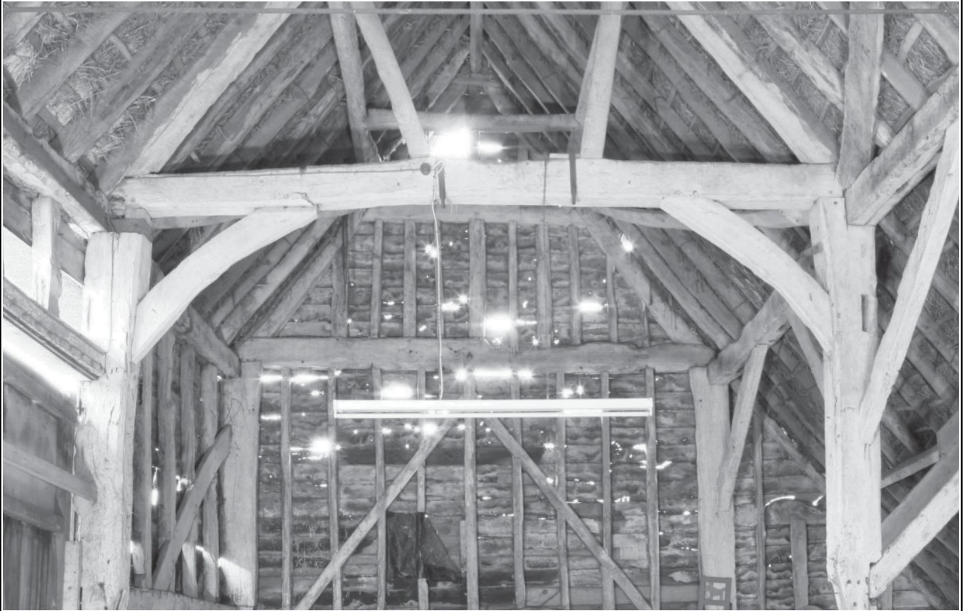
Plate 5: Framing, northern bay, looking N
