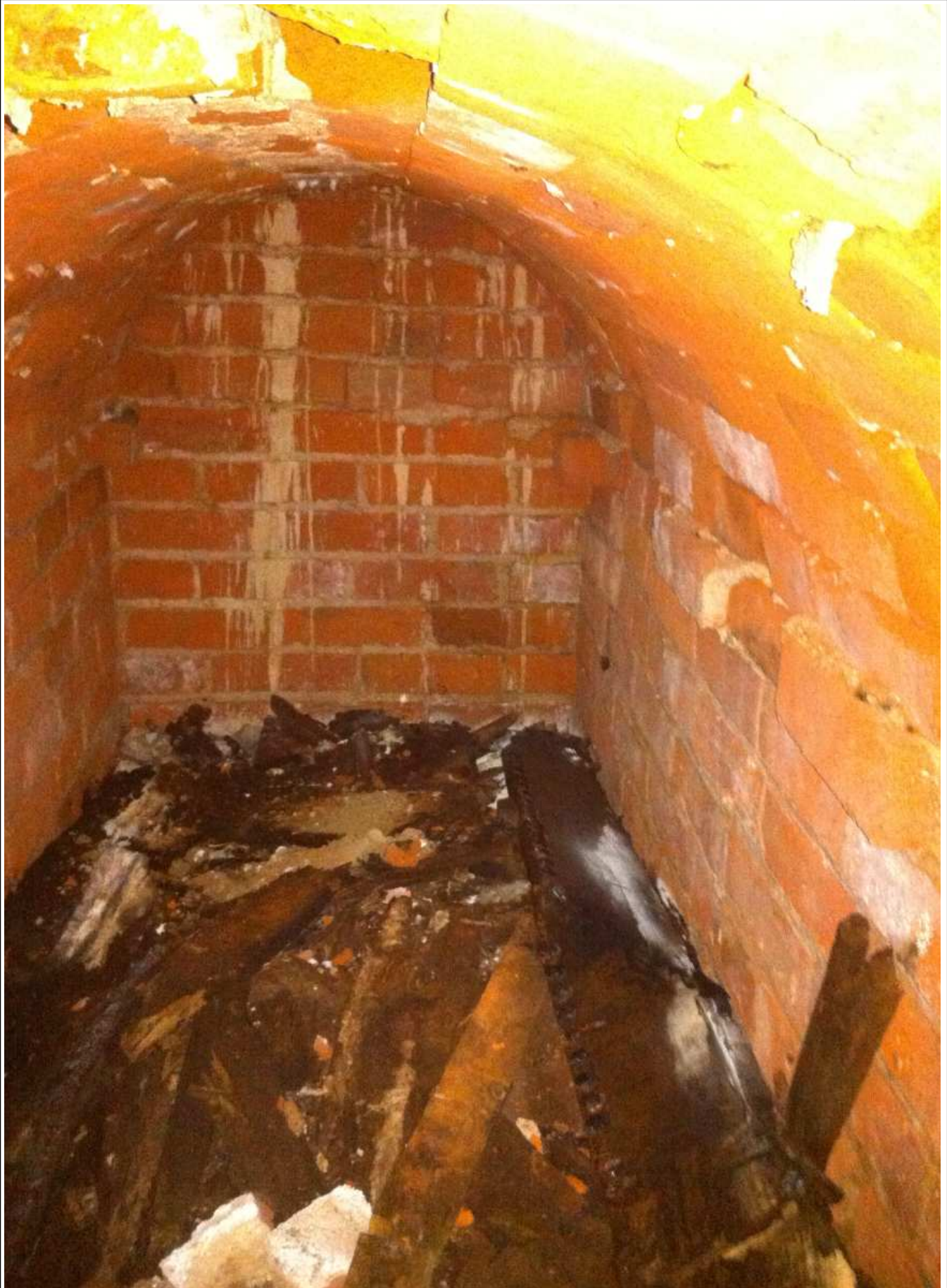
Plate 9: Vault beneath the chancel, looking east. Photograph supplied by contractors.
