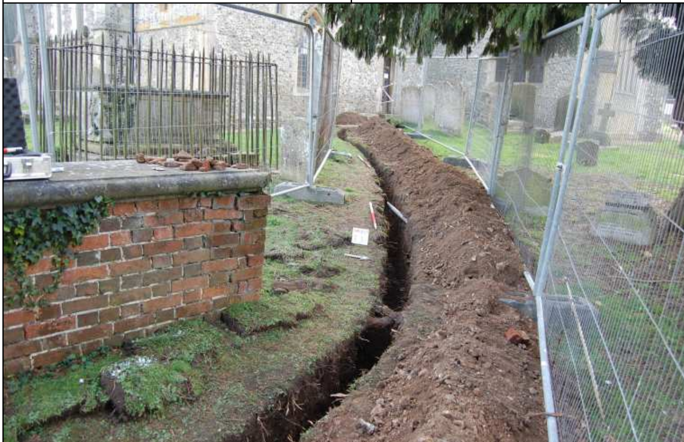
Plate 5: West section of trench, looking south-west
