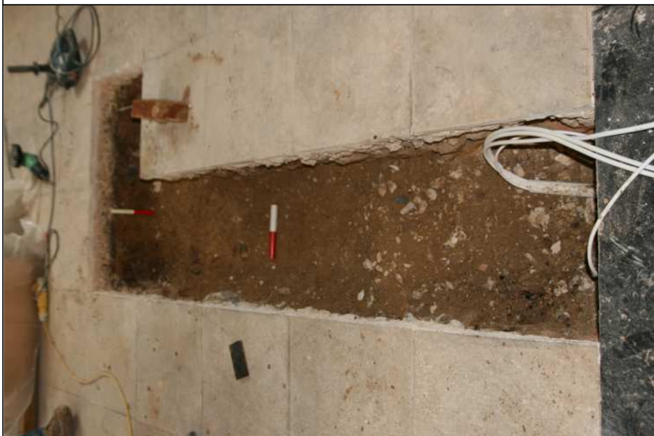
Plate 6: South-eastern internal trench, looking east
