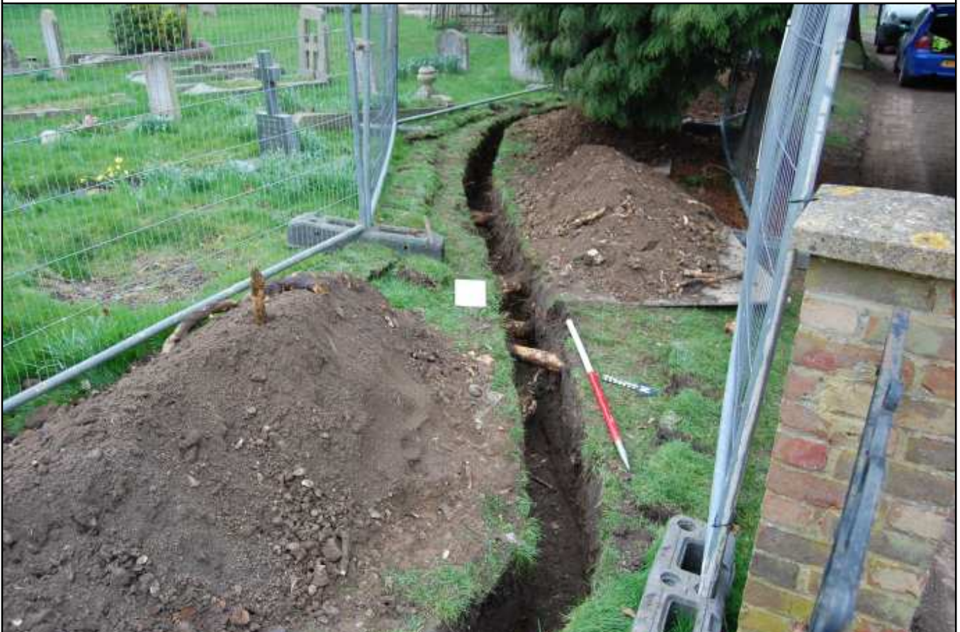
Plate 4: Middle Section of trench, looking southwest
