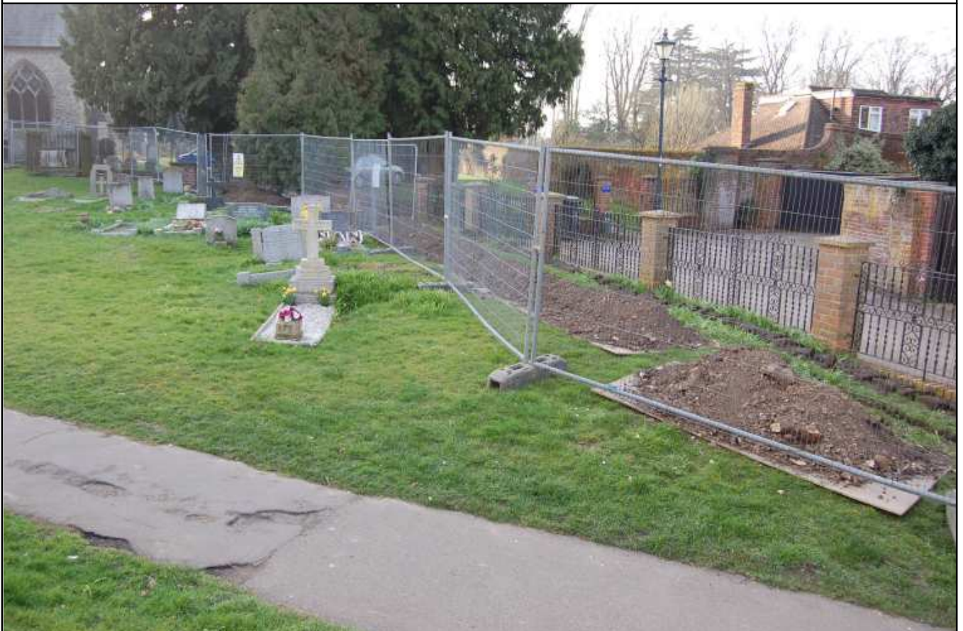
Plate 2: Area of work for gas main, looking west
