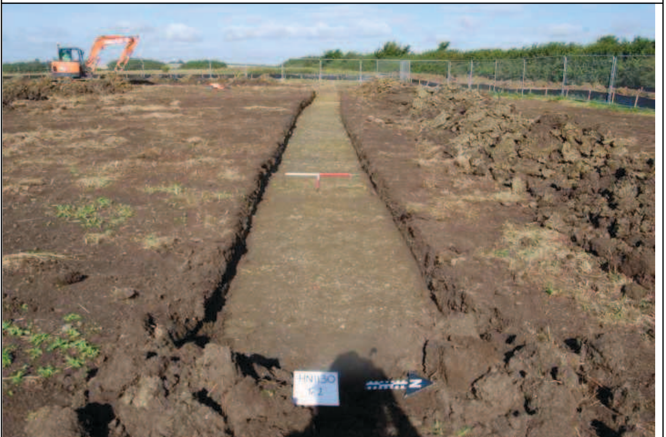
Plate 2: Trench 2, looking W
