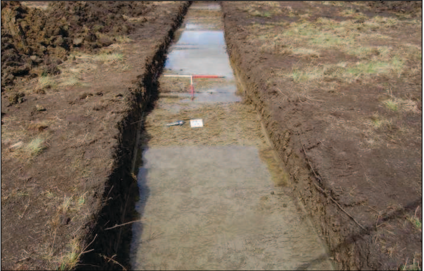
Plate 15: Trench 9, looking W
