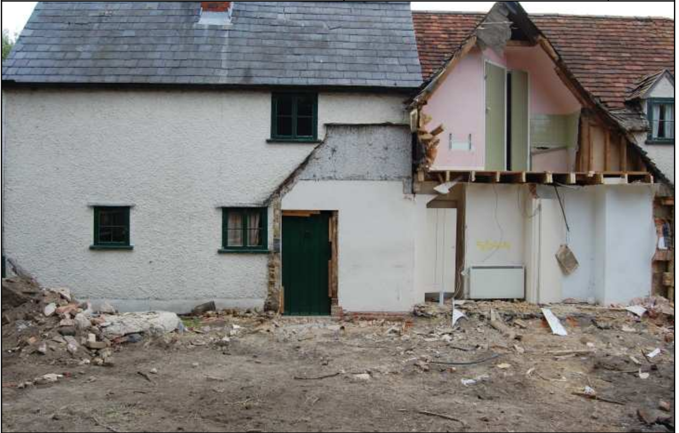
Plate 1: North end of W elevation, looking E
