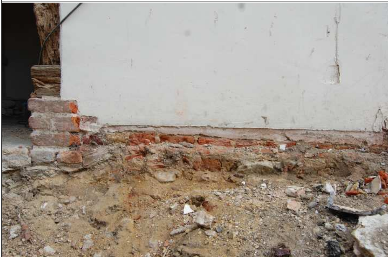
Plate 4: Brick plinth below W elevation
