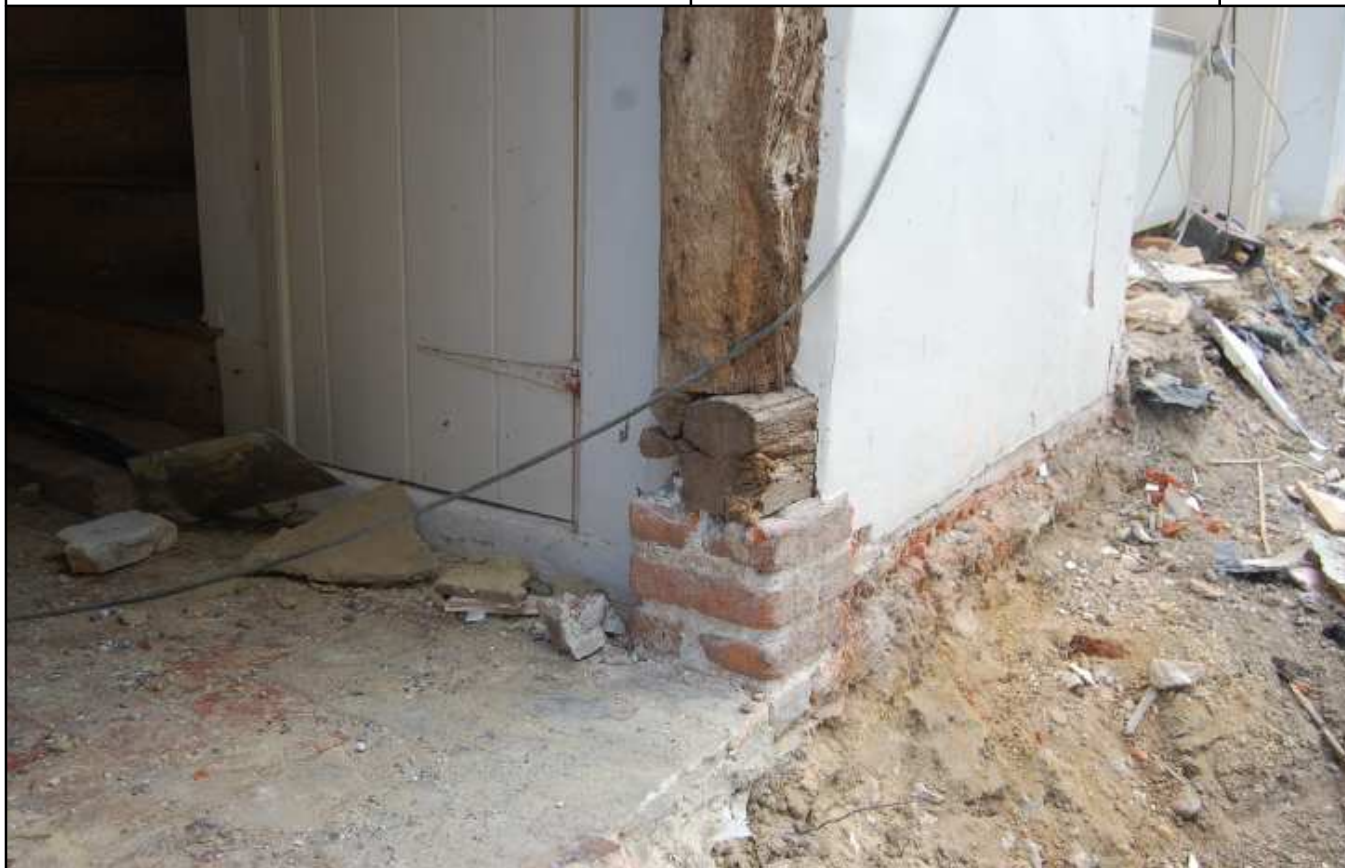
Plate 3: Post and cut wall plate, doorway at S end of northern block
