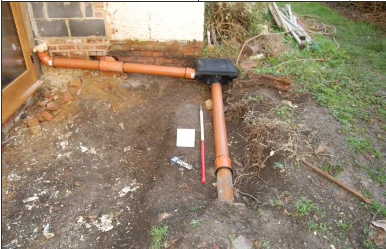
Plate 9: Trench 1, looking W
