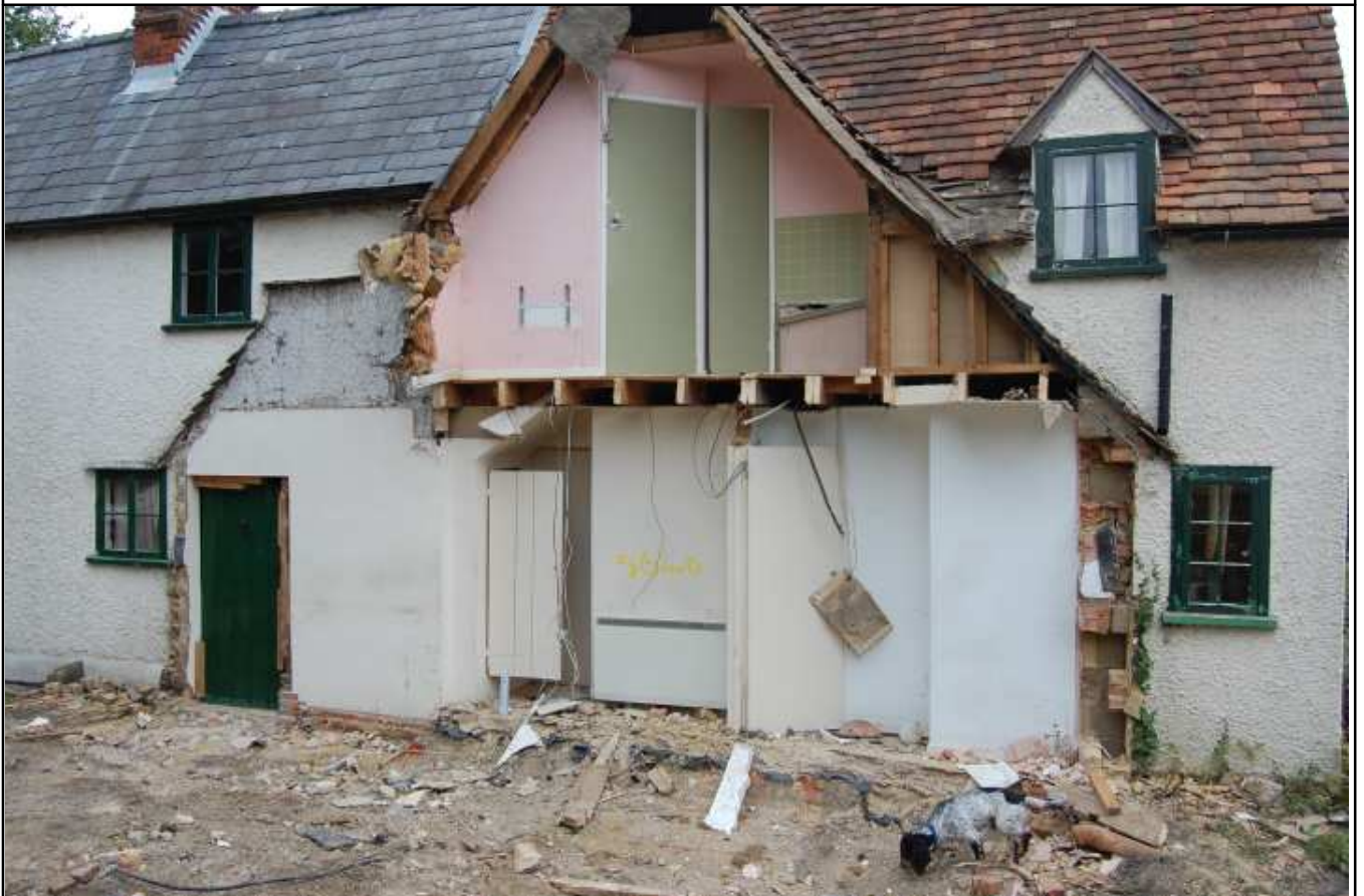
Plate 2: South end of W elevation, looking SE
