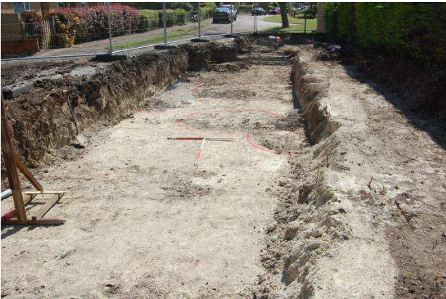
Plate 05 - Area 4, looking SE
