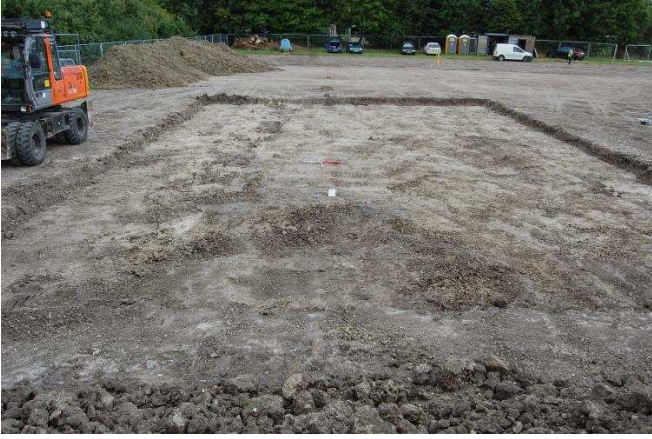
Plate 01 - Area 1, looking N
