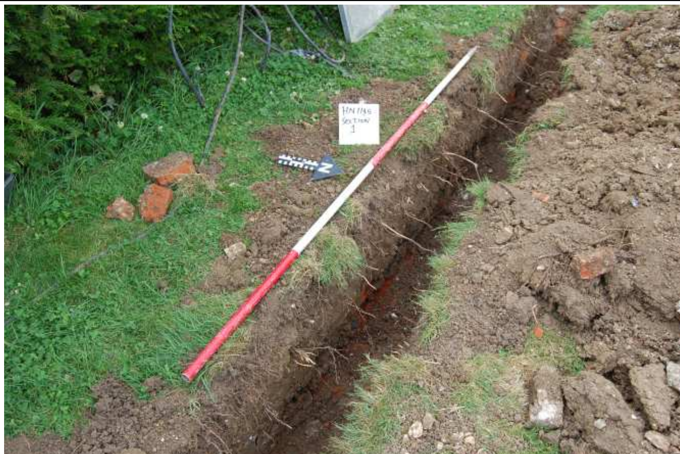
Plate 4: Service trench, looking SE
