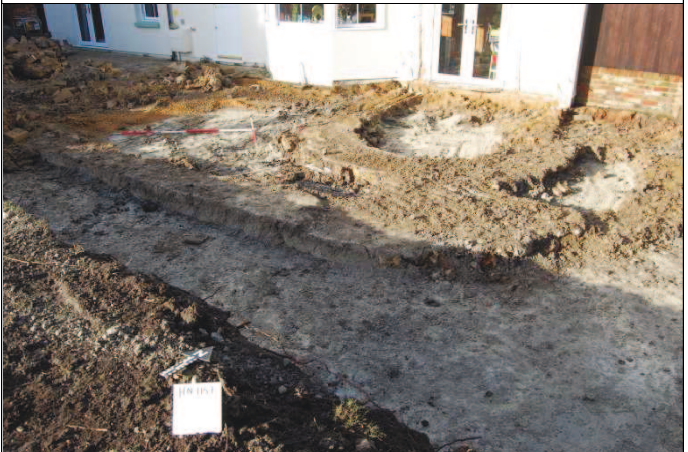
Plate 2: Area of ground reduction, looking SW
