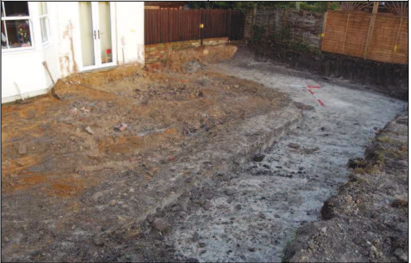
Plate 1: Area of ground reduction, looking NW
