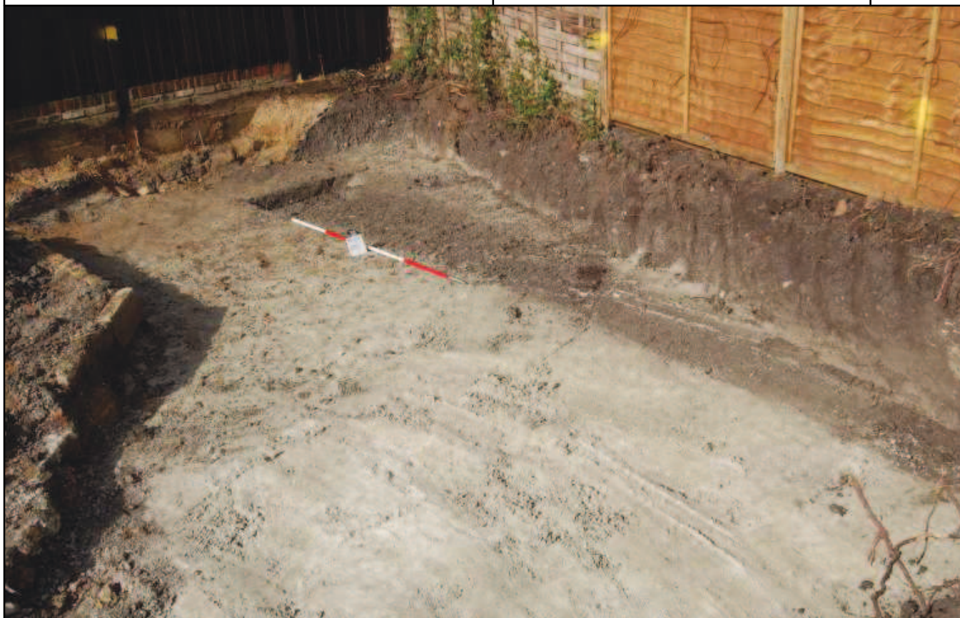
Plate 3: Ditch [101] looking NW
