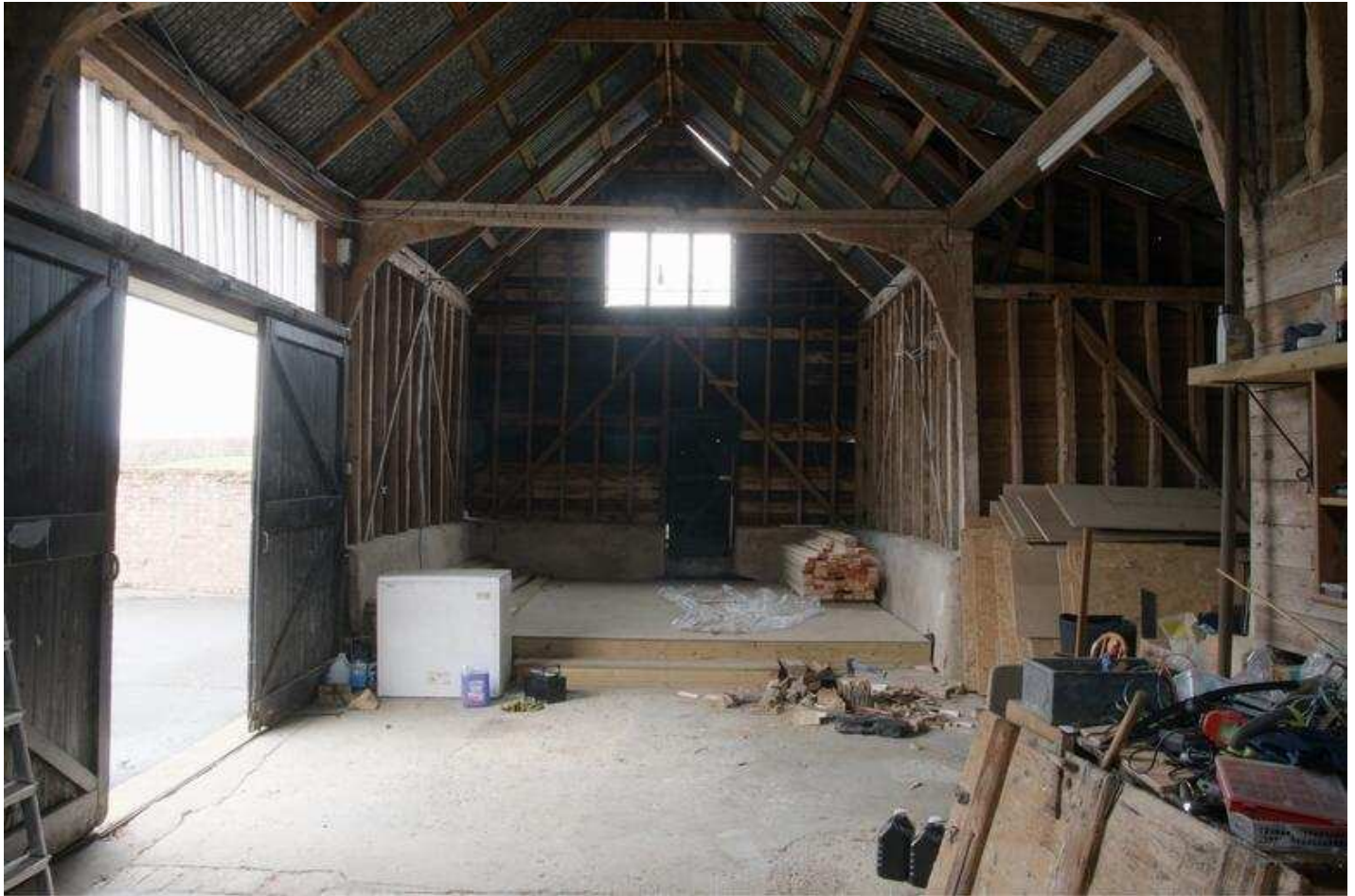
Plate 07 - SW gable end
