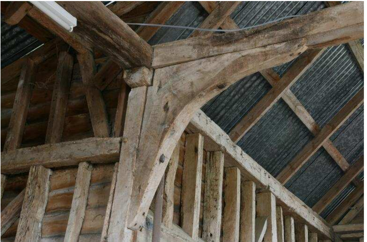
Plate 10 - Bay 2 & 3, detail of brace, NE side
