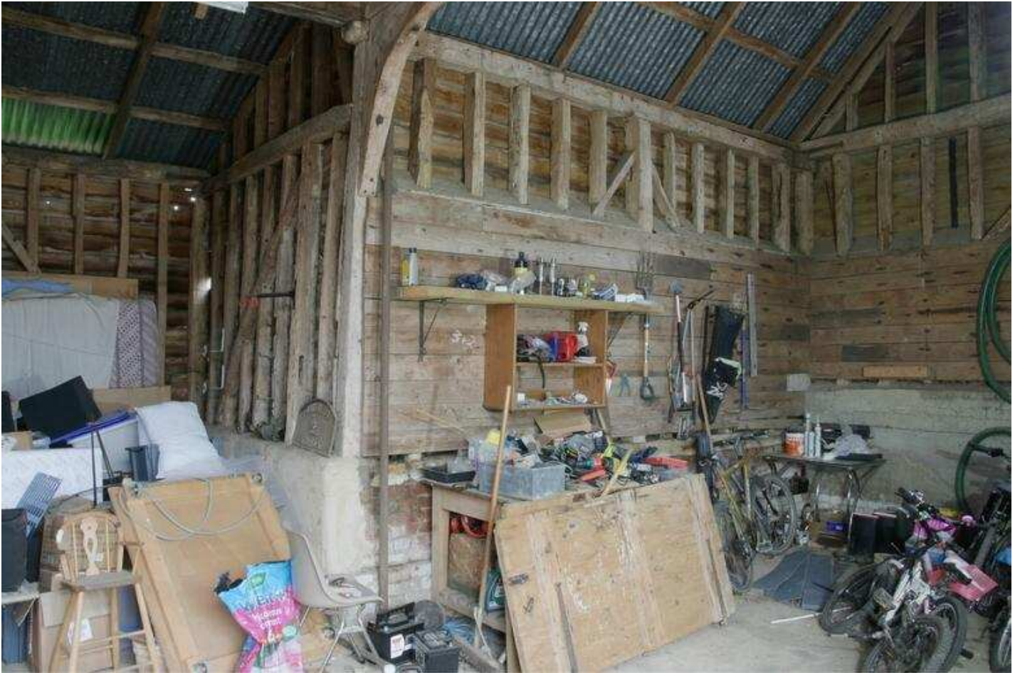
Plate 05 - NW & NE elevations, Bay 3
