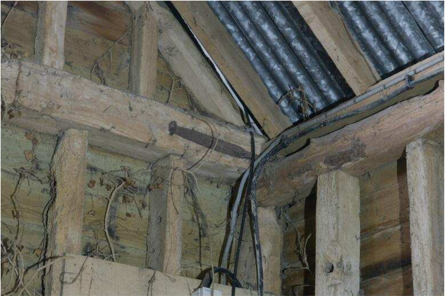
Plate 09 - Bay 1, iron brace in SE corner
