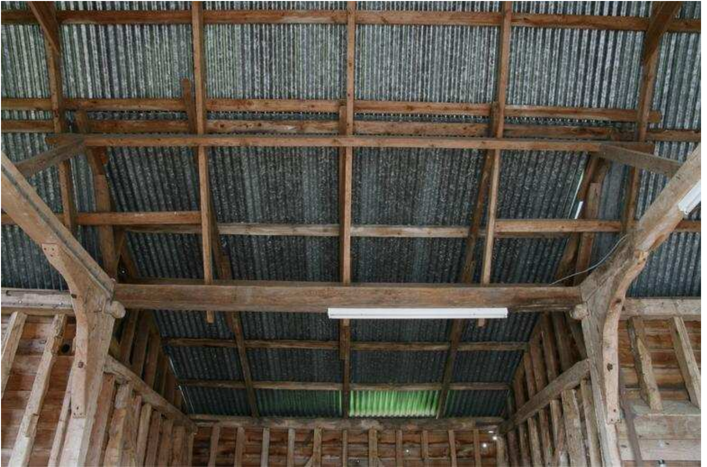
Plate 17 - replaced wall plate across opening to midstrey
