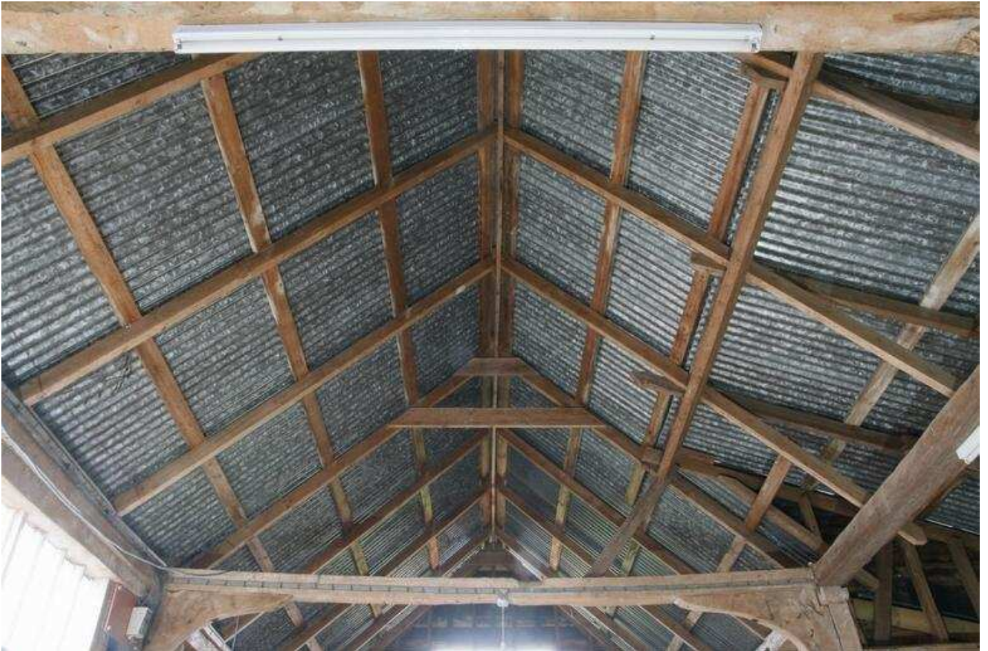
Plate 20 - roof structure, looking NW
