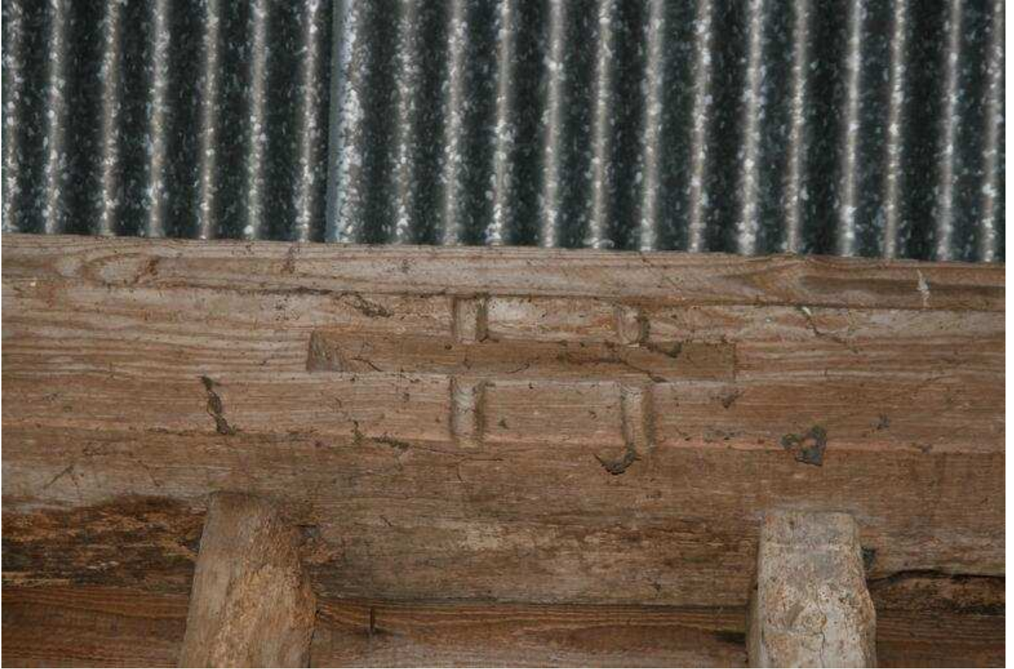
Plate 19 - Bay 3, NW elevation, detail of reused wallplate
