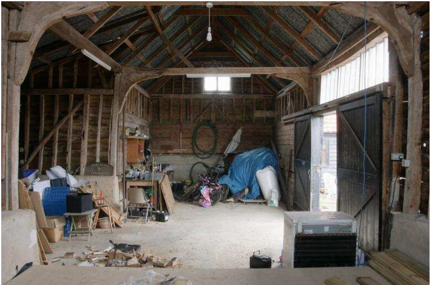
Plate 08 - NE gable end
