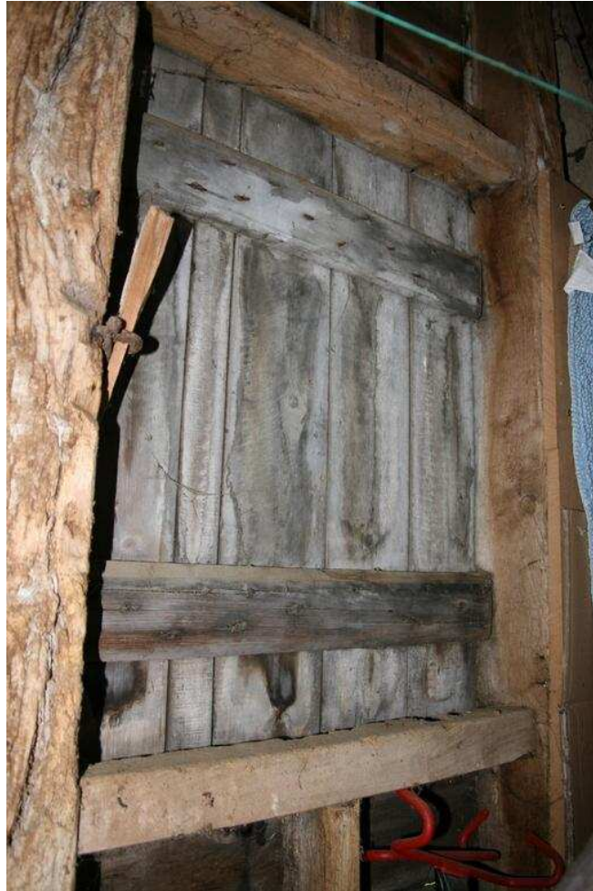
Plate 15 - detail of shutter, NW elevation of midstrey
