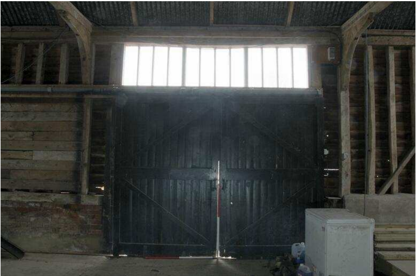
Plate 12 - double doors in SE elevation of Bay 2
