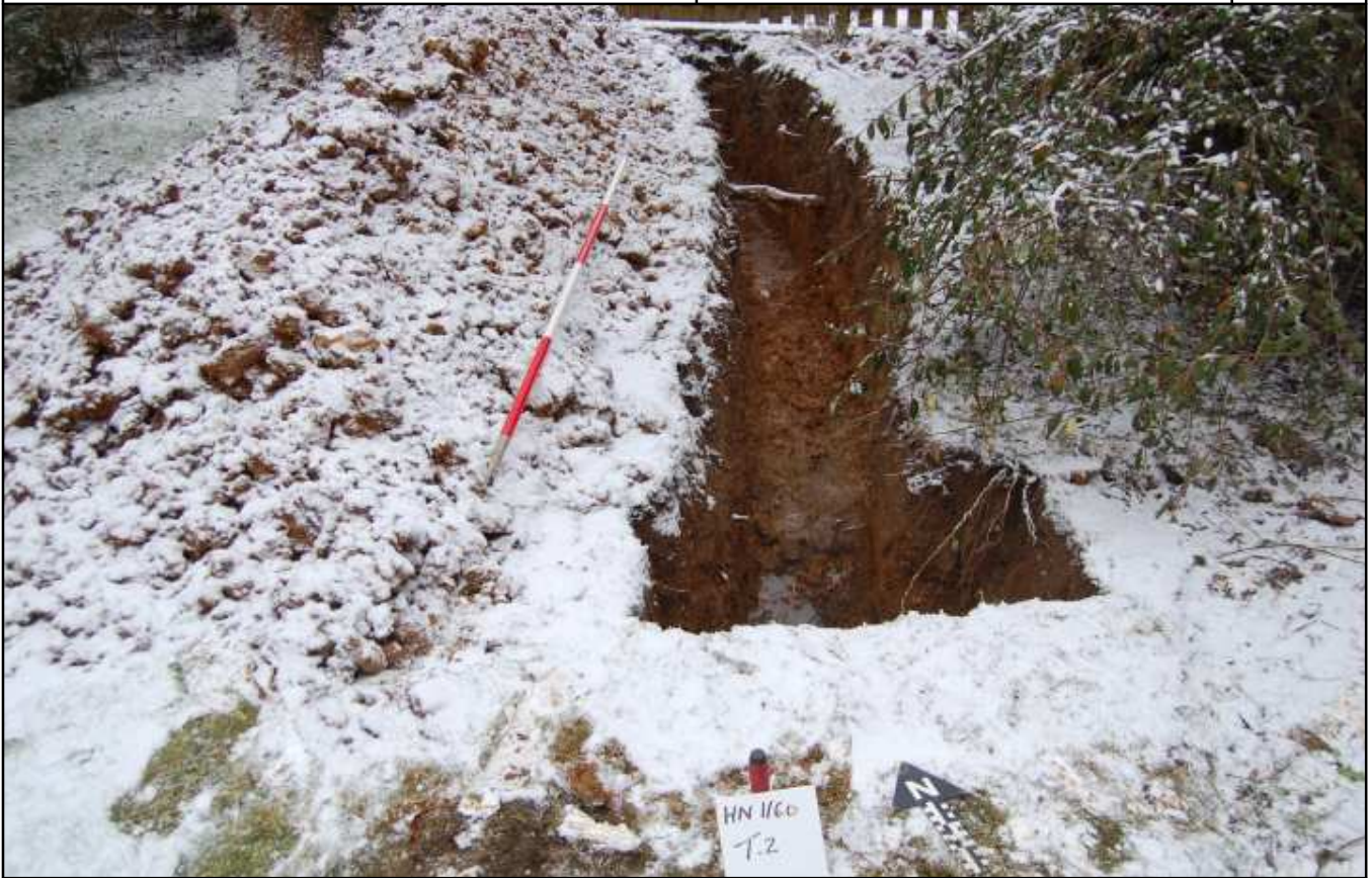
Plate 3: Service trench, looking N
