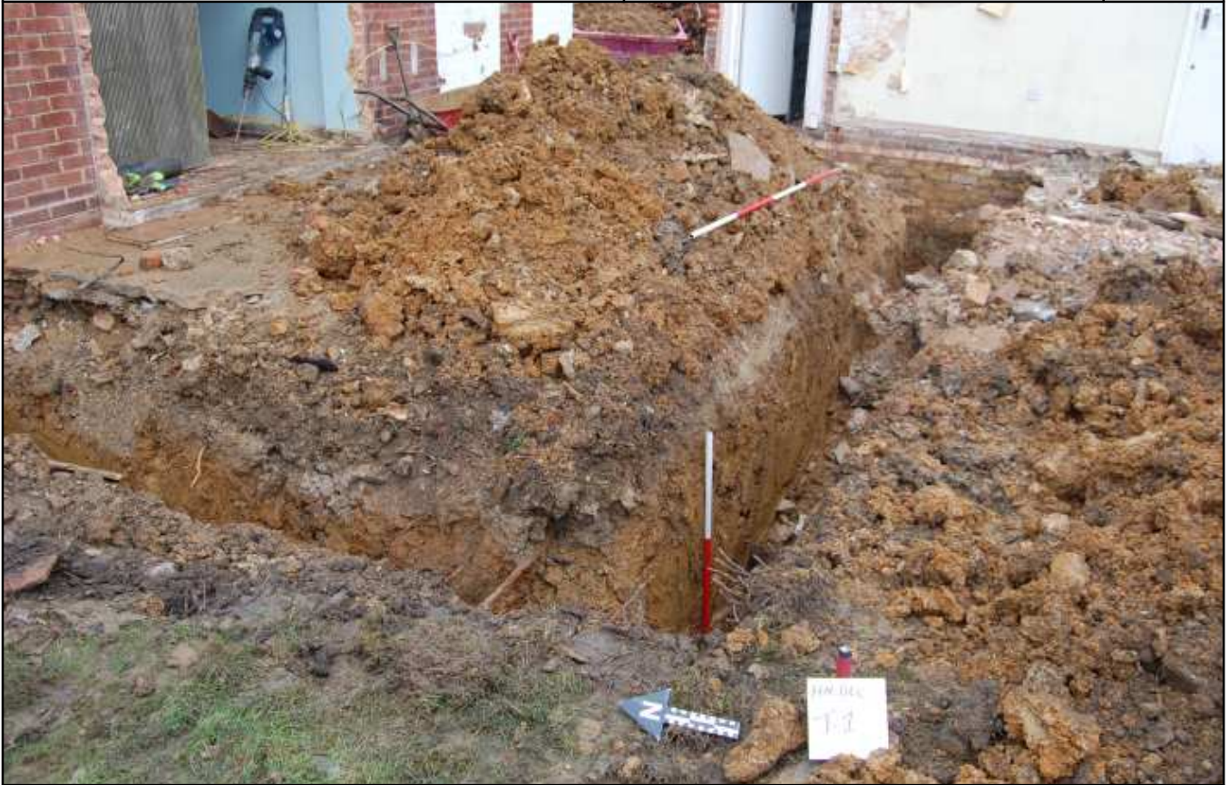
Plate 1: Footings for new extension, looking NE
