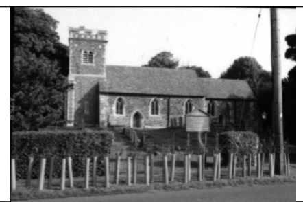
Frame 15: S Elevation of church
