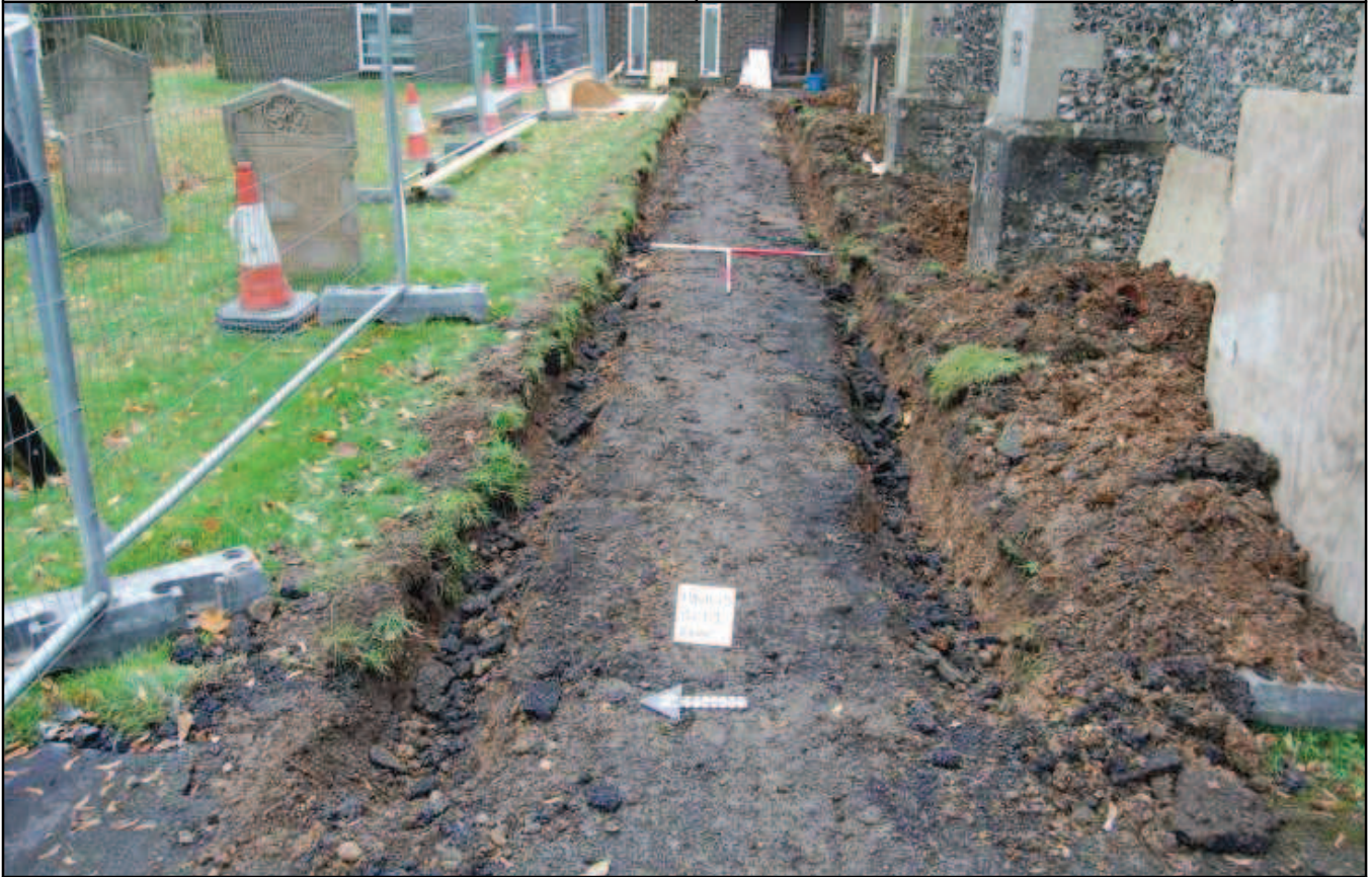
Plate 1: Area of main ground reduction, looking east
