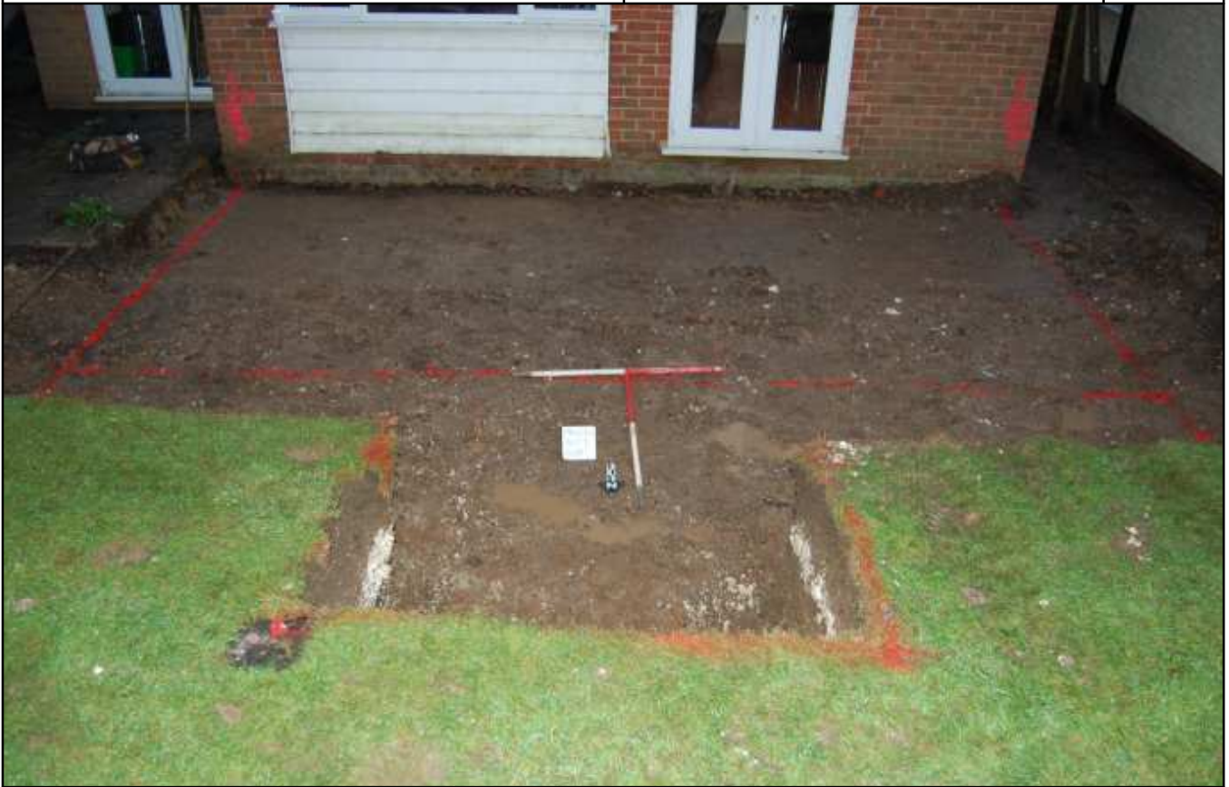
Plate 1: General ground reduction for Plot 1, looking south
