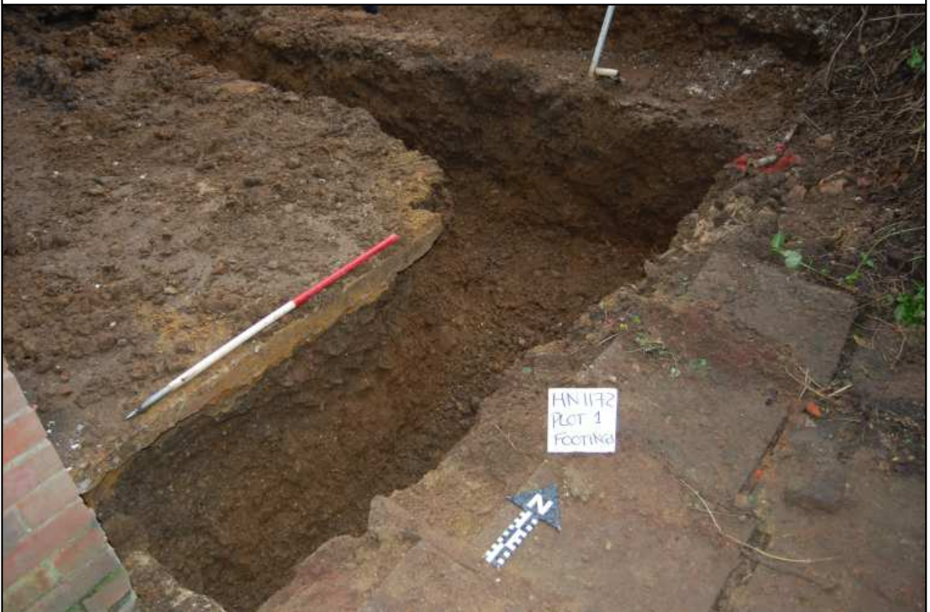
Plate 4: Indicative footing trench within plot 1, looking northwest
