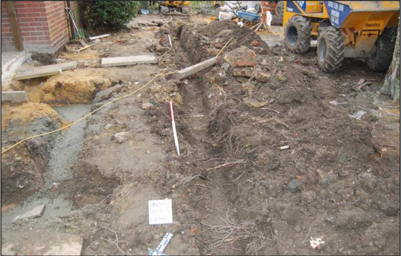
Plate 7: Drainage trench, looking southeast
