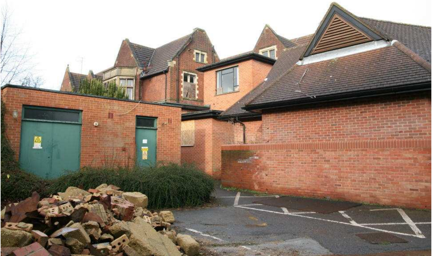
Plate 05 - Extensions to east end of south range, facing north-west
