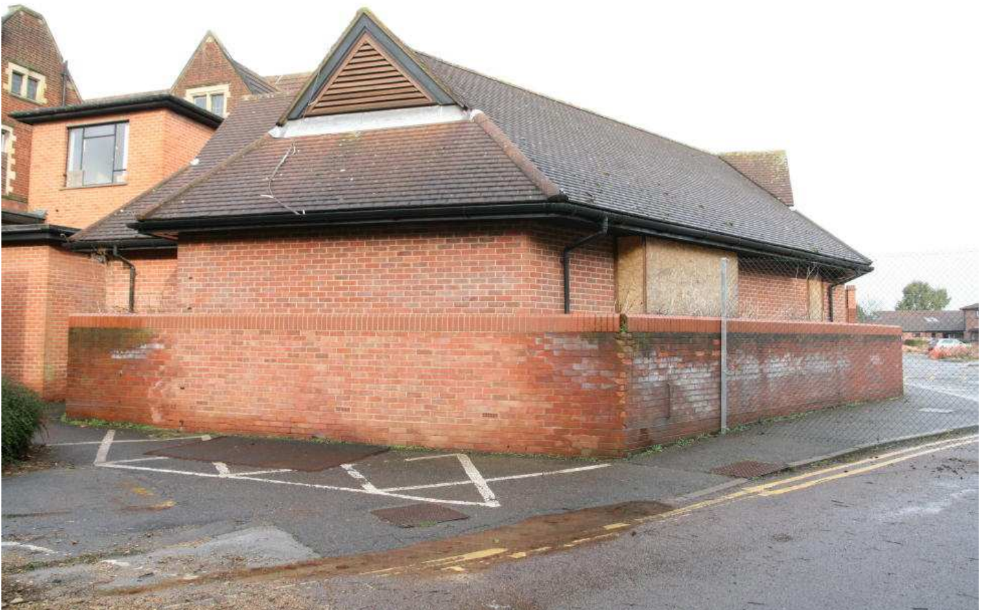
Plate 06 - Eastern extension, facing north-west
