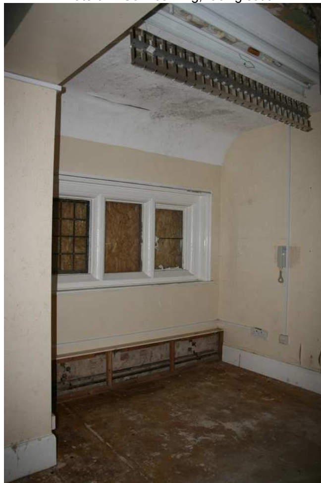
Plate 08 - Service wing, western room, facing north-east
