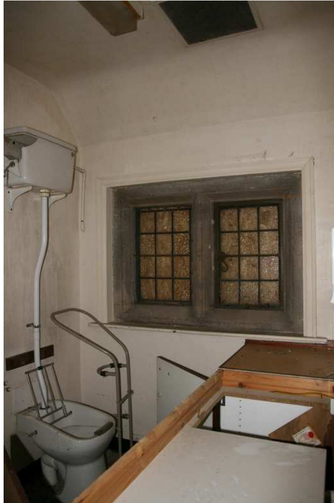
Plate 09 - Service wing, eastern room, facing north
