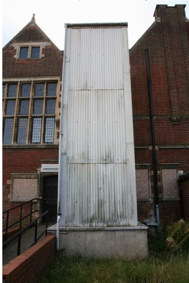
Plate 02 - Lift shaft, facing south
