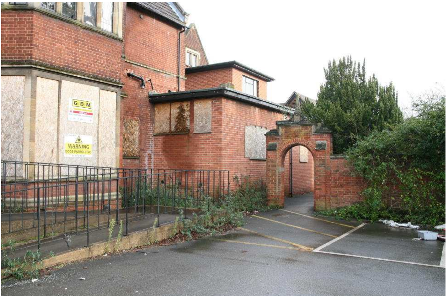
Plate 04 - Extensions to east end of south range, facing north-east
