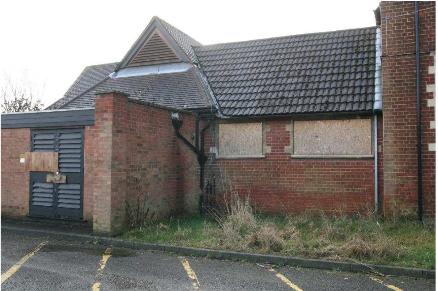
Plate 07 - Service wing, facing south
