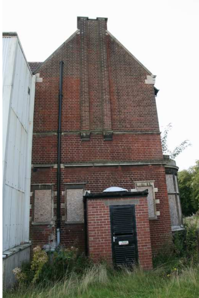
Plate 03 - Lift motor housing, facing south
