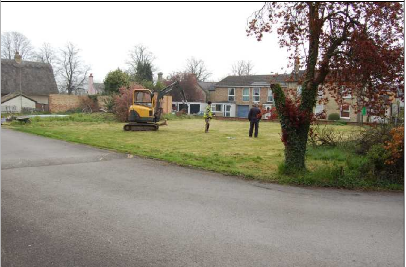
Plate 2: Site prior to excavation, looking east
